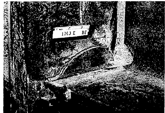
b. Column Flange "Divot" Fracture
