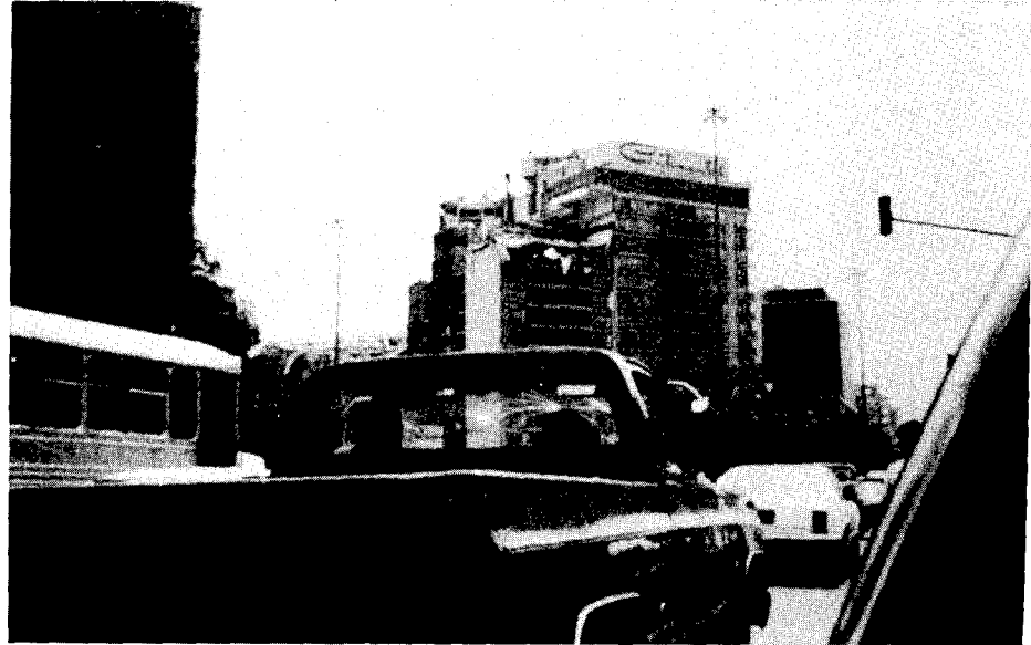
FIGURE 6 Hotel Continental after 1985 Mexico City earthquake (EQE, Inc., San Francisco).
