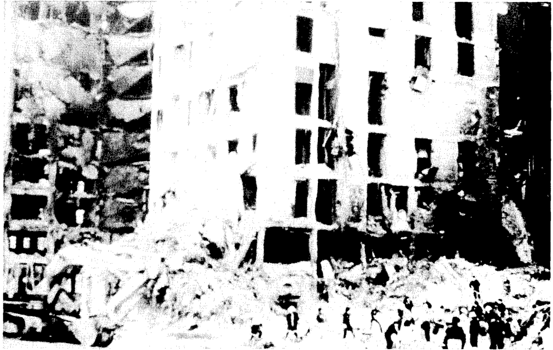
FIGURE 24 Hotel Regis after 1985 Mexico City earthquake and subsequent fire.
