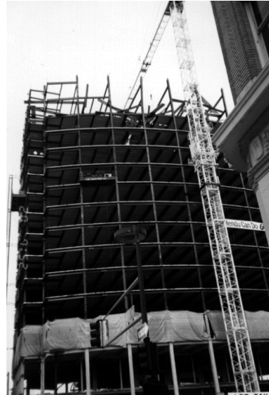
Construction of a modern steel frame building in which the ends of beams are rigidly joined to columns by welded connections.
