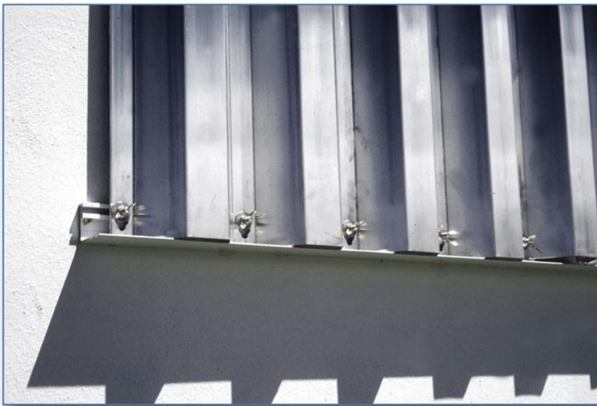
Figure 6-55 View of a metal shutter designed to provide missile protection for windows
