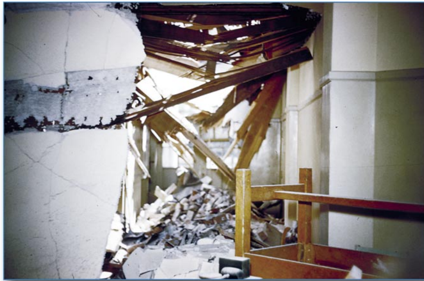
Figure 4-19 Destroyed exit corridor, Bakersfield, Kern County, CA, 1952
