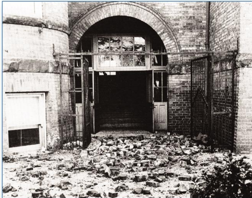
Figure 4-22 Another dangerous entry collapse, Seattle, WA, 1949
