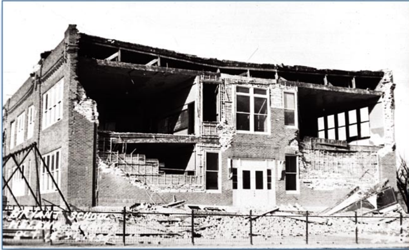
Figure 4-20 Typical school damage, Helena, MT, 1935
