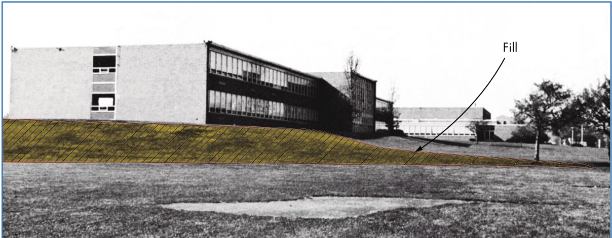
Figure 5-5 High school in Bloomsburg, PA, elevated on fill
