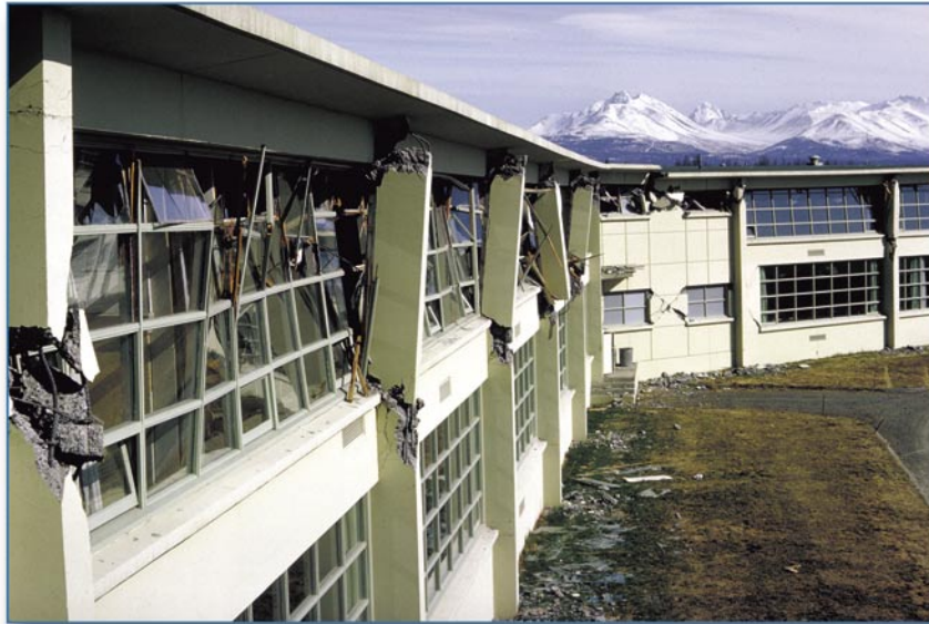
Figure 4-25 Severe structural damage to the West Anchorage High School, Anchorage, AK, 1964
