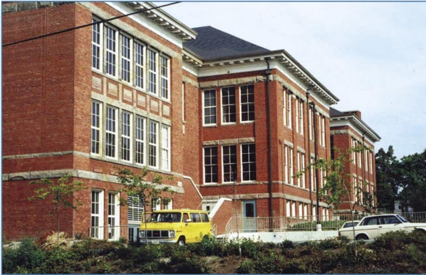
Figure 4-37 Retrofit of B.F. Day Elementary School, Seattle, WA
