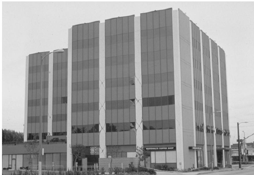
Figure 3-1 Six-story concrete-moment-frame medical building that was severely damaged by the magnitude-6.8 Northridge, California, earthquake of January 17, 1994. The building was subsequently demolished without removing contents. (photo courtesy of the Earthquake Engineering Research Center, University of California at Berkeley)
