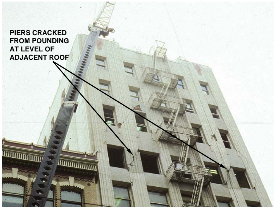
Figure 3-12 Photo showing damage caused by the pounding of a 10-story steel-frame building (with masonry infill walls) against a seven-story building. Most of the cracking damage to the piers of the taller building was at the roof line of the shorter building (Most of the cracking damage to the piers of the taller building was at the roof line of the shorter building. ATC-20 Training Slide Set photo)
