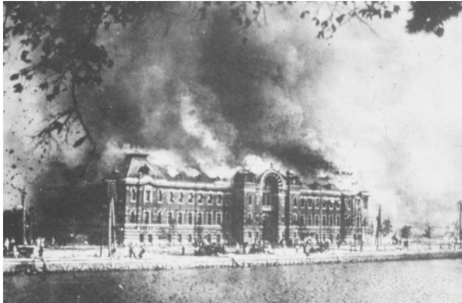
Figure 3-14 Photo showing the burning of the Tokyo Police Station following the magnitude-8.3 Tokyo/Kanto earthquake of 1923.
