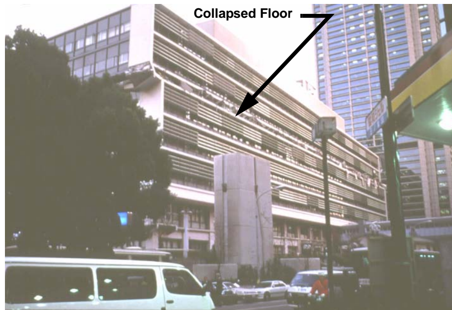
Figure 3-2 Eight-story reinforced-concrete-frame office building in Kobe, Japan that partially collapsed during the magnitude-7.8 earthquake of January 17, 1995. Note that the sixth floor is missing, due to collapsed columns at that level. Seismic codes in Japan are essentially equivalent to those in the United States. (photo courtesy of C. Rojahn)
