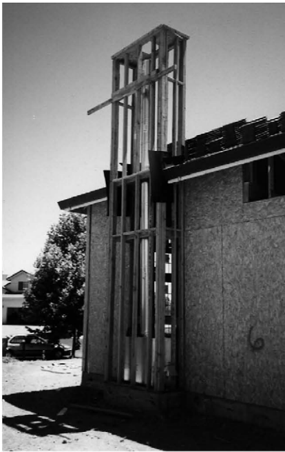
Figure 7-7 Factory-built flue and light-frame enclosure.
