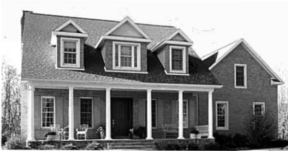
Figure 5-14 House constructed with masonry walls.
