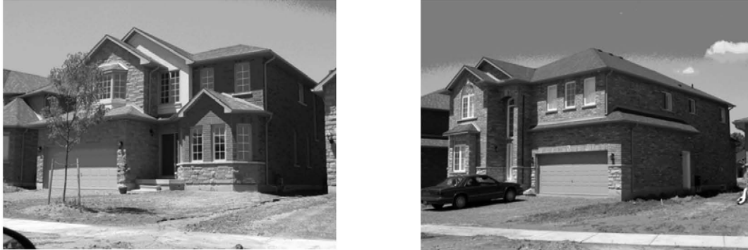
Figure 5-11 Applications of masonry and stone veneer.
