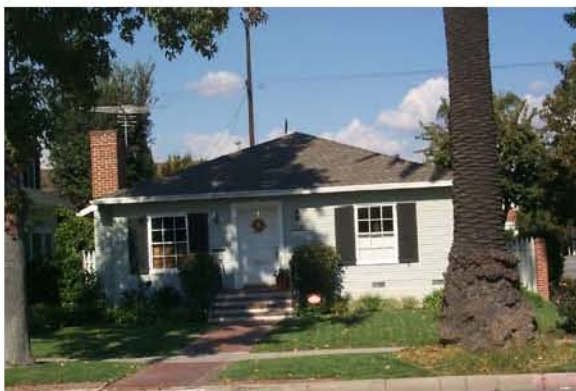
Figure E-1 Single family residence (an example of the W1 identifier, light wood-frame residential and commercial buildings less than 5000 square feet).
