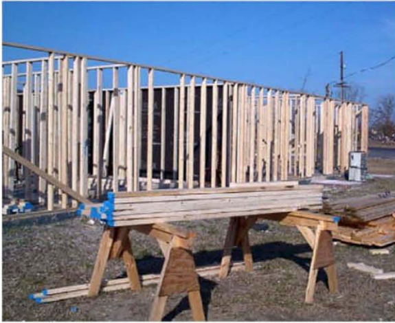
Figure E-4 Stud wall, wood-framed house.
