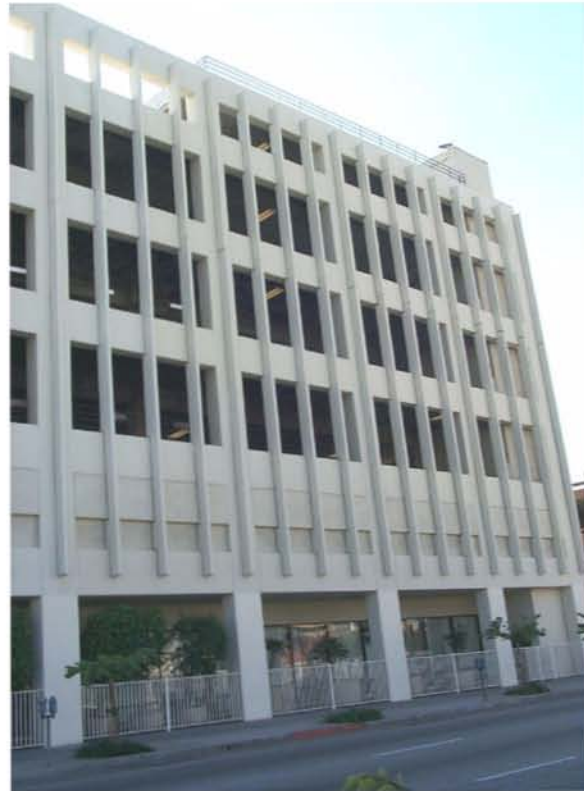
Figure E-28 Concrete moment-resisting frame building (C1) with exposed concrete, deep beams, wide columns (and with architectural window framing).
