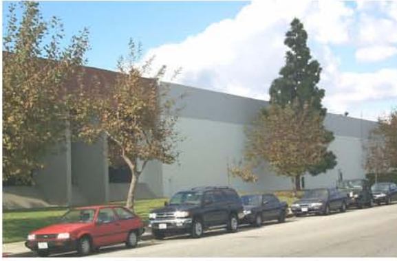
Figure E-36 Tilt-up industrial building, 1970s.
