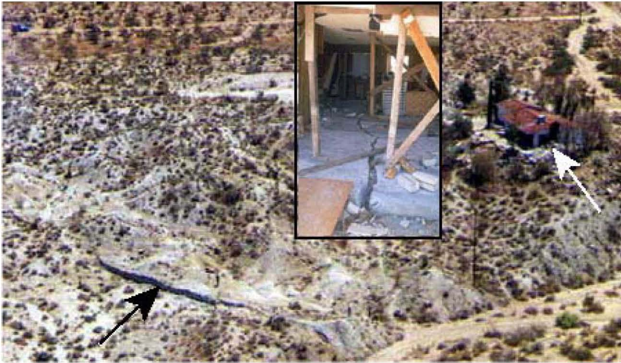
Figure F-6 Near-field effects, 1992 Landers earthquake, showing house (white arrow) close to surface faulting (black arrow); the insert shows a house interior.
