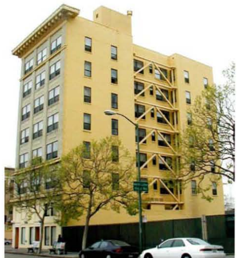
e. Pre-1933 URM (rehabilitated)
