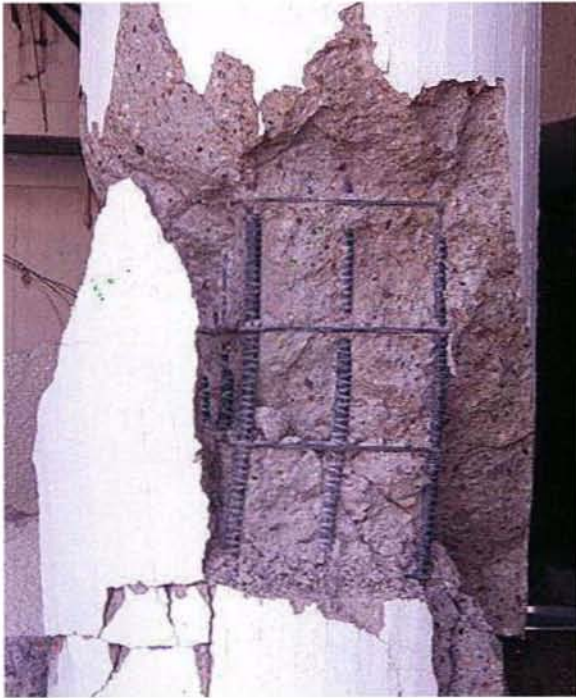
Figure E-27 Example of ductile reinforced concrete column, 1994 Northridge earthquake; horizontal ties would need to be closer for greater demands.
