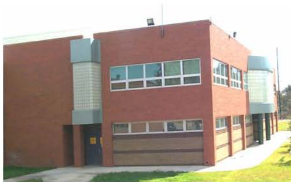
Figure E-46 Modern reinforced brick masonry.
