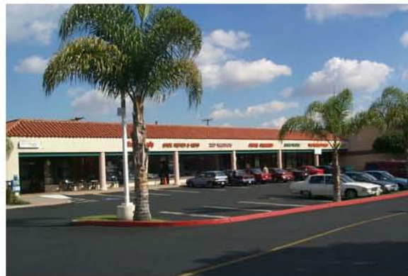
Figure E-2 Larger wood-framed structure, typically with room-width spans (W2, light, wood-frame buildings greater than 5000 square feet).
