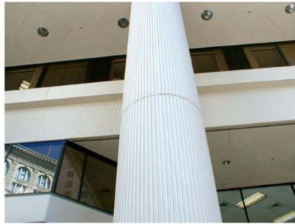
Figure D-3 Detail of the column facade of Figure D-2.
