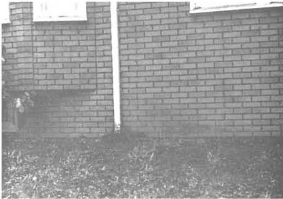
Figure D-16 Asphalt siding with brick pattern.
