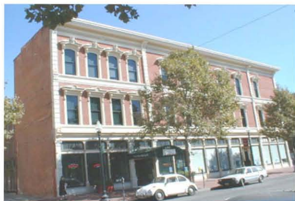
Figure E-51 West coast URM bearing-wall building.
