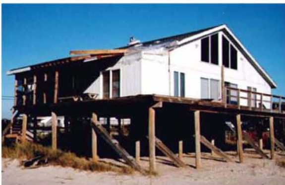
Figure E-6 Timber pole framed house.
