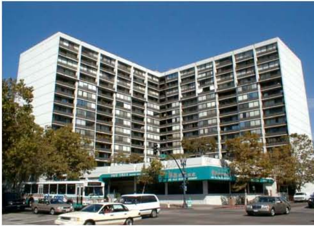
Figure 3-18 Example of a building, with a plan irregularity, with two wings meeting at right angles.
