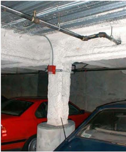
Figure 3-11 Interior view showing fire-proofed columns and beams, which indicate a steel building (S1, S2, or S4).
