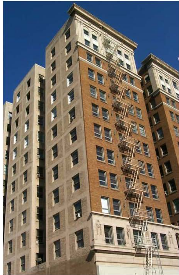
Figure 5-9 Exterior view of 3711 Roxbury.
