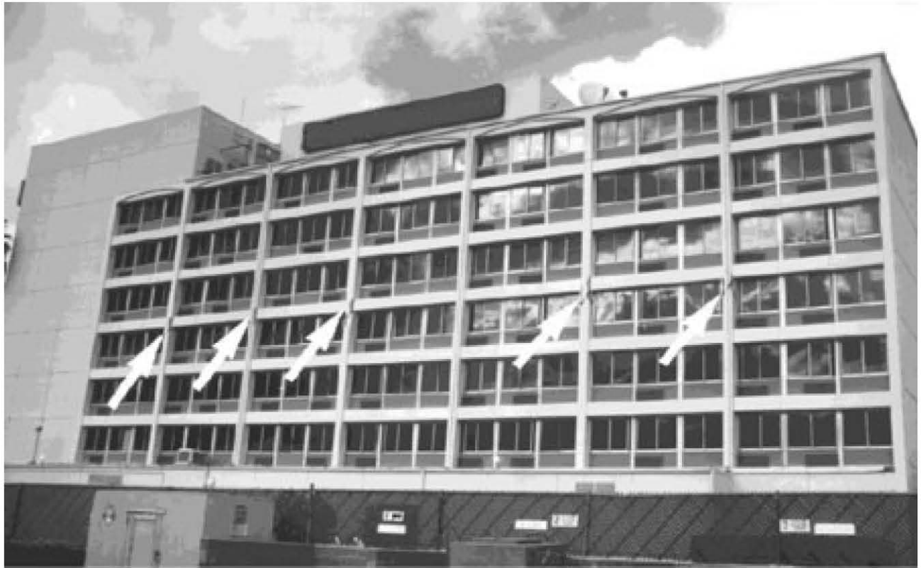
Figure E-29 Locations of failures at beam-to-column joints in nonductile frames, 1994 Northridge earthquake.
