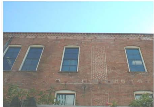
Figure E-55 Upper: Two existing anchors above three new wall anchors at floor line using decorative washer plates. Lower: Rehabilitation techniques include closely spaced anchors at floor and roof levels.
