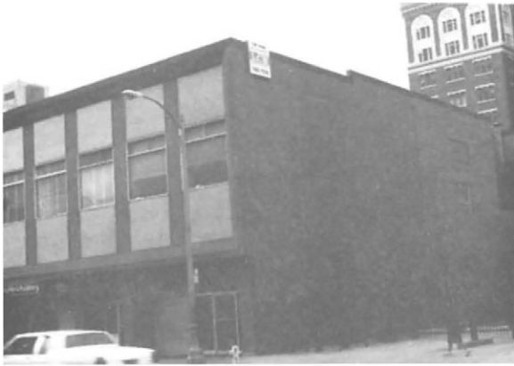
Figure D-9 A concrete shear-wall structure with a 1960s renovated facade.
