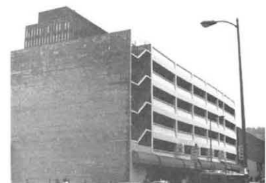
g. 1950 – 1965 parking structure
