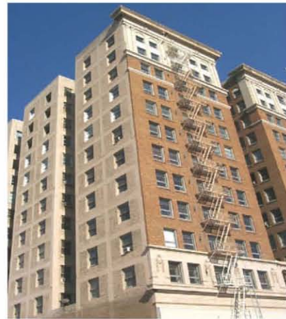
Figure E-33 Concrete frame with URM infill.
