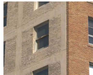
Figure E-34 Blow-up (lower photo) of distant view of C3 building (upper photo) showing concrete frame with URM infill (left wall), and face brick (right wall).
