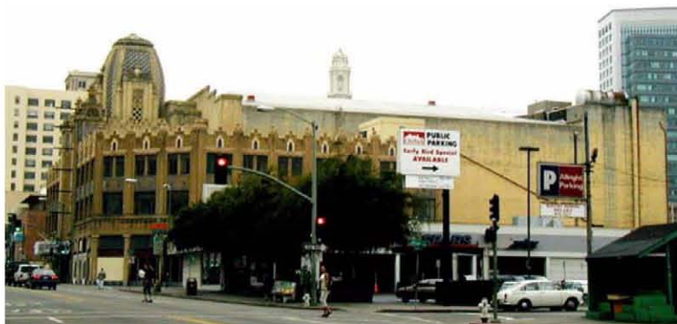
h. 1920-1930; theater and shops complex, reinforced concrete
