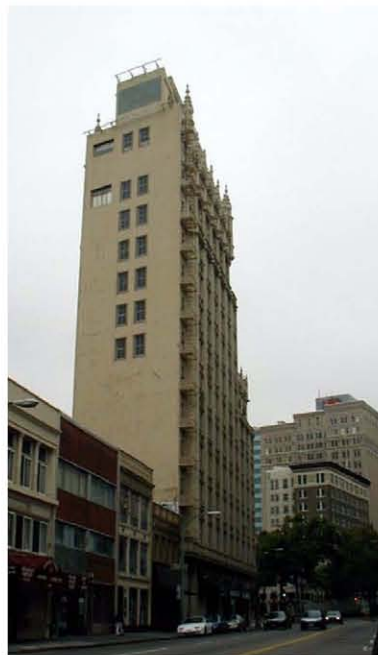
e. 1920-1930; windows create coupled shear walls.
