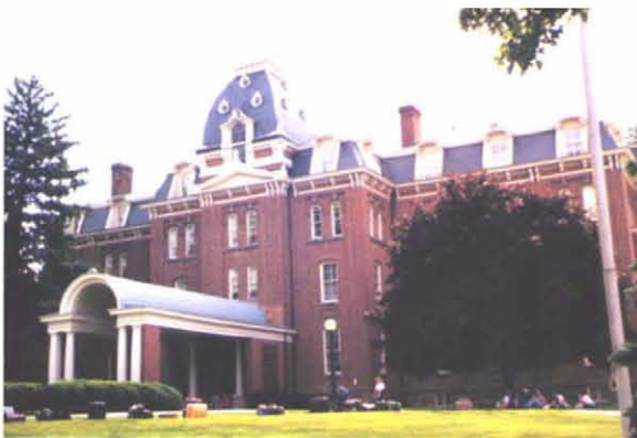
Figure E-50 East coast URM bearing-wall building.
