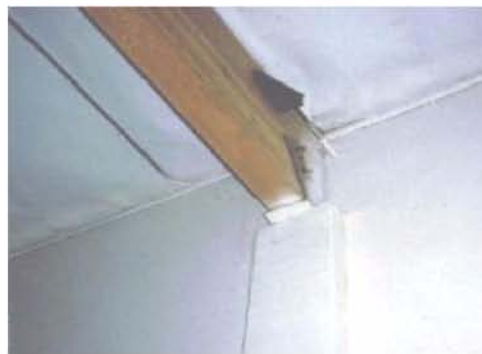
Figure E-40 Newly installed anchorage of roof beam to wall in tilt-up building.
