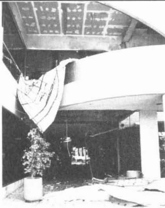
Failure of suspended ceiling and light fixtures in furniture store Earthquake Damage: 1994, Northridge, California Photo Credit: William McKeivitt
