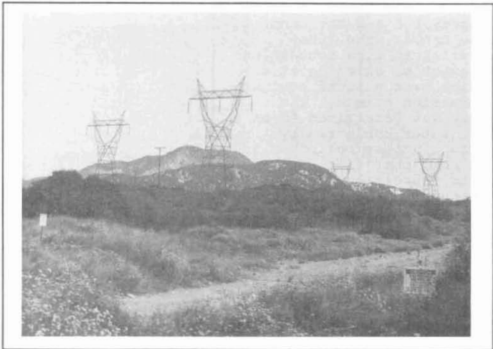
Figure 18 Power Lines, Natural Gas & Petroleum Products Pipelines Intersection Over the San Andreas Fault Rift Zone
