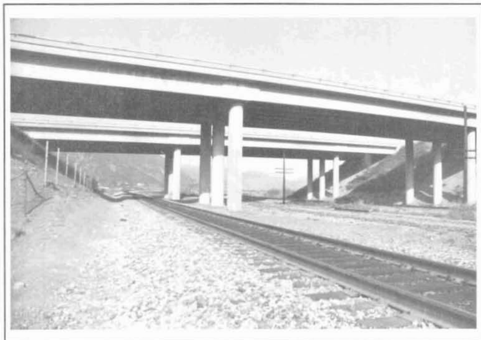
Figure 25 I-15 Bridge Over The Railroads In Cajon Wash
