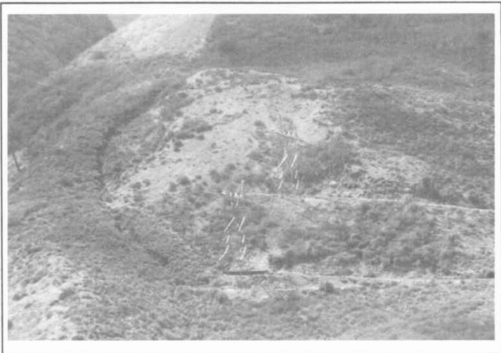
Figure 17 A Landslide Scar With Power Towers In The Slide Area
