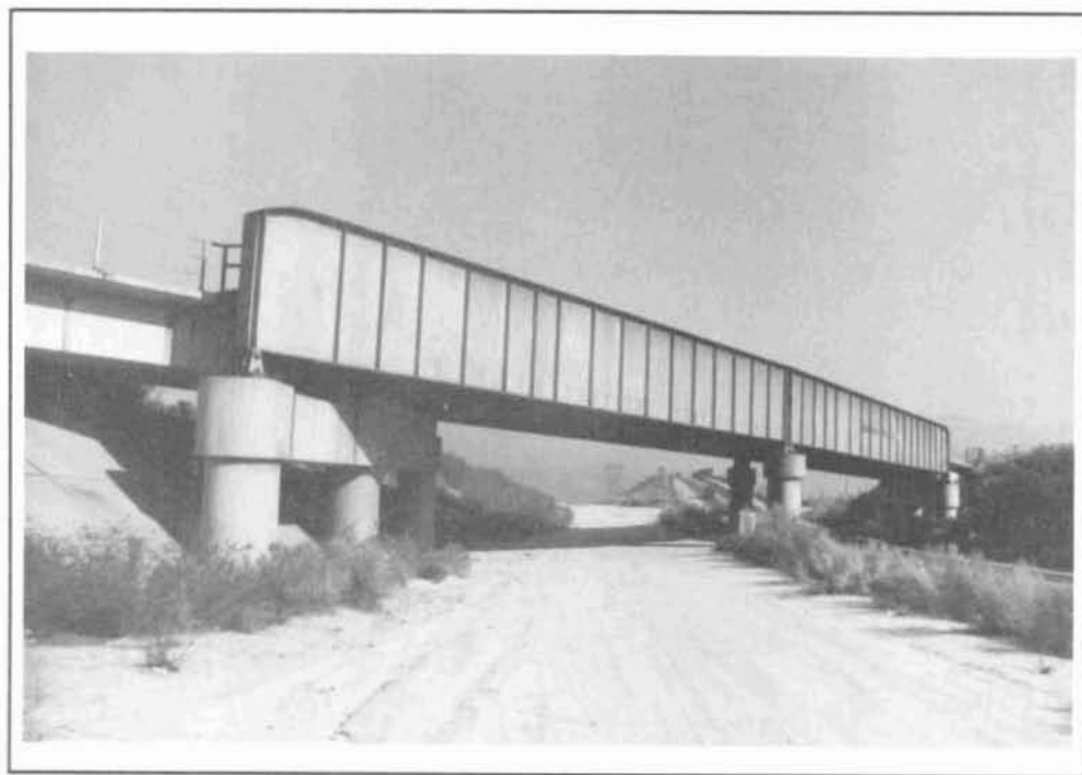
Figure 29 Railroad Bridge Over Highway 138 (Collapse Expected)
