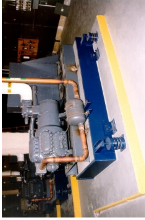
Figure 121: Typical installation of an open spring arrangement with snubbers.
