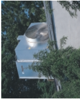
Figure 36: Fluid cooler cross flow with self-contained sump.
