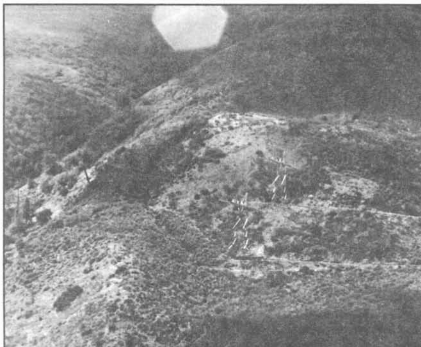
Figure 8 Electrical Towers on a Landslide Scar (Directly Above a Fuel Pipeline & a Railroad)
