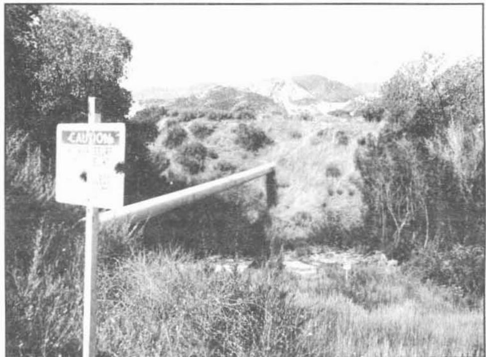
Figure 9 Two Natural Gas Pipelines, One Exposed One Buried, Next to Highway 138
