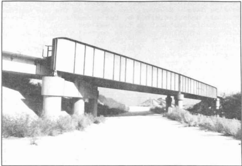
Figure 10 A Railroad Bridge Estimated to Collapse Onto Highway 138 (Highway 138 is located under the right span)
