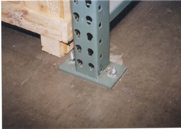
Figure 1-5 Typical column base plate connection.
