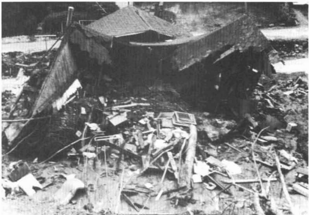
Figure 7. The remains of a house where three children died in a mudflow in Kanawha City, West Virginia. The movement was triggered by heavy rainfall from a cloud-burst on July 9, 1973 (Lessing et al., 1976).
