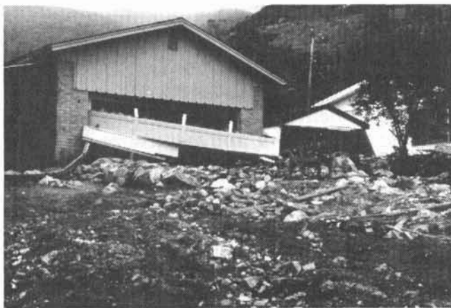
Figure 2. Major damage to homes in Farmington, Utah as a result of 1983 Rudd Creek mudslide (photograph by Robert Kistner, Kistner and Associates).
