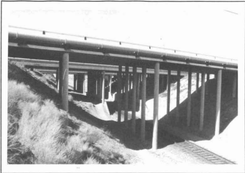
Figure 3.5-7 I-15 and Access Road Bridges Over the Railroad
