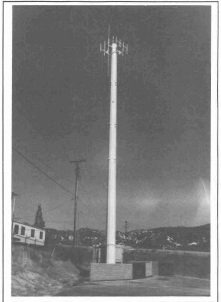
Figure 3.2-9 Cajon Junction Cellular Phone Antenna
