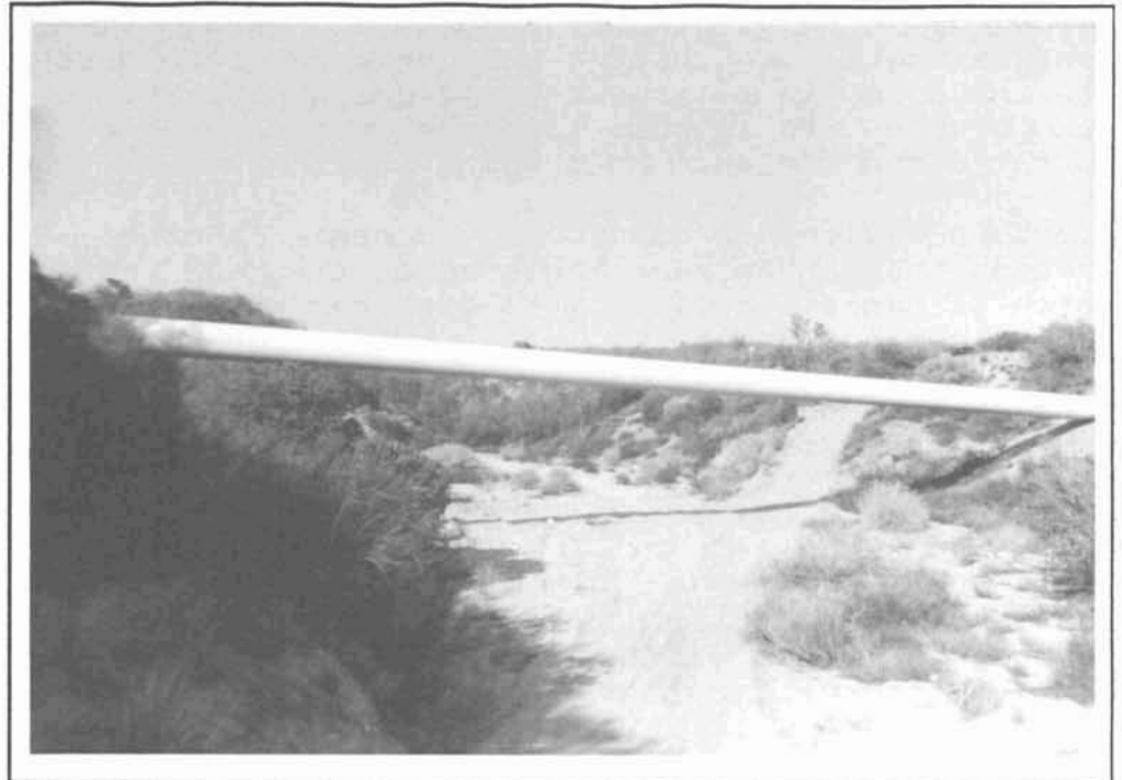
Figure 3.4-3 An Exposed Section Of The Natural Gas Pipeline
