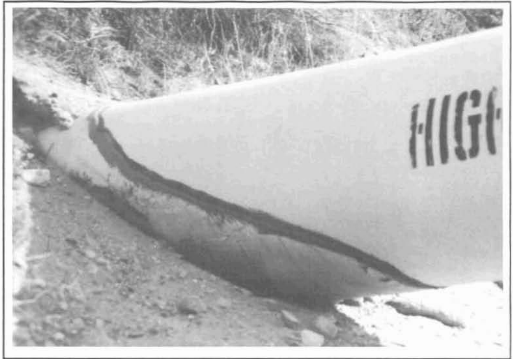
Figure 3.4-4 Details of the Ground Support For Exposed Sections Of Natural Gas Pipelines
