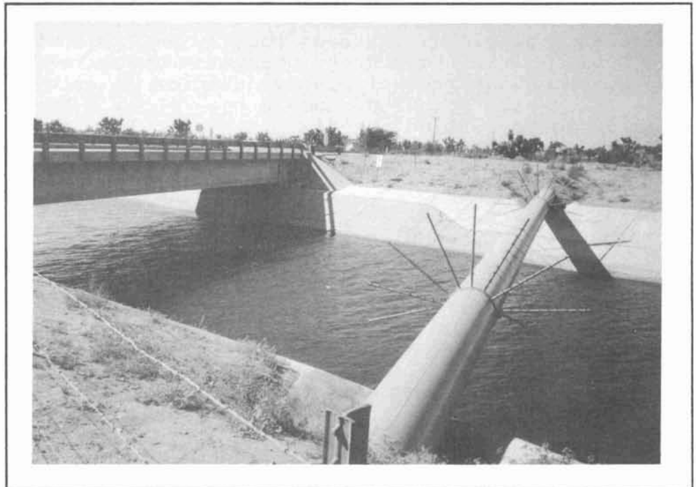
Figure 3.4-6 The Natural Gas Pipeline Crossing the California Aqueduct
