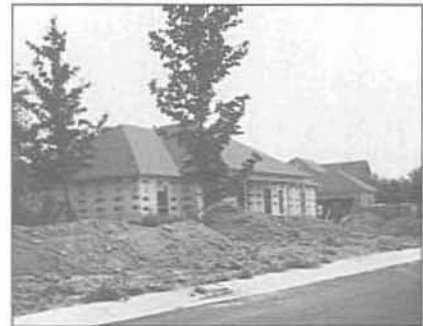
FIGURE 5.1 New construction continues to flourish in Jonesboro. (Source: City of Jonesboro)
