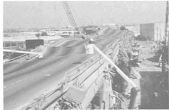
MMI IX: General panic; ground-cracking; considerable damage in buildings designed to seismic code. (Photo: J. David Rogers)
