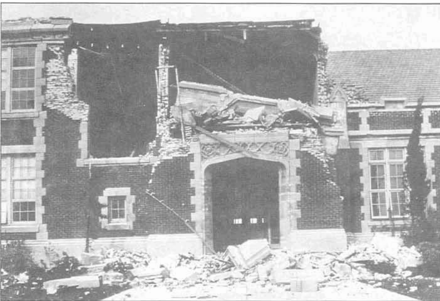
FIGURE B.2 This school building sustained severe damage in the 1933 Long Beach, California, quake. (Photo: U.S. Dept. of Commerce, NOAA)
