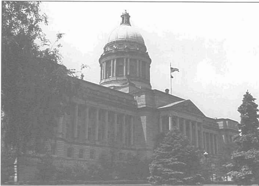
FIGURE 4.2 Kentucky has a statewide building code requirement (state capitol shown above). (Source: Kentucky Legislative Research Commission)
