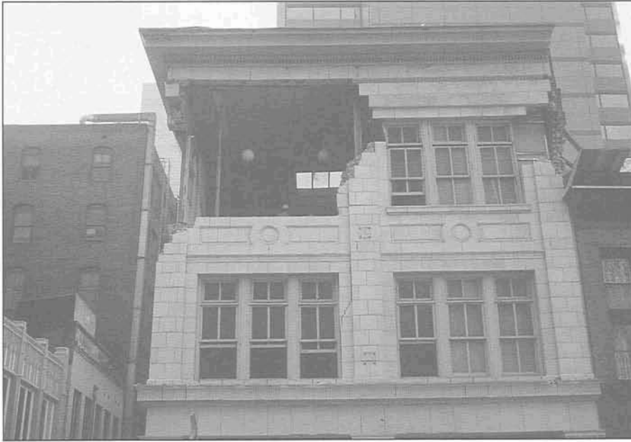
FIGURE 3.1 Most of the building damage in the 1989 Loma Prieta earthquake was to older unreinforced masonry buildings built before the adoption of seismic codes. (Photo: Rob Olshansky)
