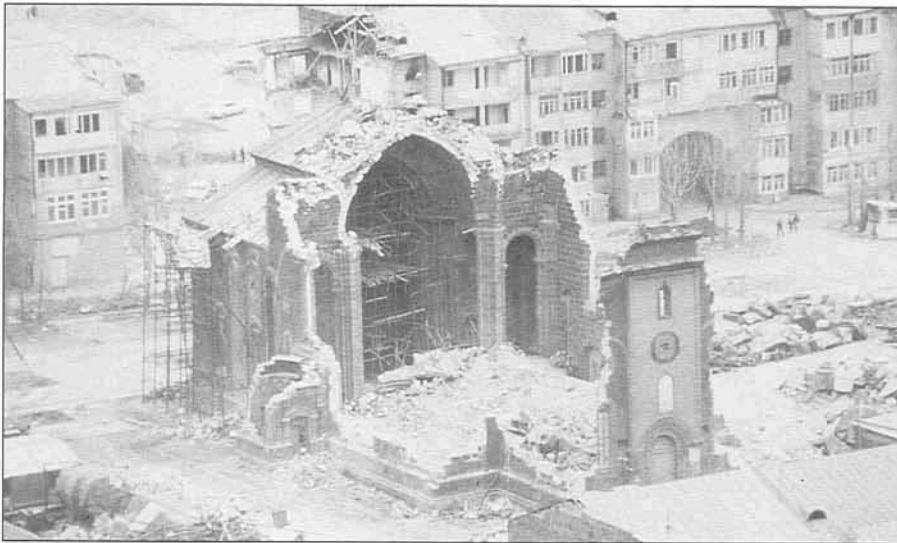
FIGURE 3.6 The extensive damage in Armenia in 1988 can be attributed to the lack of seismic-resistant design and construction. The same limitations are true of existing building stock throughout the United States. (Photo: NOAA)
