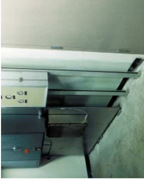
Figure 155: Two different ways to support control panels: using a metal plate attached to floor and ceiling with steel angles (left); using struts extending to floor and ceiling (right).
