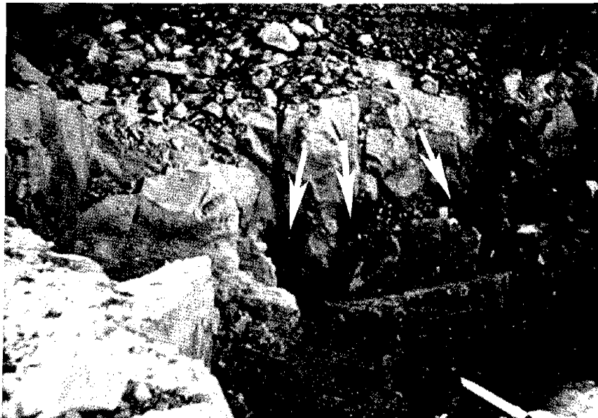
FIGURE 5-1 Caverns in dolomite foundation of a gravity concrete dam. (Later filled with concrete to ensure adequate bearing for the dam.)
