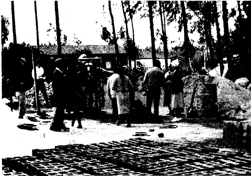
FIGURE 7.5 Minga (traditional community work group) making mud bricks using a brick-compacting machine that had been donated to the community, Tabacundo, Pichincha Province.
