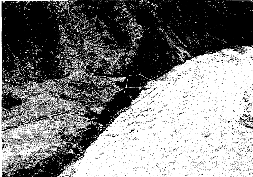
FIGURE 1.9 Destruction of Trans-Ecuadorian oil pipeline and highway by flood erosion on the left bank of the Coca River as a result of the March 5, 1987, earthquakes.
