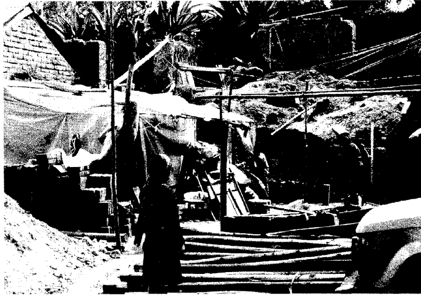
FIGURE 7.4 Temporary dwelling of plastic sheeting used as a residence while family builds a new home using a metal frame, Tabacundo, Pichincha Province.
