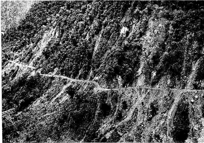
FIGURE 5.5 Landslides along the Trans-Ecuadorian highway 3 km W of its crossing of the Salado River. These rock falls, slides, and avalanches, which were triggered by the March 5, 1987, earthquakes, had blocked the highway almost continuously in the stretch shown in this photograph. The highway was passable at the time of this April 25, 1987, photograph because of the efforts of Corps of Engineers (Ecuadorian Army) highway maintenance crews.
