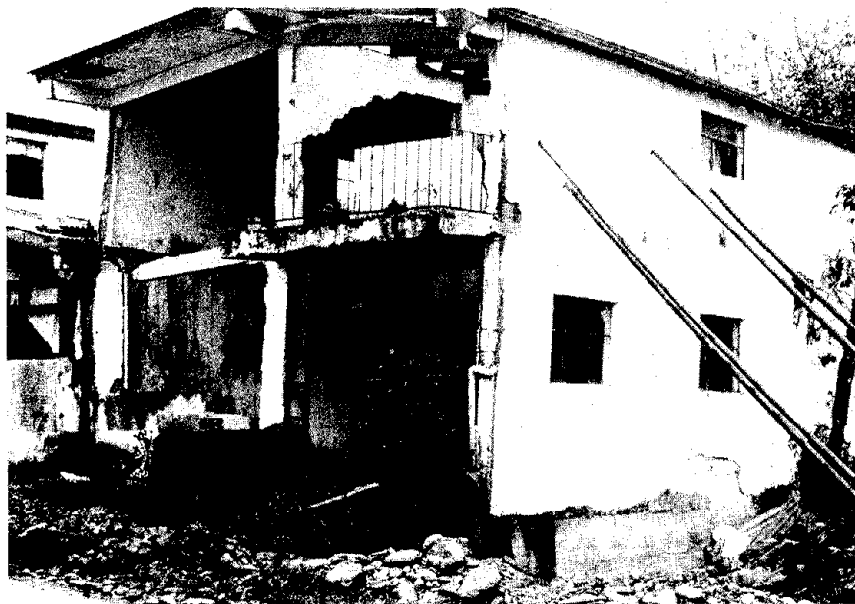
FIGURE 7.2 Damaged concrete-block dwelling in Baeza, Napo Province.
