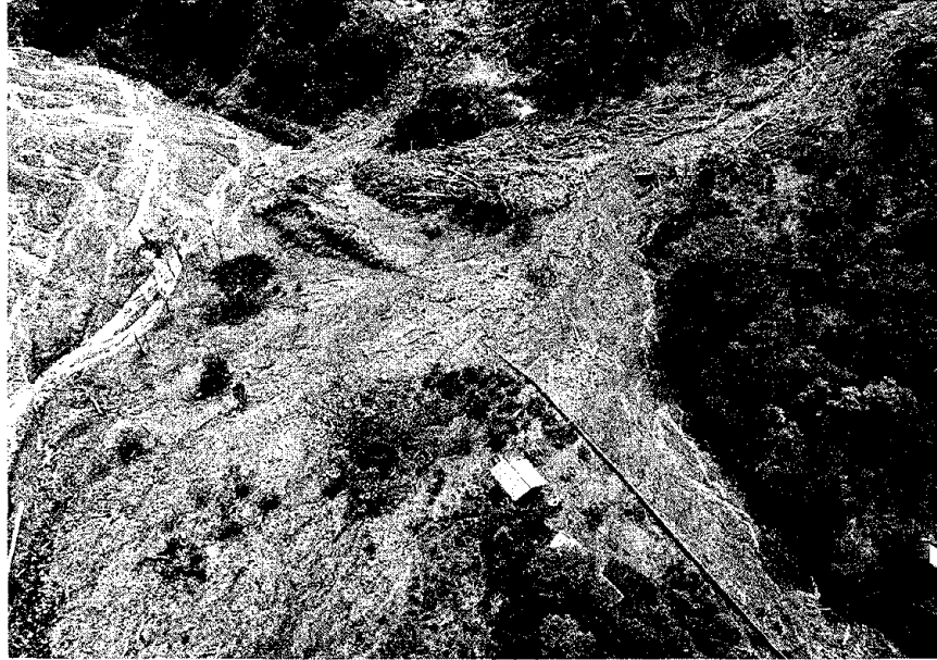
FIGURE 1.8 Aerial view of destruction of the Trans-Ecuadorian oil pipeline and adjacent highway by a debris flow issuing from a minor tributary of the Coca River. Location is near mouth of the Reventador River.
