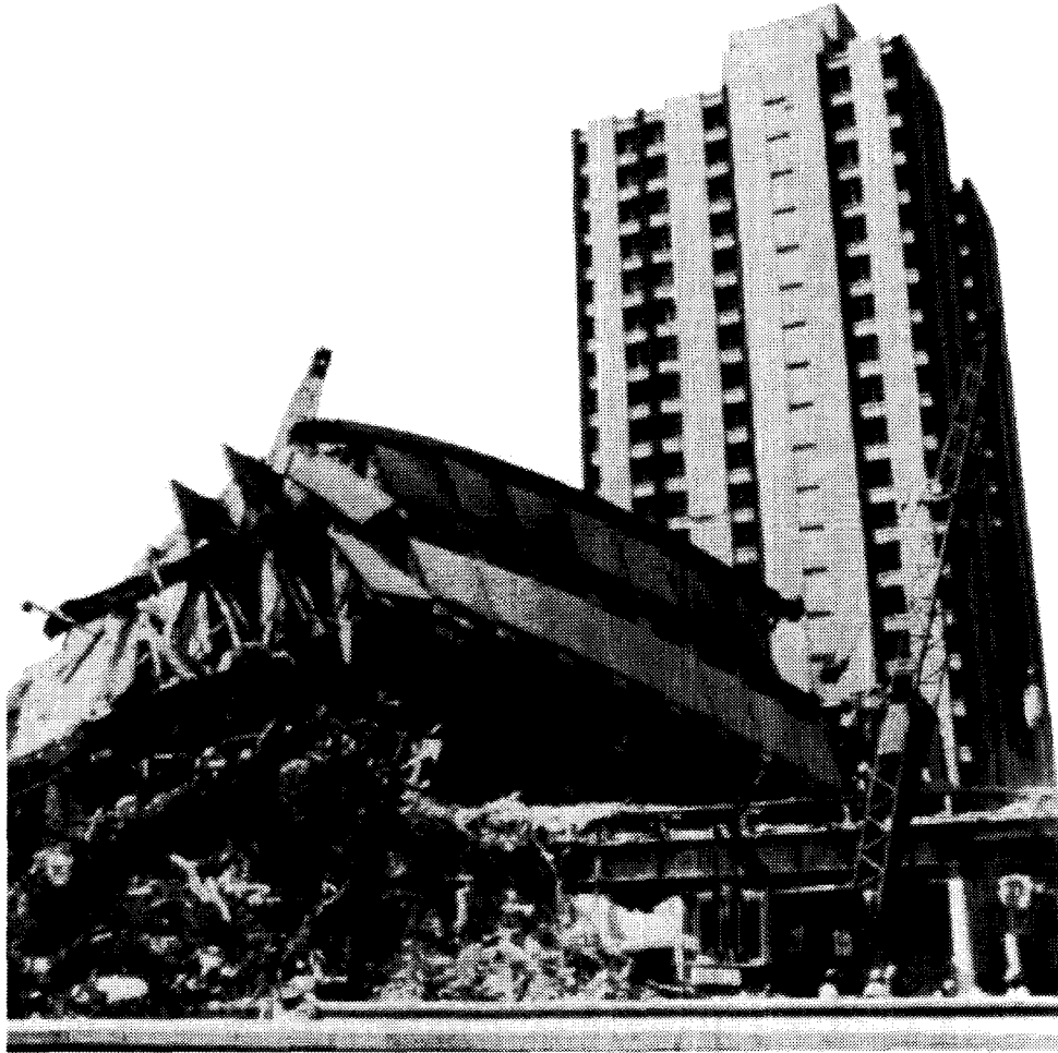
Figure 5. A 21-story steel frame building that has collapsed onto an adjacent 14-story building in Mexico City, 1985.
