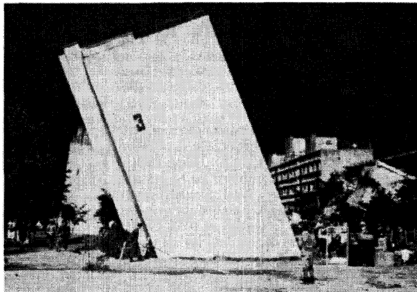
Figure 3b. Close-up view of one of the apartment buildings affected by liquefaction during the Niigata earthquake. Photograph: Courtesy of G. W. Housner.
