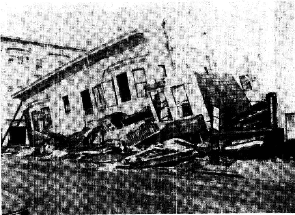
Figure 2a. Four-story building which suffered total collapse of its lower stories (location #3).
