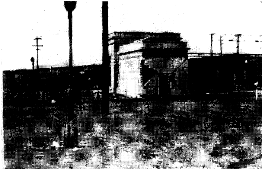
Figure 13. Substation control house damage.
