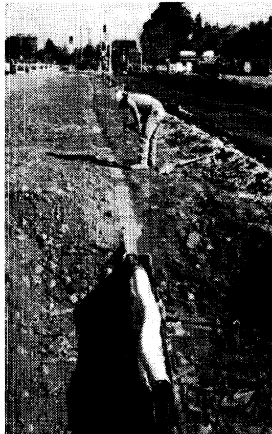
Photo 10. Burying fibre optic cable in process.
