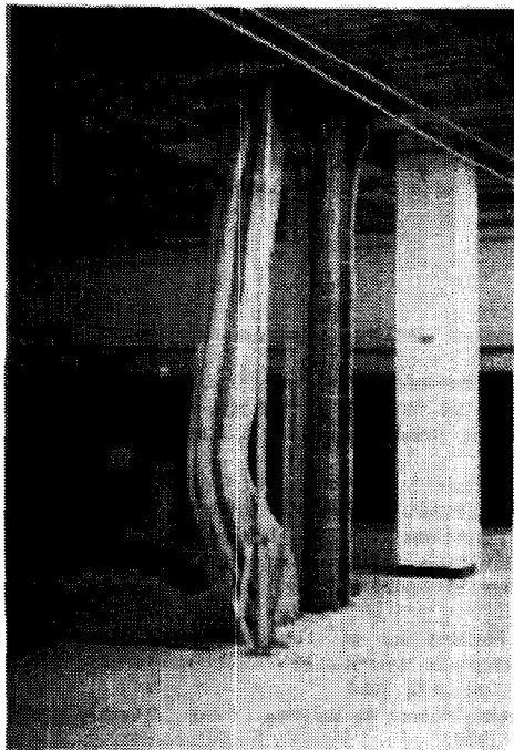
Figure 11a. Oakland CO friction clip failure.
