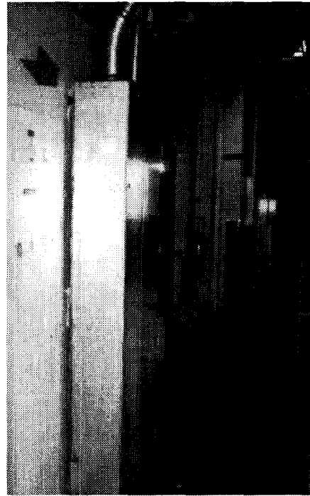
Photo 5. Loma Prieta earthquake 1989. An AC panel in a central office pulled away from the wall. Close up view on the left.
