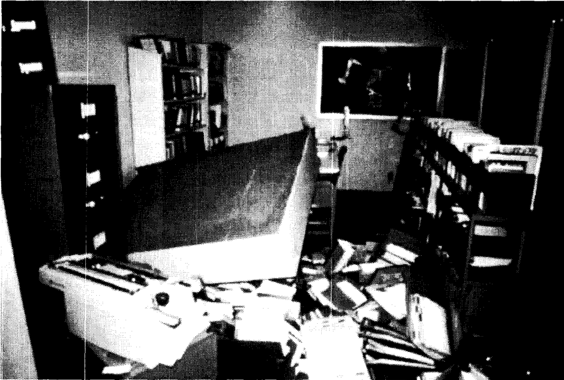
Figure 9. Example of earthquake non-structural damage.
