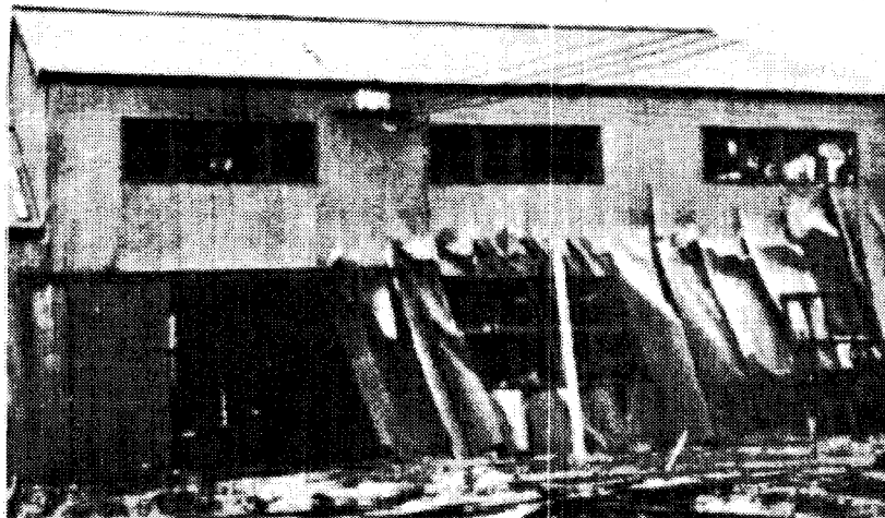
Figure 4b. Building pulled apart by lateral spreading during the 1964 Niigata earthquake. Source: Kawasumi (1968).
