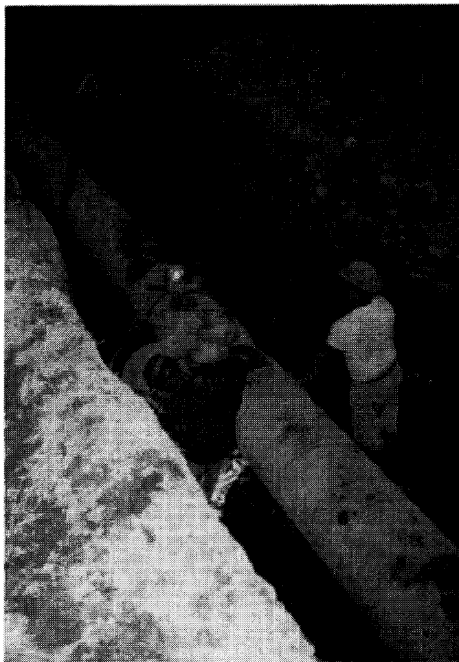
Figure 1. Typical pipeline earthquake failure repair.
