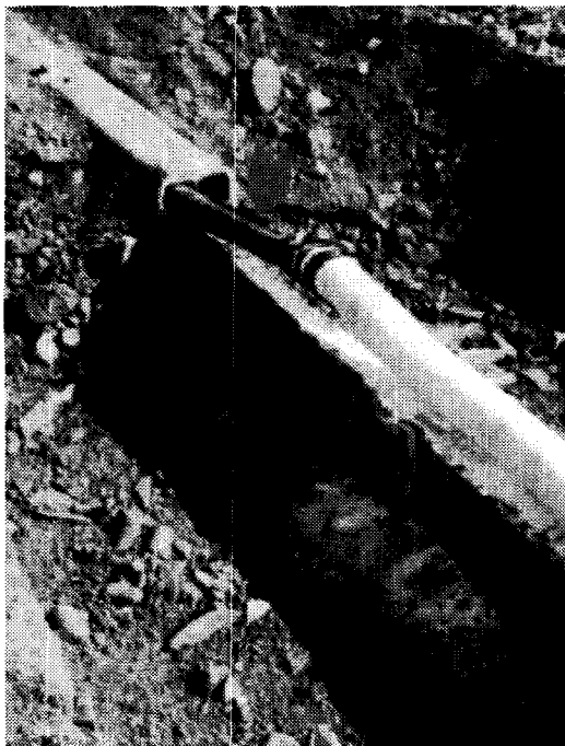
Photo 10. Burying fibre optic cable in process.
