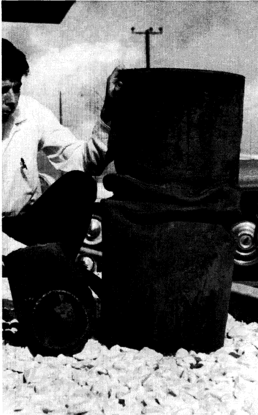
Figure 10. Buckled steel gas pipeline, 1971 San Fernando Earthquake (Photo courtesy Southern California Gas Company).
