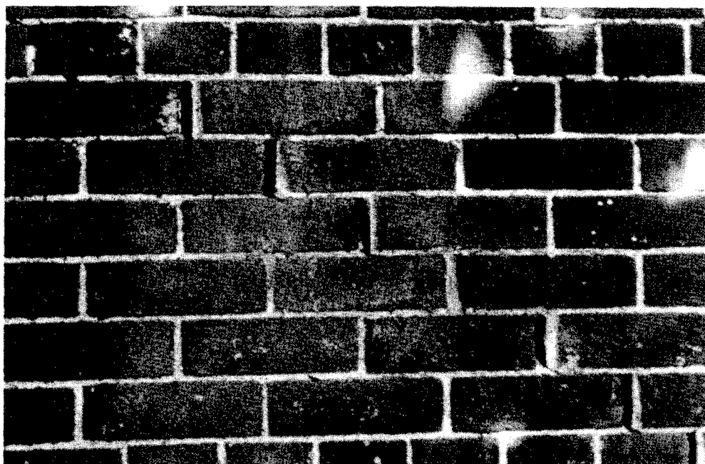
Figure 7-10 Photo of Bed Joint Sliding
