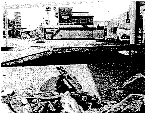
Photo. 3 Up-lift of Underground Gas Storage Tank
