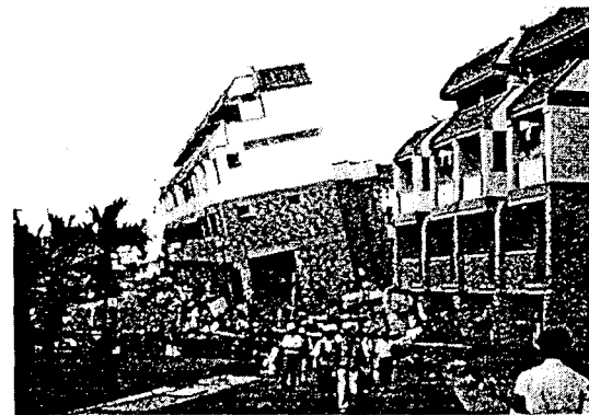
Photo 6 Building just above fault (Shihkang, Taichung County)
