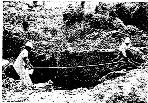
Photo 4 Offset of a Drainage Pipe of 3.6 m (Point I, refer to Fig. 3)
