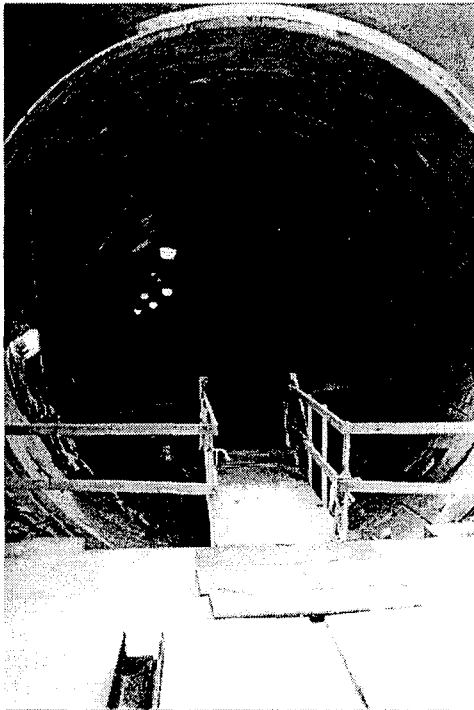
Figure 8: Tunnel under construction in Río Piedras. Precast concrete liner segments are visible.
