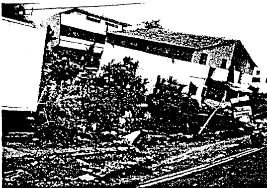
Photo 5 Building just above fault (Fengyuan City, Taichung County)
