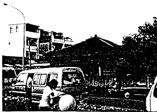
Photo 20 Damage of the wooden building (Tungshih City, Taichung County) The wooden building of tiled roof is observed. Though the building of the photo remained for an inclination, it was also seen the result to collapse in the vicinity.
