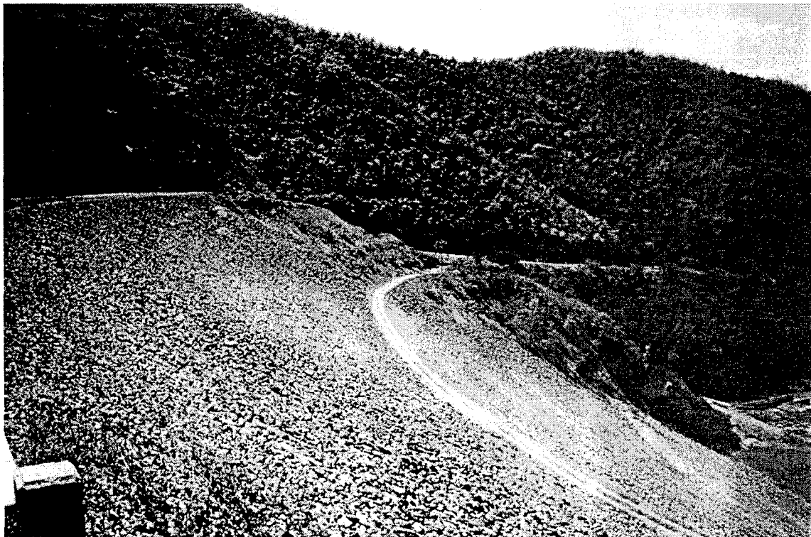
Figure 3: View of Cerrillos Dam embankment.
