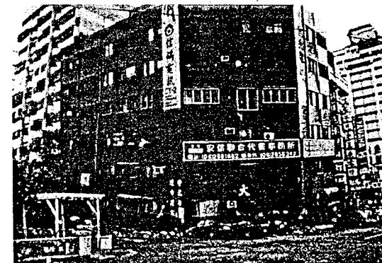
Photo 12 Middle-rise building which is built in the corner lot where first floor collapsed (Taichung City) By there being small twists by the localization of the wall and wall quantities of first floor, it is supposed destroying the column of first floor. Large damage is not observed in the building in the vicinity.
