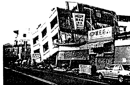
Photo 10 The low-rise building (Fengyuan City, Taichung County) The wall was distributed irregularly even in the low rise, and there was heavy damage in the building with small walls on first floor.
