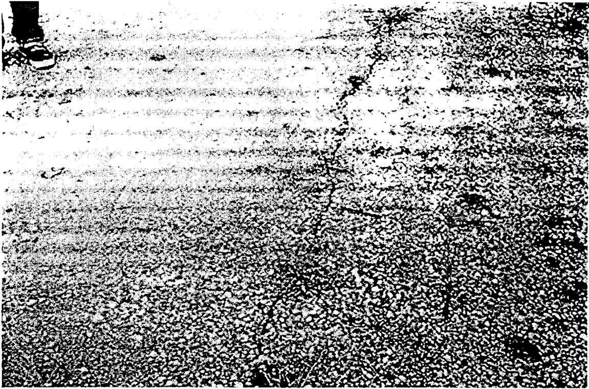
Figure 3. Longitudinal crack near the edge of the crest of Gokce Dam on the upstream side. The location is about at the middle of the dam. The width of the crack was about 7 mm at its greatest
