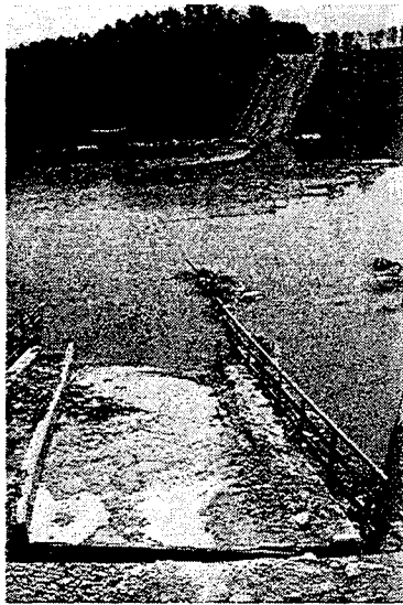
Photo 8 Collapse of Sakarya Central Bridge
