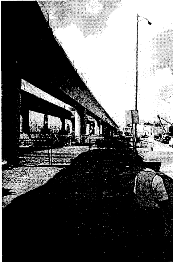
Figure 6: Elevated guideways under construction in Bayamón.
