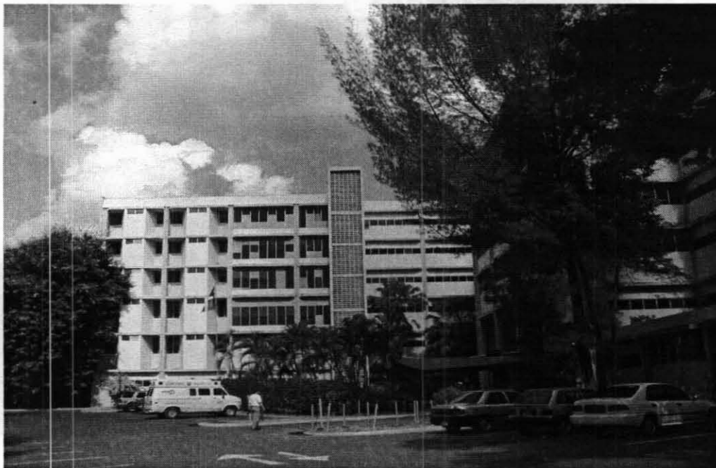
South Wing of Hospital
