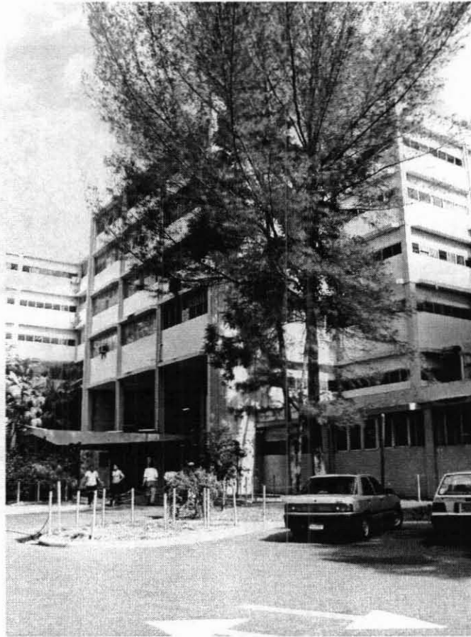
View from the rear of Hospital
