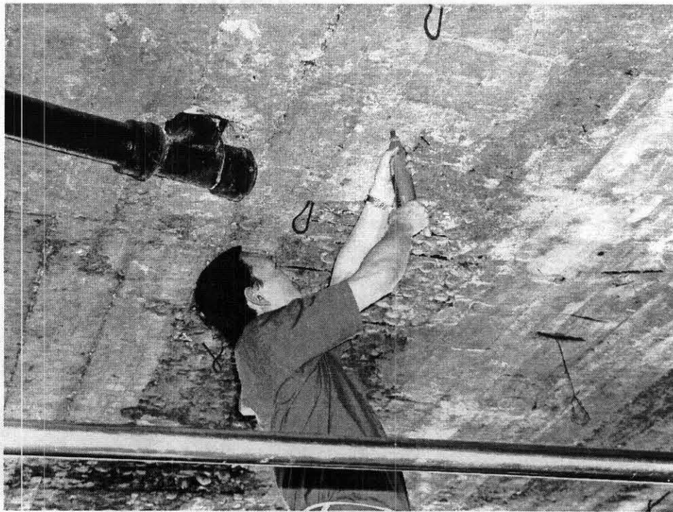
Bottom of Second Floor Slab.
