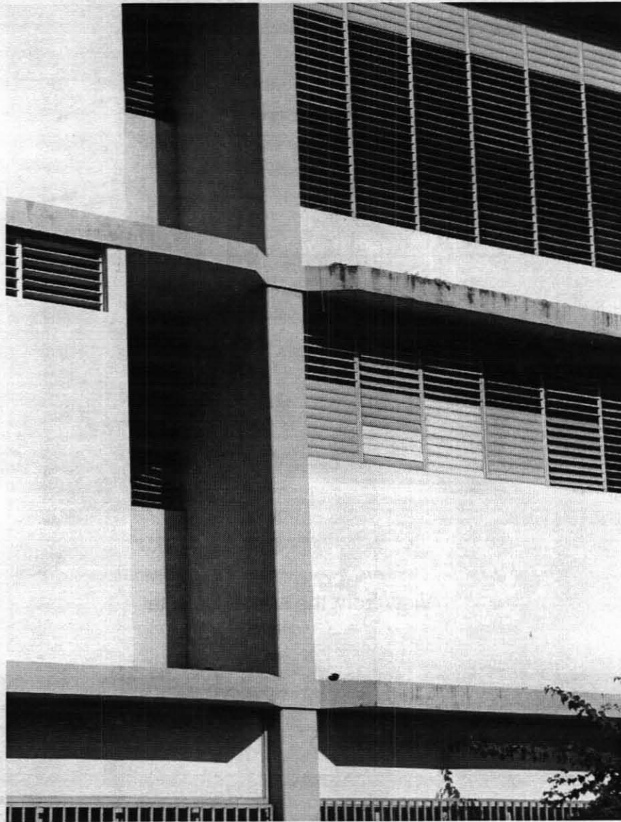
Detailed view of louvers
