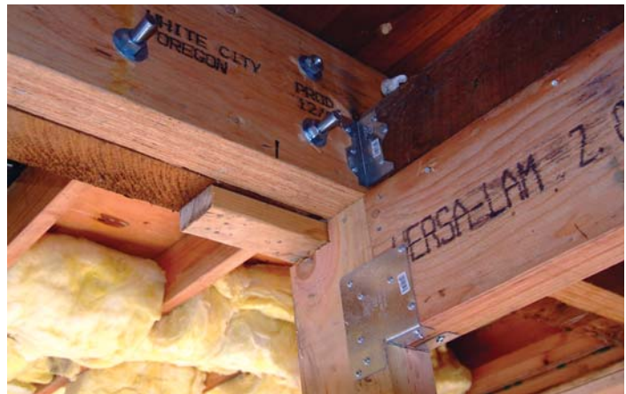
Napa, CA, Feb. 14, 2006 - A home is retrofitted with earthquake straps and bolts to prevent movement in the event of an earthquake (Photo credit: FEMA).
