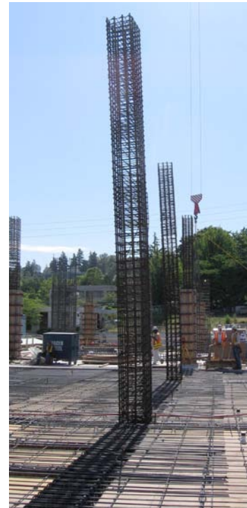
Figure 7-6 – Longitudinal column reinforcement spliced every other floor to reduce congestion.
