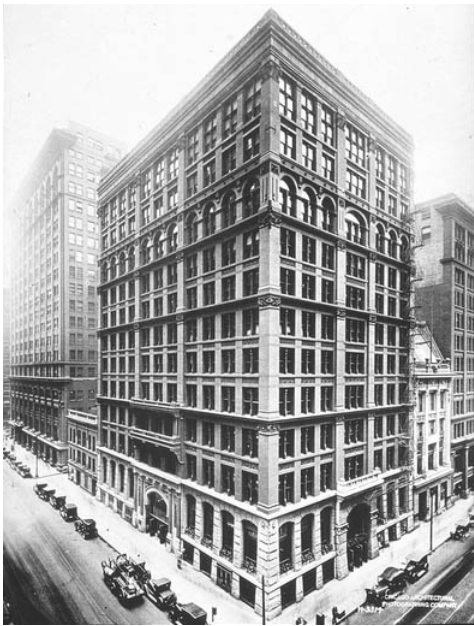
Figure 2-1 - The Home Insurance Building – Chicago, IL, 1885, an early skyscraper.
