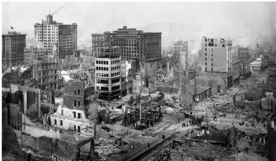
Figure 2-5 - Steel frame buildings in downtown San Francisco performed well in the 1906 earthquake.
