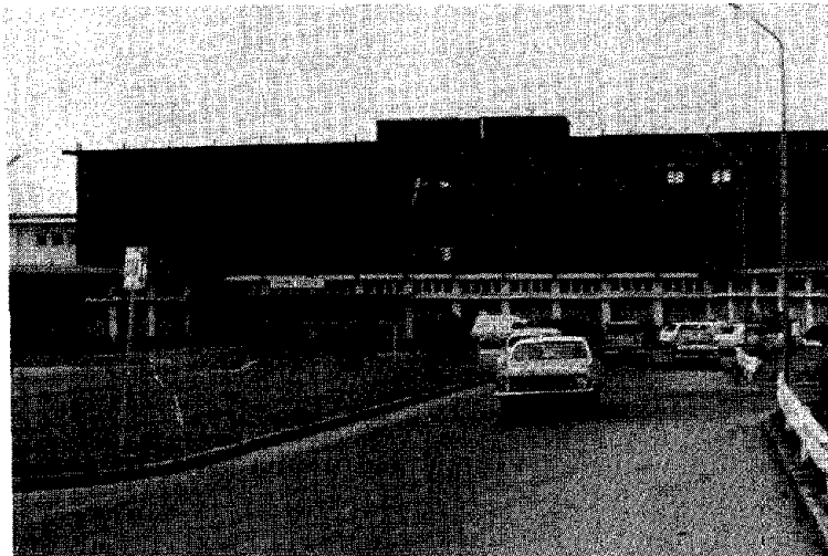
Fig. 26. Darwin Hospital - Larrakeyah
