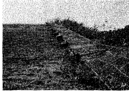
Photo-19. Damage of net fence
