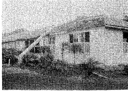
Photo-13. Damage to arc lamp standard (Mihara Junior High School)
