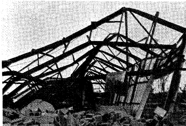
Fig. 30. Industrial building - Winnellie
