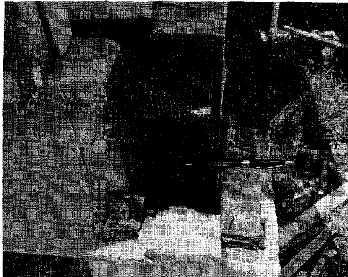
Fig. 15. Beam to column connection - precast concrete high-set
