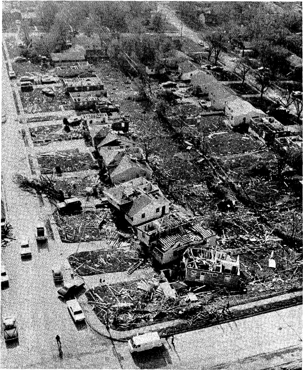
Figure 1. Row of houses twisted off foundations (courtesy R. Paskach, Omaha World-Herald).
