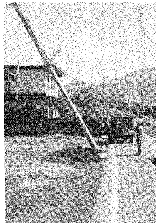
Photo-17. Damage to telegraph pole
