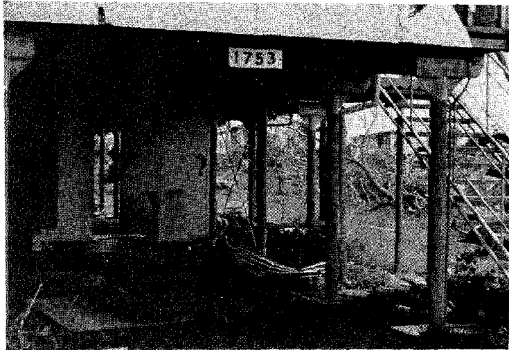
Fig. 4. Pipe columns used in older construction
