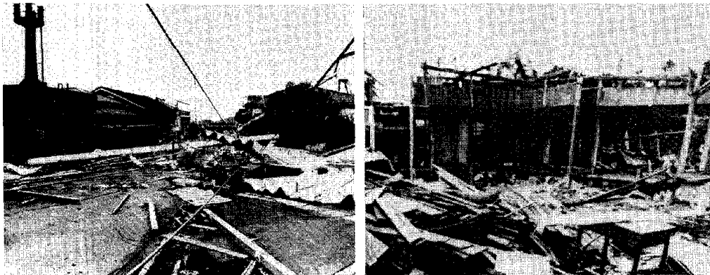
Photo. 2 Examples of houses damage on Hachijojima.
