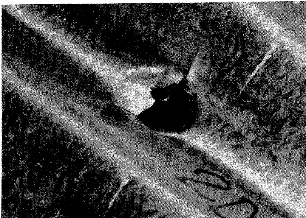
Fig. 32. Typical fatigue failure of CGI cladding
