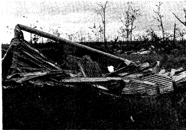
Fig. 34. Failure of lamp standard due to debris loading
