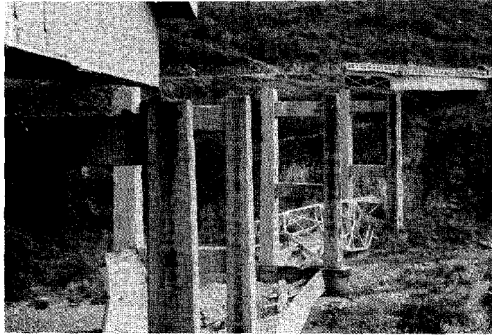
Figure 9 Agua Caliente - View from East Abutment
