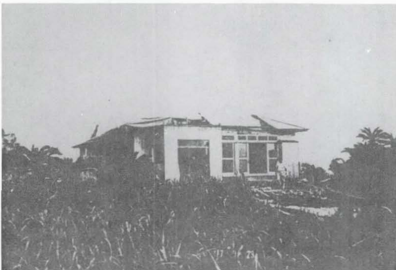
PHOTO 14: ROOF DAMAGE INDUCED BY THE BREAK OF EXTERIOR WALL OPENINGS (IN FRONT)
