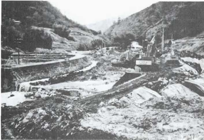
Photo 2. Sludge Removal from the Mochikoshi River
