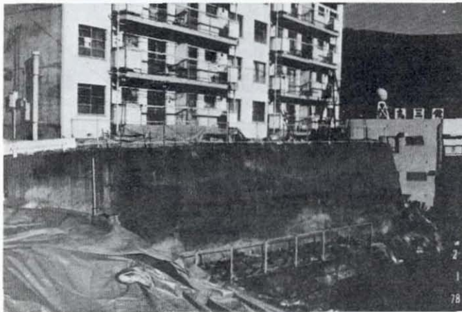
FIGURE 36: THE DAMAGED RETAINING WALL AND 4-STORY APARTMENT HOUSE, INCLINED AT AN ANGLE OF 0.5^{\circ} - 1.5^{\circ} (INATORI-REGION)
