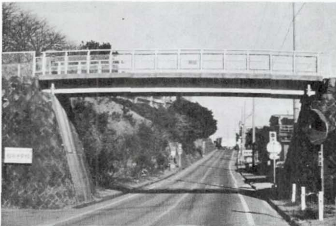
FIGURE 19: OVERCROSSING FOR PEDESTRIAN LOCATED ONLY 20 m FROM FAULTS NEAR INATORI JUNIOR HIGH SCHOOL AT INATORI AREA IN HIGASH-IZU TOWN, WHICH SURVIVED WITH MINOR CRACKS AT PARAPETS
