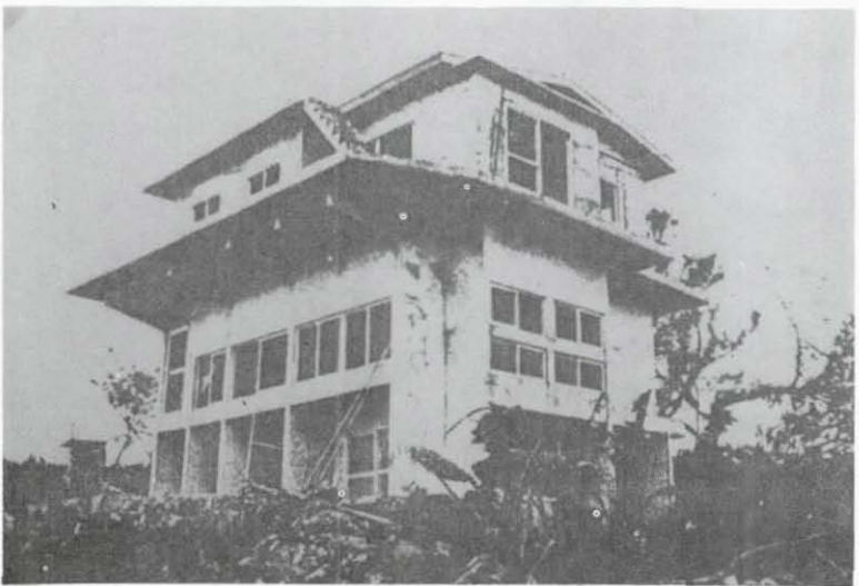
PHOTO 15: DAMAGE TO OPENINGS OF A REINFORCED CONCRETE DWELLING
