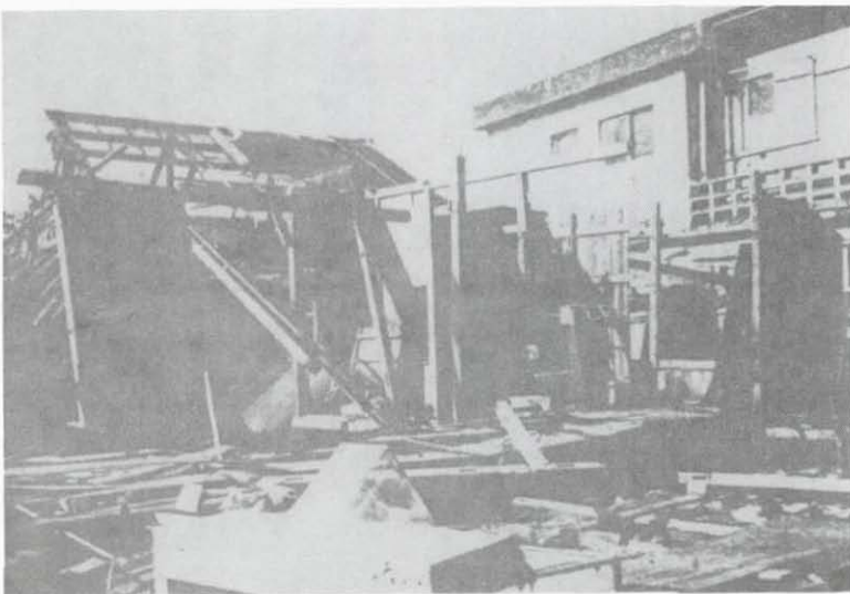
PHOTO 12: TOTAL COLLAPSE OF WOODEN DWELLINGS
