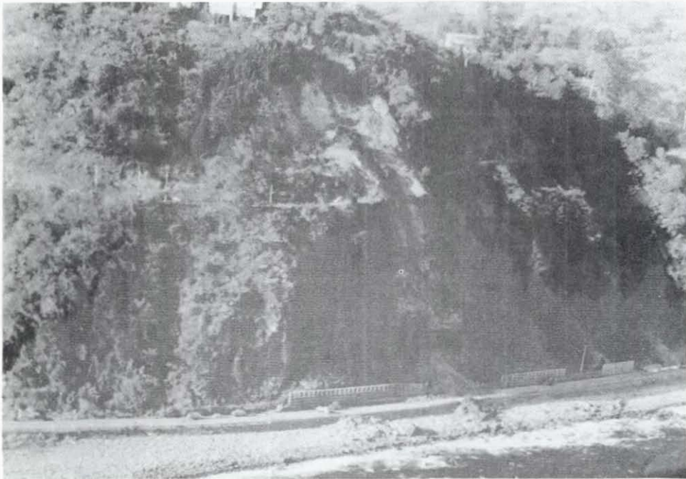
FIGURE 12: SLOPE FAILURE AT OHKAWA AREA IN HIGHSHI-IZU TOWN (ROUTE 135, PHOTOGRAPH FROM SHIZUOKA PREFECTURE)
