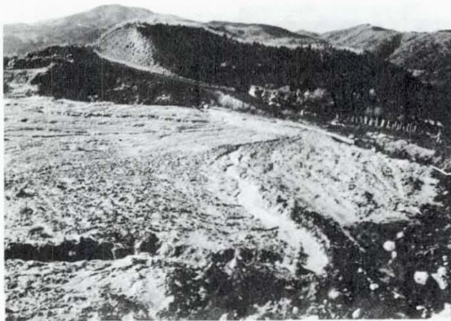
FIGURE 21: COLLAPSED DAM AND TEMPORARY DAM
