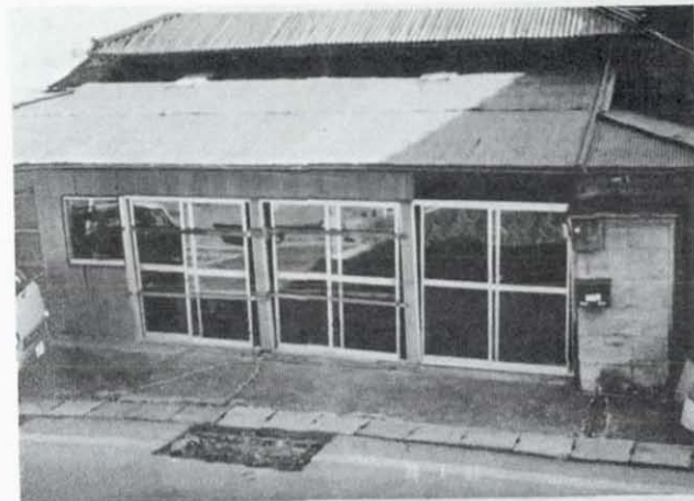
FIGURE 27: FAULT PASSED GROUND UNDER THIS HOUSE (INATORI-REGION)
