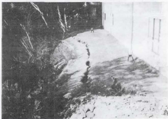
FIGURE 32: CRACKS DUE TO LOOSENESS OF THE STONE WALL (NASHIMOTO-REGION)
