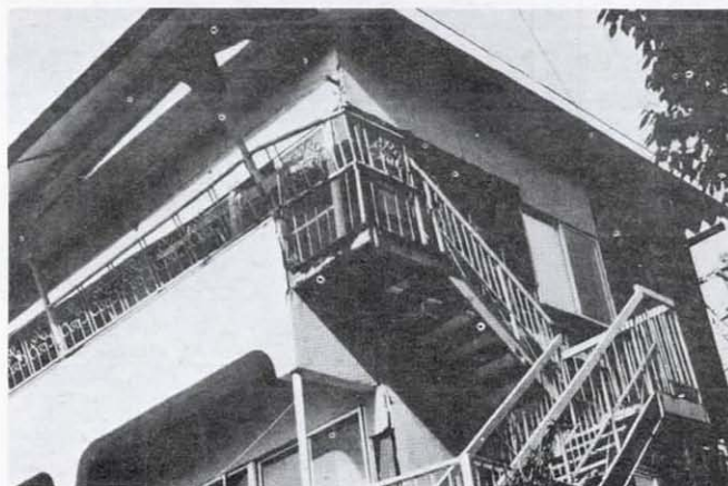
Photo 6. Residential Damage in Shimoda City
