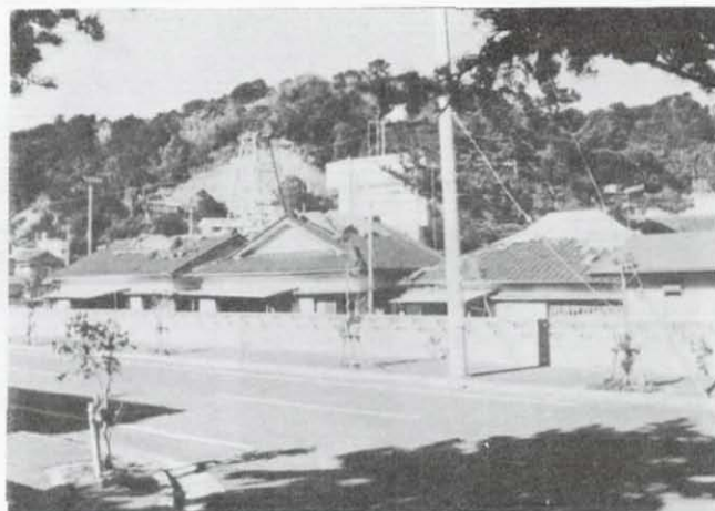
FIGURE 22: ROOF TILES FELL OFF AROUND RIDGES -- SIMILAR DAMAGE COULD BE SEEN EVERYWHERE (KATASE-REGION)
