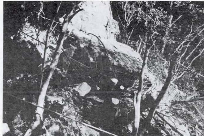
Photo 4. Temporary Countermeasures to Prevent Rock Fall in Shimoda City
