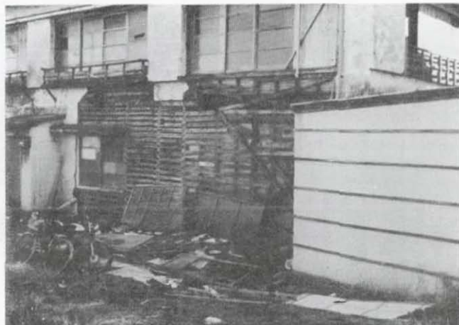
FIGURE 23: ROTTEN EXTERIOR WALLS WERE PEELED OFF (KATASE-REGIONAL)
