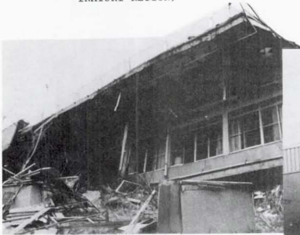
FIGURE 39: COMPLETE COLLAPSE OF STEEL FRAMES (RESTAURANT, INATORI-REGION)
