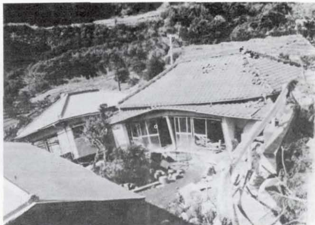
FIGURE 31: HOUSES SWEEPED AWAY AND CRUSHED BY THE FLOW OF EARTH AND SAND (NASHIMOTO-REGION)
