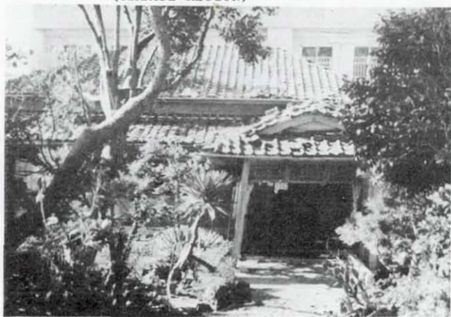
FIGURE 24: LEANING HOUSE, DAMAGE CAUSED BY HEAVY ROOFS AND STRUCTURAL ROTTENNESS (KATASE-REGION)
