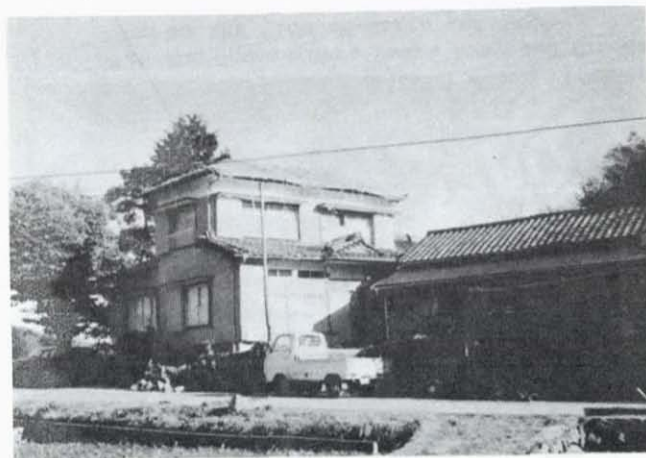
FIGURE 29: NEW HOUSE (THE LEFT-HAND ONE WAS LEANING, AND ITS STRIP FOOTINGS WERE CRACKED) (NEMOTONOTA-REGION)
