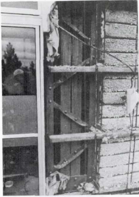
FIGURE 38: DAMAGE OF MORTAR FINISH ON METAL LATHING (HOTEL, INATORI-REGION)
