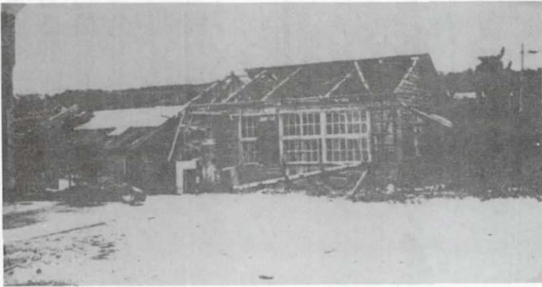
PHOTO 7: GABLE ROOF, HALF OF WHICH WAS BLOWN AWAY
