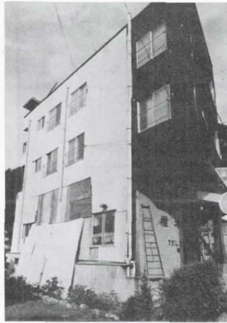
FIGURE 40: DEFORMED COLUMN (ALREADY REPAIRED) (KAWAZU-REGION)
