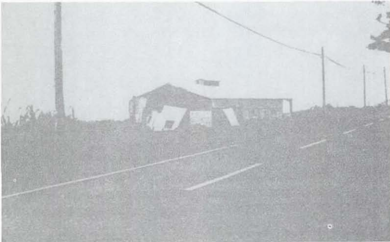
PHOTO 17: DAMAGE TO SLATE SIDING OF A STEEL FRAME FACTORY
