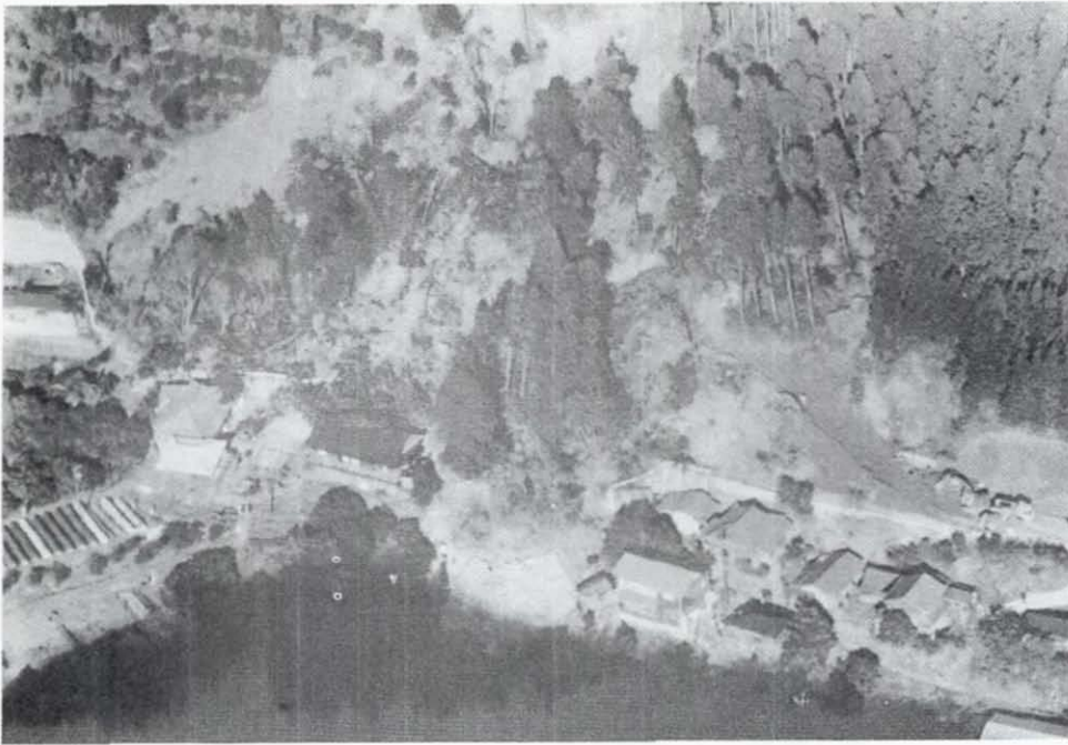
FIGURE 11: SLOPE FAILURE AT NASHIMOTO AREA IN KAWAZU TOWN (SHUZENJI-SHIMODA ROUTE, PHOTOGRAPH FROM SHIZUOKA PREFECTURE)
