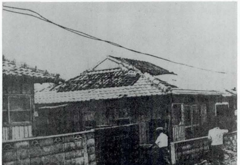
PHOTO 6: DAMAGE TO TILE-ROOFING WITHOUT BED BOARDS
