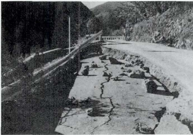
FIGURE 13: SETTLEMENT OF EMBANKMENT IN YUGANO AREA (SHUZENJI-SHIMADA ROUTE)
