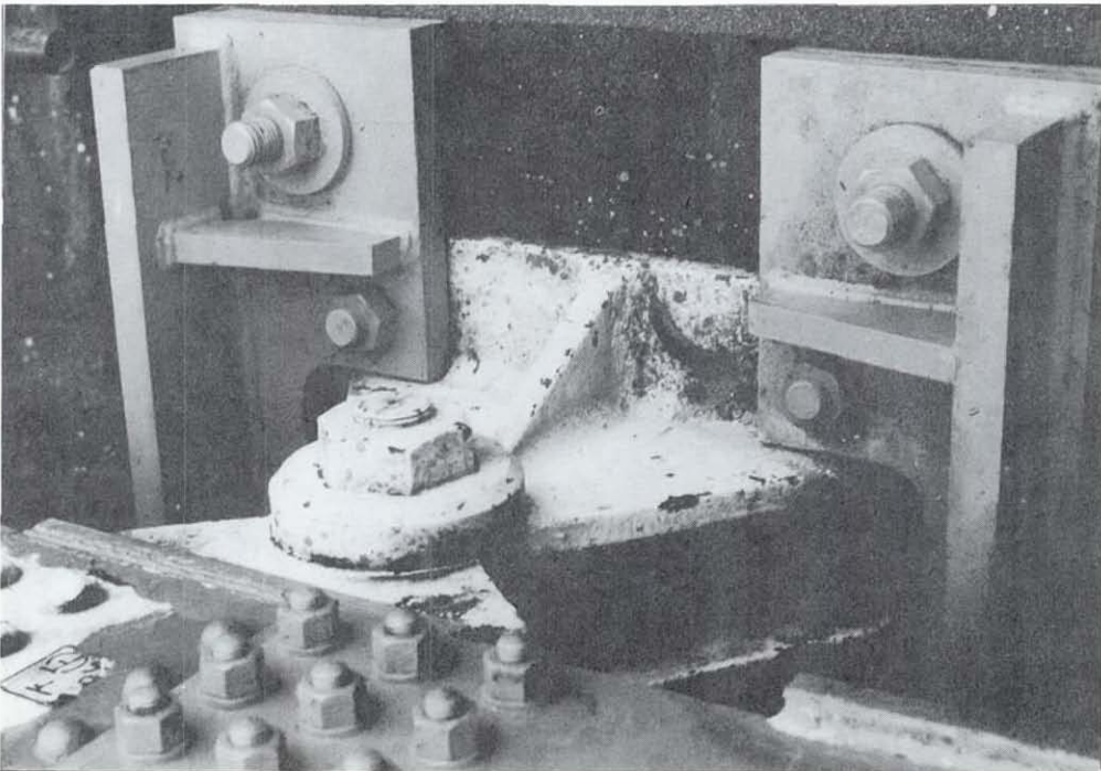
Figure 7.10 Kin-noh Bridge. Bearing restraining device used on the repaired bearing supports of the truss spans. The restrainers were placed before the June 12 event.
