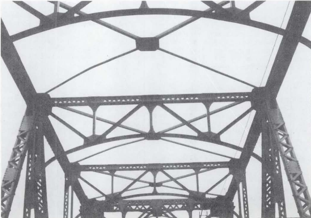
Figure 7.42 Maiya Ohashi Bridge. Buckled lateral bracing of the overhead truss.
