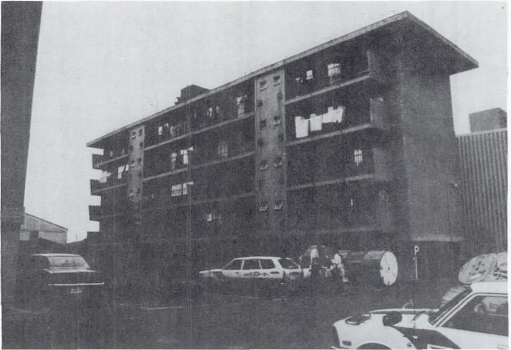
Figure 5.46 Apartment building adjacent to Yazaki Industries warehouse building to the south. The building was undamaged.
