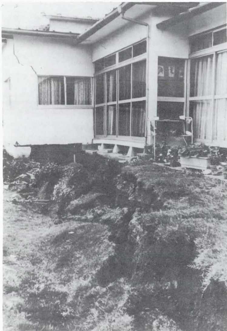
Figure 5.84 Sendai. Damage to single family residence due to loss of foundation support. (Japan National Land Agency photograph)
