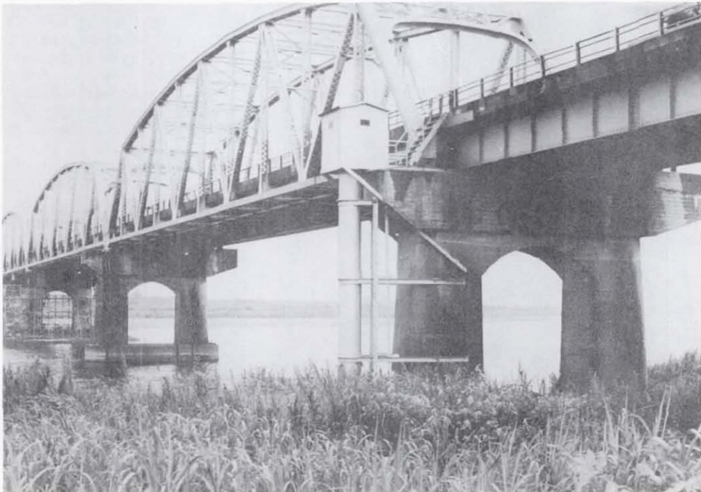
Figure 7.28 General view of the Abukuma Bridge. Note the trace of pier cracking on the pier in the foreground and scaffolding at and surface preparation of the pier in the background.
