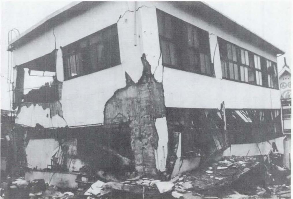
Figure 5.47 Paloma Building - Viewed from the east. Collapse occurred at the east end of the building.
