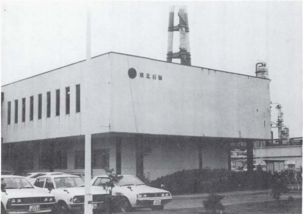
Figure 6.49 Sendai Refinery, Tohoku Oil Company, Ltd.: A wing of the damaged steel-framed administration building. Damage was obvious only to the architectural finishes.
