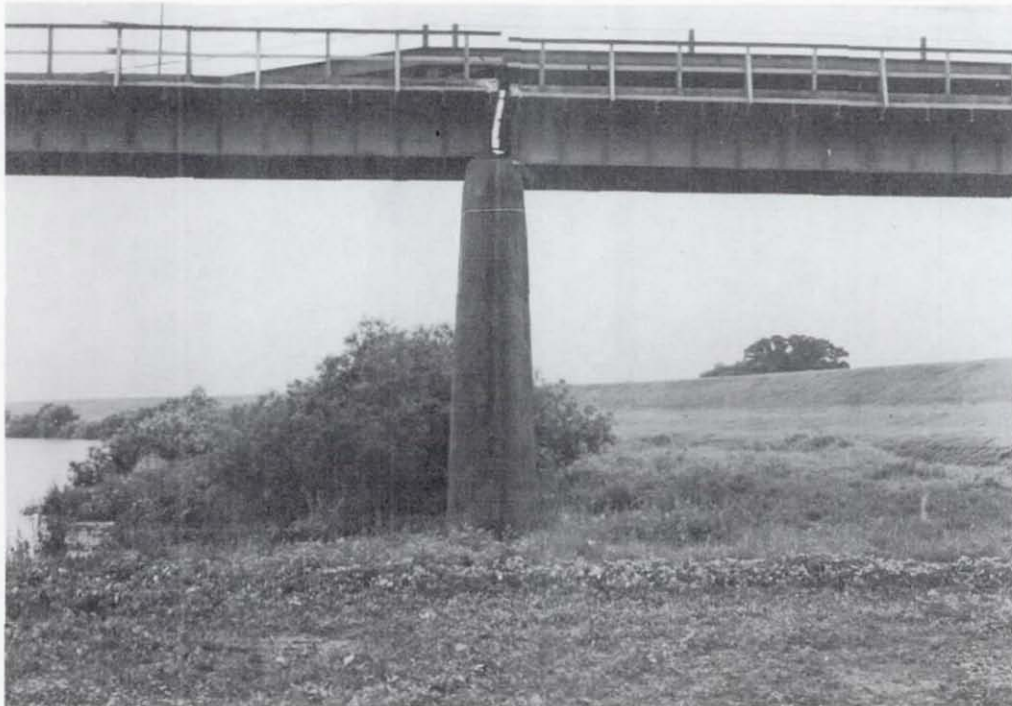
Figure 7.38 Longitudinal displacement of superstructure. Note the temporary structure which spans the dislodged main span.
