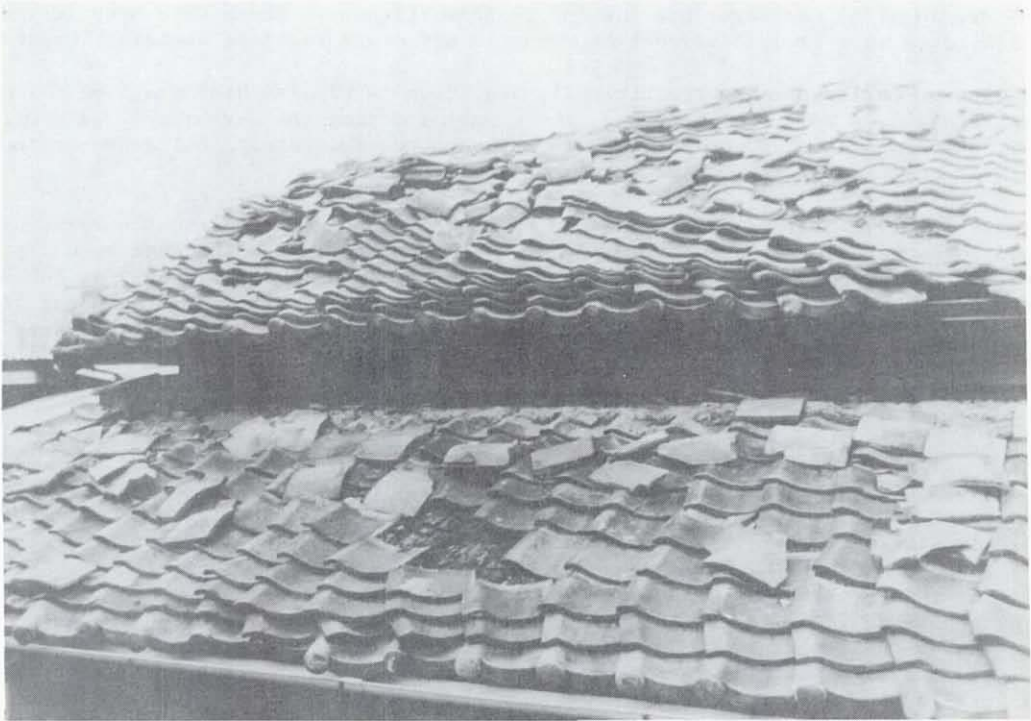
Figure 5.86 Typical damage to tile roofs in Sendai (Japan National Land Agency photograph)
