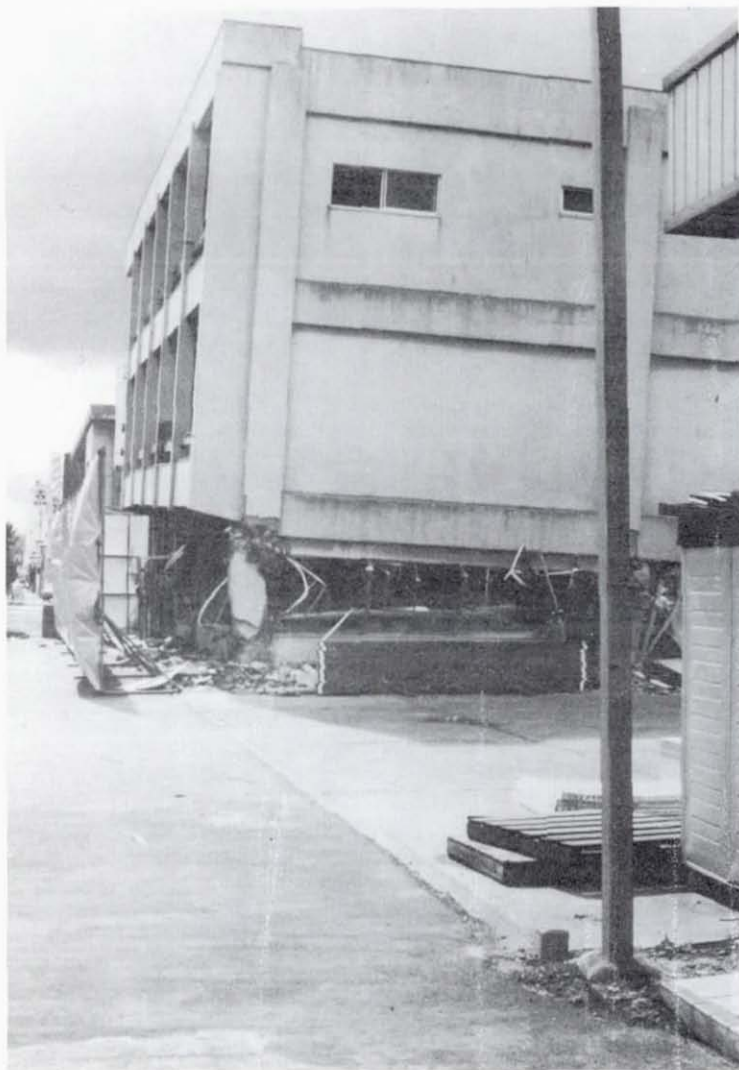
Figure 5.24 Maruyoshi Building, view from the east. Failure of first story columns occurred in shear.
