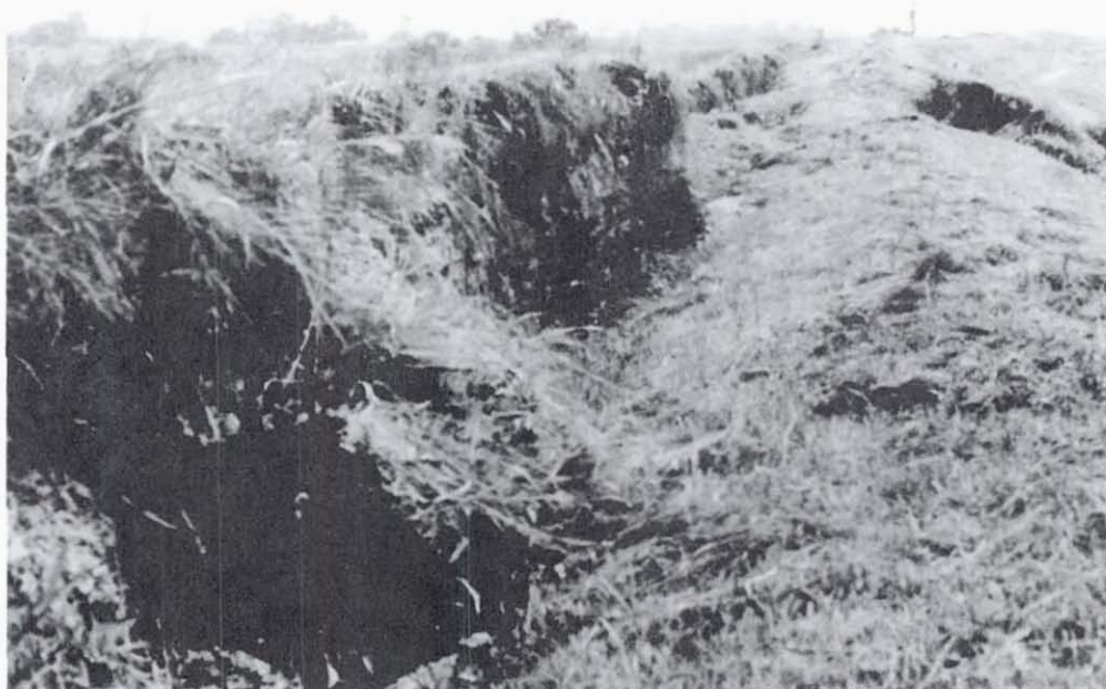
Figure 8.12 Site 3, Yoshida River. Scarps in dike caused by slumping. Note man in background for scale. (Photo courtesy K. Kawashima, PWRI)
