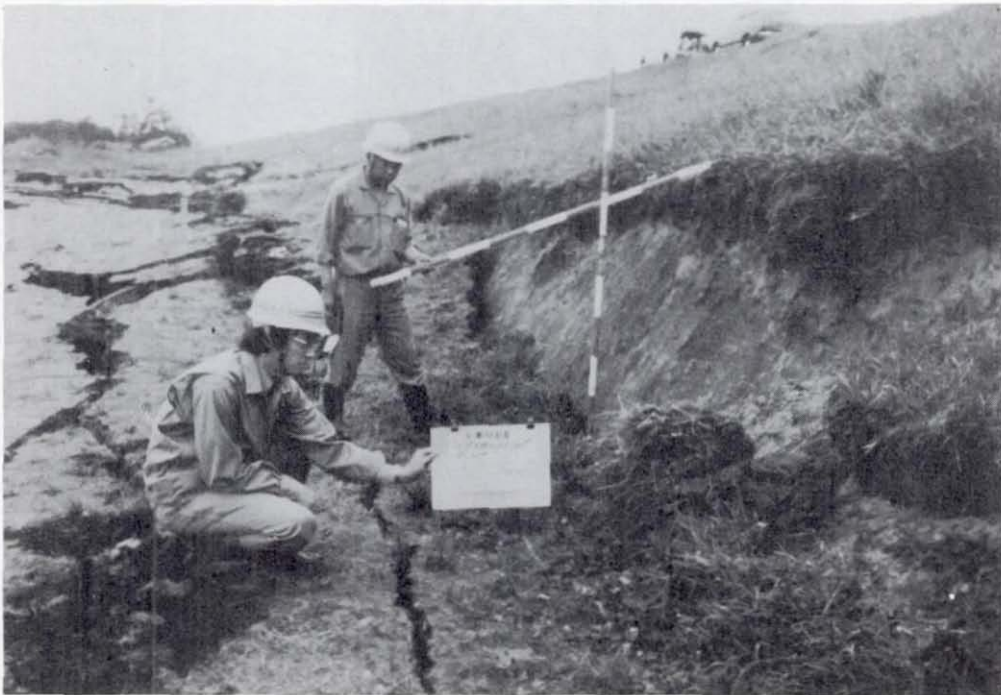
Figure 8.3 Site 1, Natori River. Slumping of dike on flank away from river. View north. (Photo courtesy Tohoku Regional Construction Bureau)
