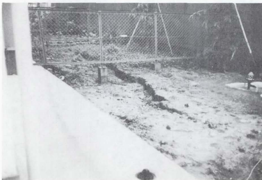
Figure 5.83 Sunny Heights Apartment Building. Ground cracking and settlement adjacent to walkway surrounding the building.
