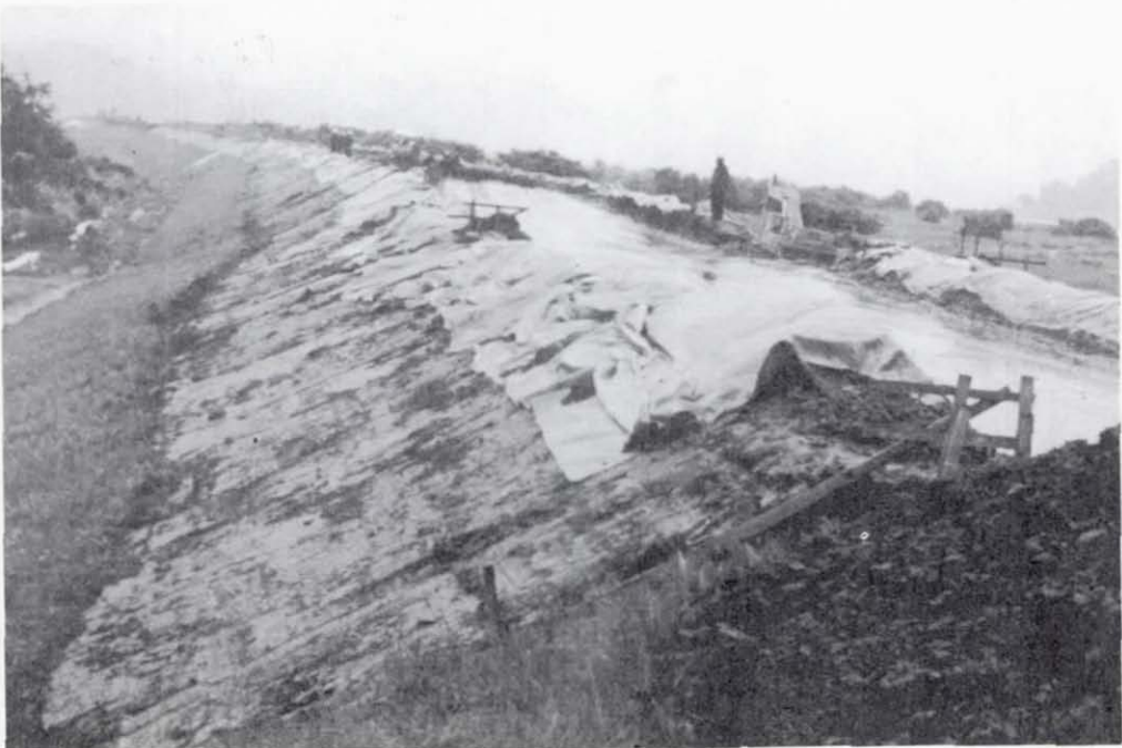
Figure 8.17 Site 6, New Kitakami River. View east along crest of dike and highway that are being repaired. Uneven nature of highway surface is due to liquefaction-induced differential settlement. Settlements of up to 1.5 m occurred along a distance of 4 km.
