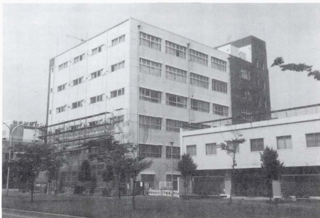
Figure 5.35 Maruhon Building, west face, showing cracking of curtain wall panels.
