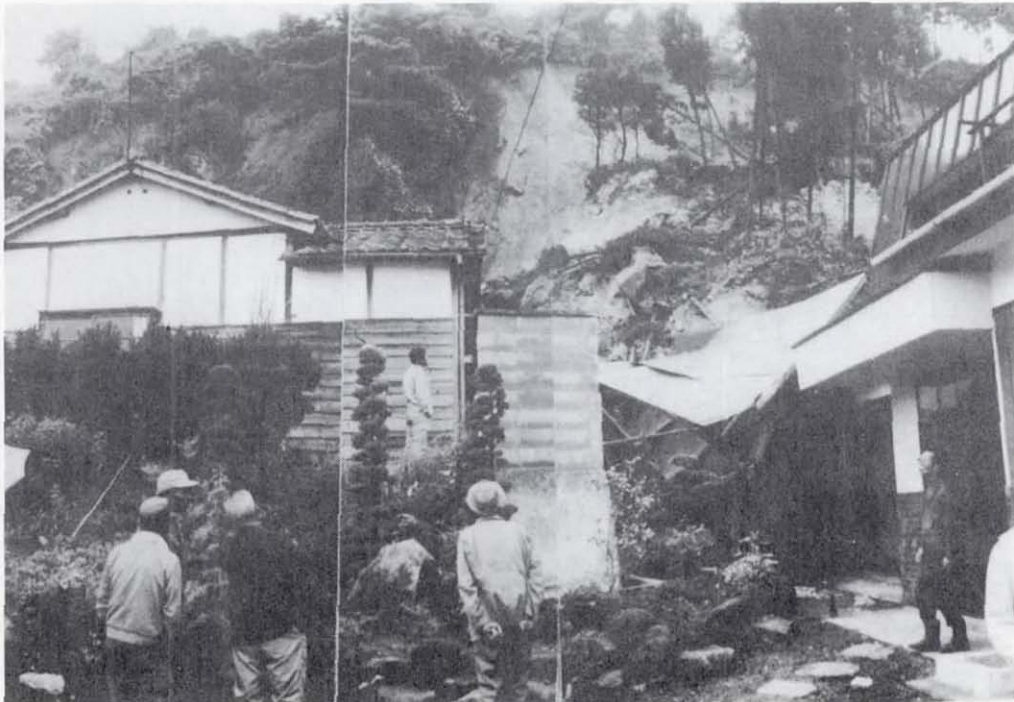
Figure 9.3 Closeup of rock fall damage to houses shown in left portion of figure 9.2. (Photograph courtesy of Y. Tsuruya)
