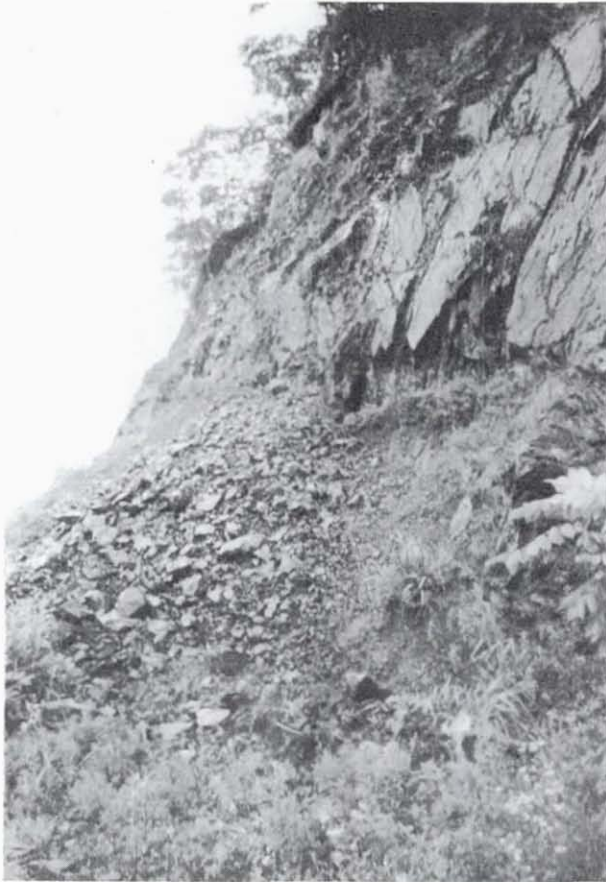
Figure 9.15 Rock fall in roadcut. Note slaty cleavage planes that form the rock fall scarp.
