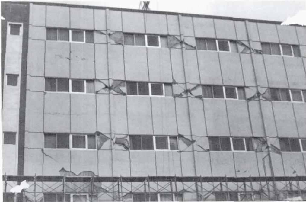
Figure 5.36 Maruhon Building, west face. Detail of the damage to panels between windows.
