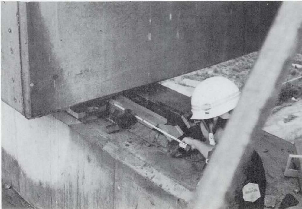
Figure 7.54 Failure of a bearing plate supporting a single cell box girder near the Higashi Sendai Construction Office. Girder displaced laterally 50 cm.
