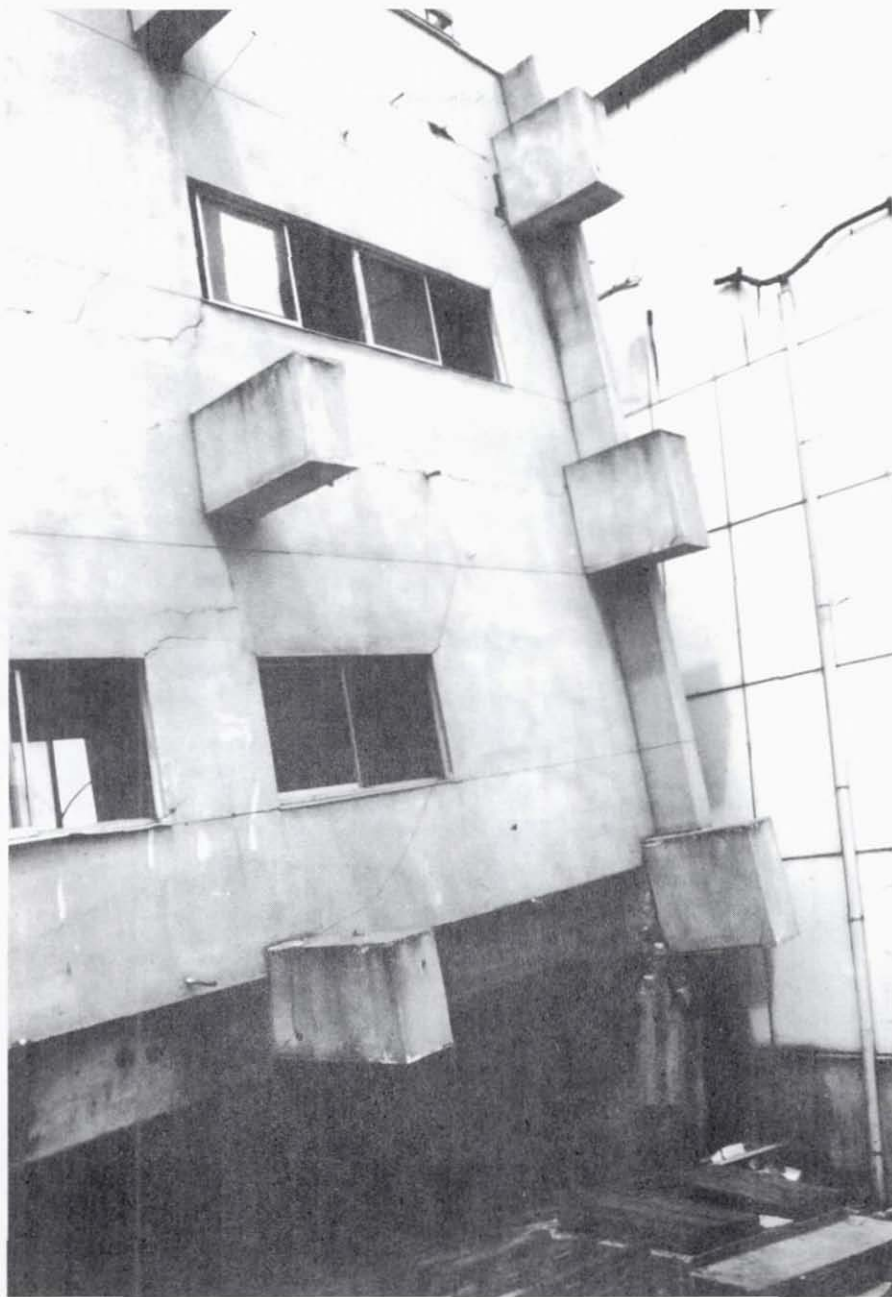
Figure 5.31 Obisan Building, south face. Walls above first story remained essentially intact.
