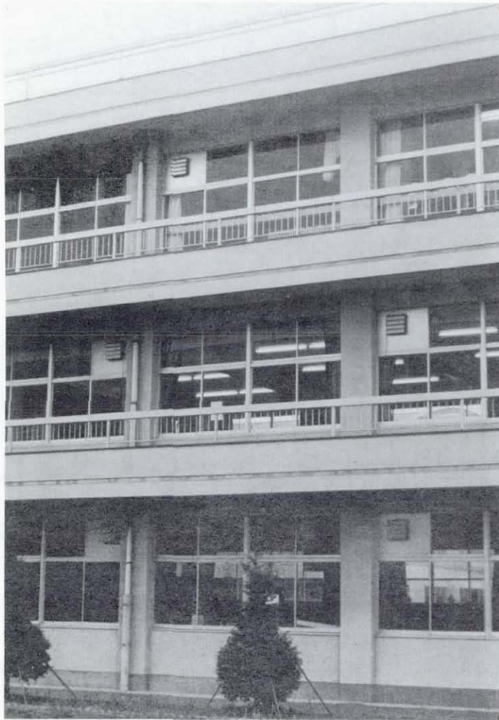
Figure 5.62 Izumi High School, typical classroom building, south face. This side of the building, which is relatively open, suffered little damage.
