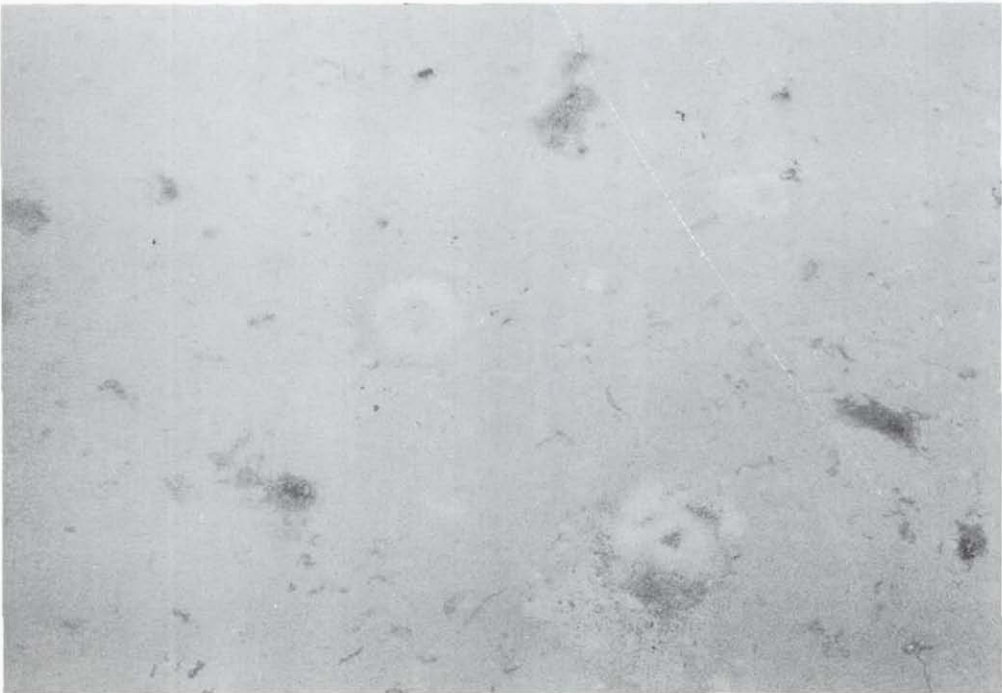
Figure 7.12 Yuriage Bridge. Liquefaction in the flood plan below the bridge.
