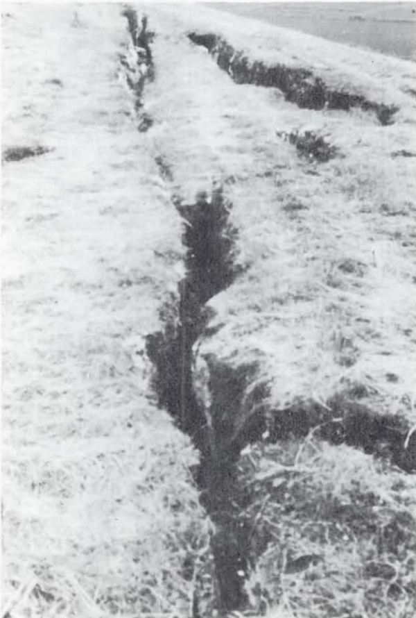
Figure 8.10 Site 3, Yoshida River. View east (downstream) along section of dike where repairs are underway. Dike crest settled as much as 1 m over a length of 5 km. Sand bags have been placed as part of repair process.
