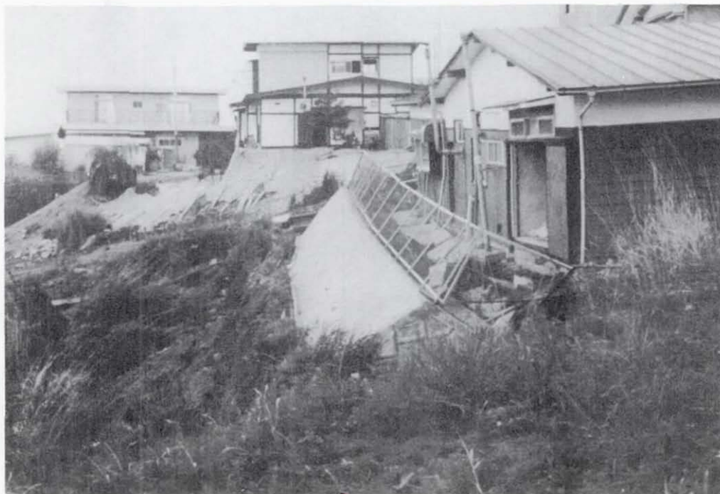
Figure 9.18 House near head of slump. House was removed due to undercutting by headwall scarp (Photograph courtesy of Y. Tsuruya).
