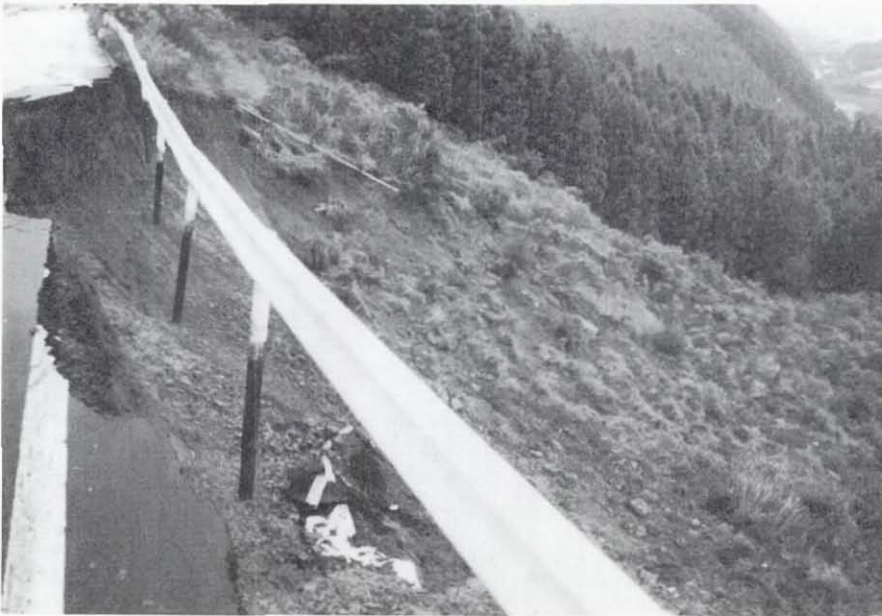
Figure 9.16 Slump in artificial fill along a highway on the Ajika Peninsula.
