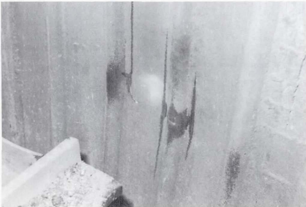
Figure 6.19 New Sendai Power Plant, Tohoku Electric Power Company: a view of the exterior of the boiler walls showing evidence that the suspended boiler had pounded against the surrounding support structure. (Tohoku Electric Power Company photograph)
