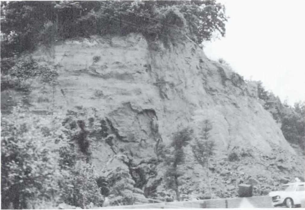
Figure 9.14 Rock fall from roadcut in weakly cemented sandstone.
