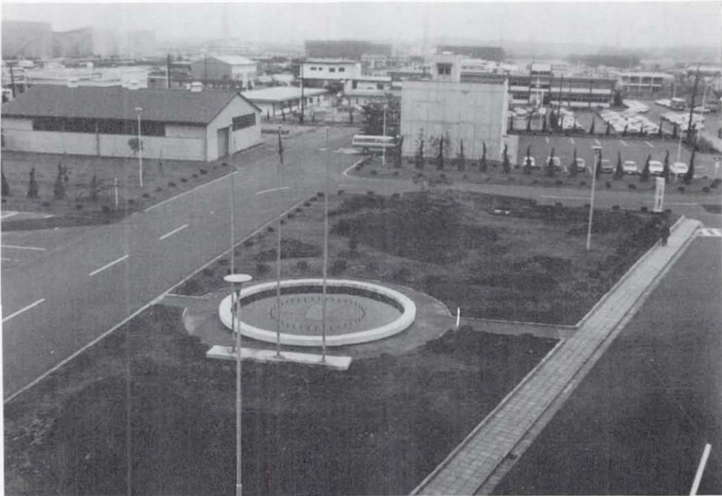
Figure 6.14 New Sendai Power Plant; Tohoku Electric Power Company: A view of the entrance area to the power plant showing settlement of fill and subsequent repair work to the pavement. The pavement settled approximately 15 cm (6 in) and was primarily in the vicinity of a backfilled underground pipeline.
