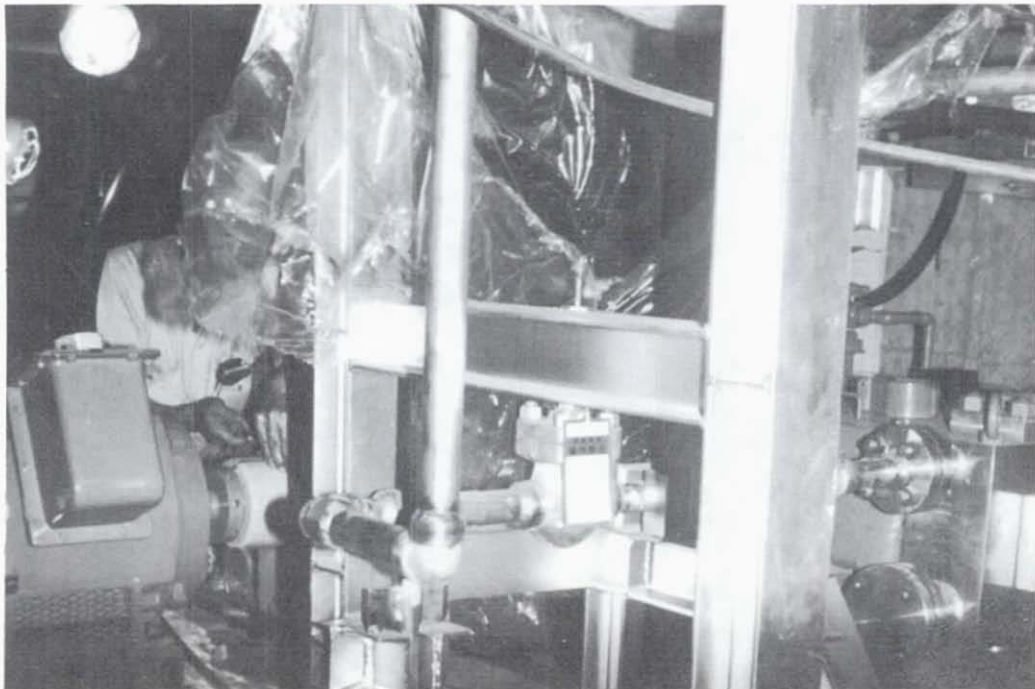
Figure 6.8 Fukushima Nuclear Power Plant: a typical view of massive seismic and/or pipe whip bracing of critical piping inside the reactor building of Unit 6. The equipment showed no evidence of damage. This unit is still under construction.
