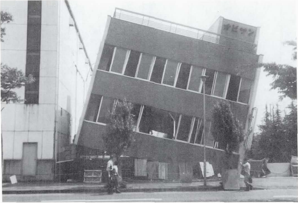
Figure 5.27 Obisan Building, viewed from the North. This three story reinforced concrete frame building had a heavy eccentric stairwell cantilevered over the column line at the right end of the building.
