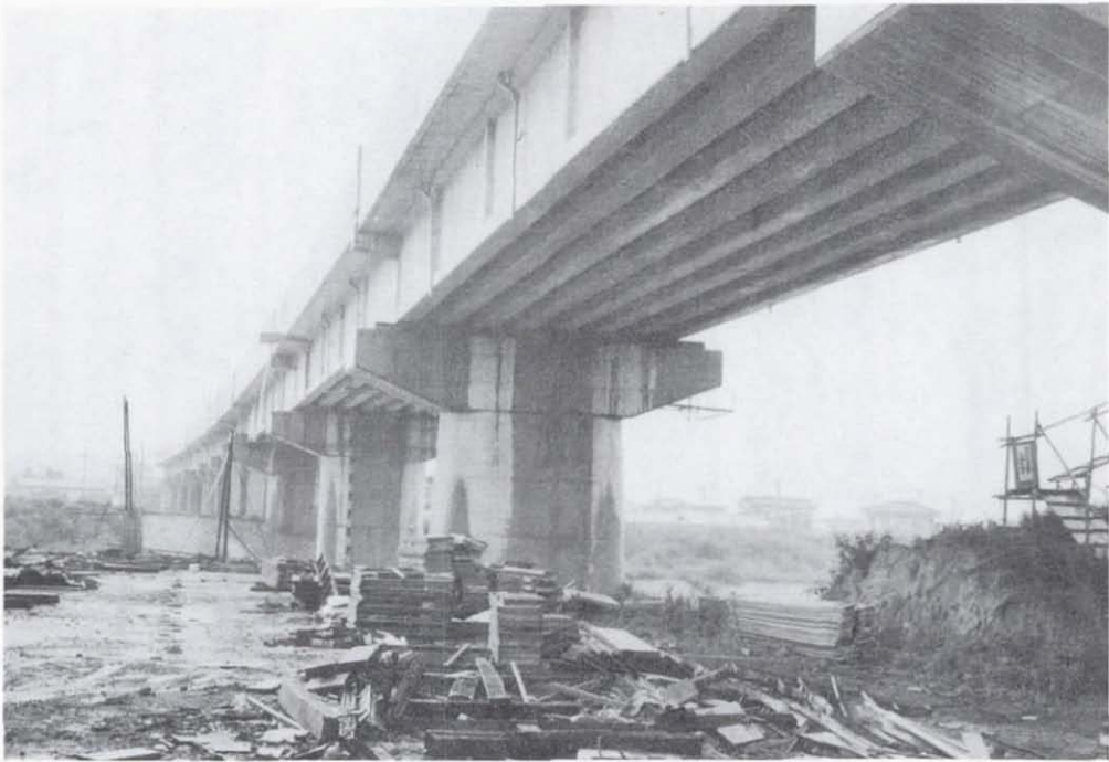
Figure 7.51 Typical structures which experienced pier cracking near the Rifu Construction Office of the Sendai Shinkansen Construction Bureau, JNR.
