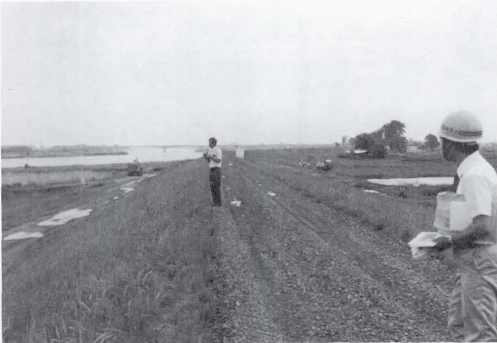
Figure 8.2 Site 1, Natori River, view downstream (southeast) along repaired portion of dike. Dike is made of compacted sand. It rises 2 m above the high water level of the river and has side slopes of 2H:1V. Natori River in center-left background.
