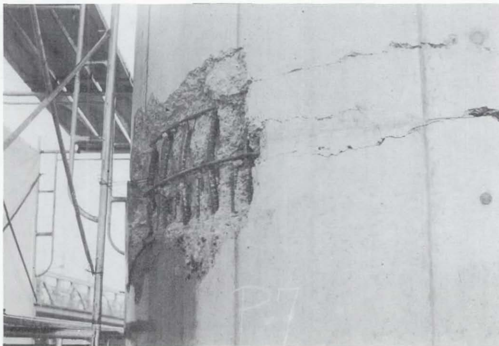
Figure 7.50 Natori River Bridge. Detail of spalled concrete at the Natori River Bridge site showing the buckled vertical rebar.
