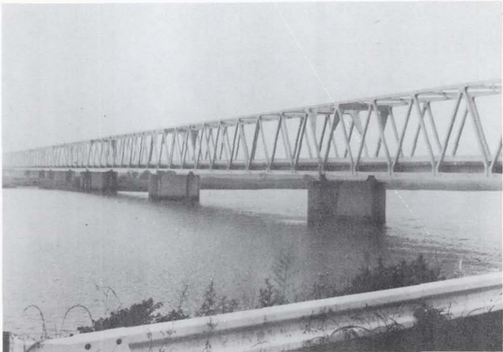
Figure 7.34 Kitakami Ohashi Bridge. No structural damage was reported.
