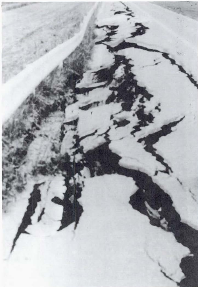
Figure 8.18 Site 6, New Kitakami River. Cracking of dike crest and roadway due to liquefaction-induced slumping. (Photo courtesy K. Kawashima, PWRI)
