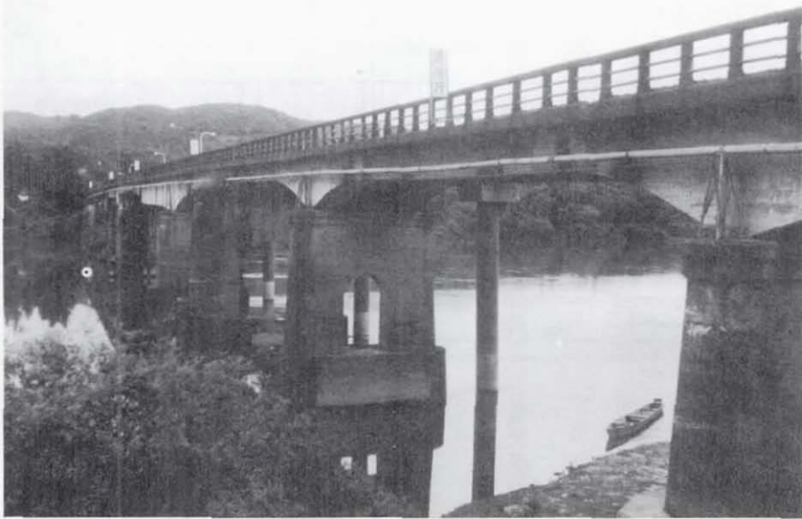
Figure 7.43 General view of the Toyoma Bridge which was closed to traffic. The columns in the background support an independent steel box girder pedestrian structure which was undamaged.
