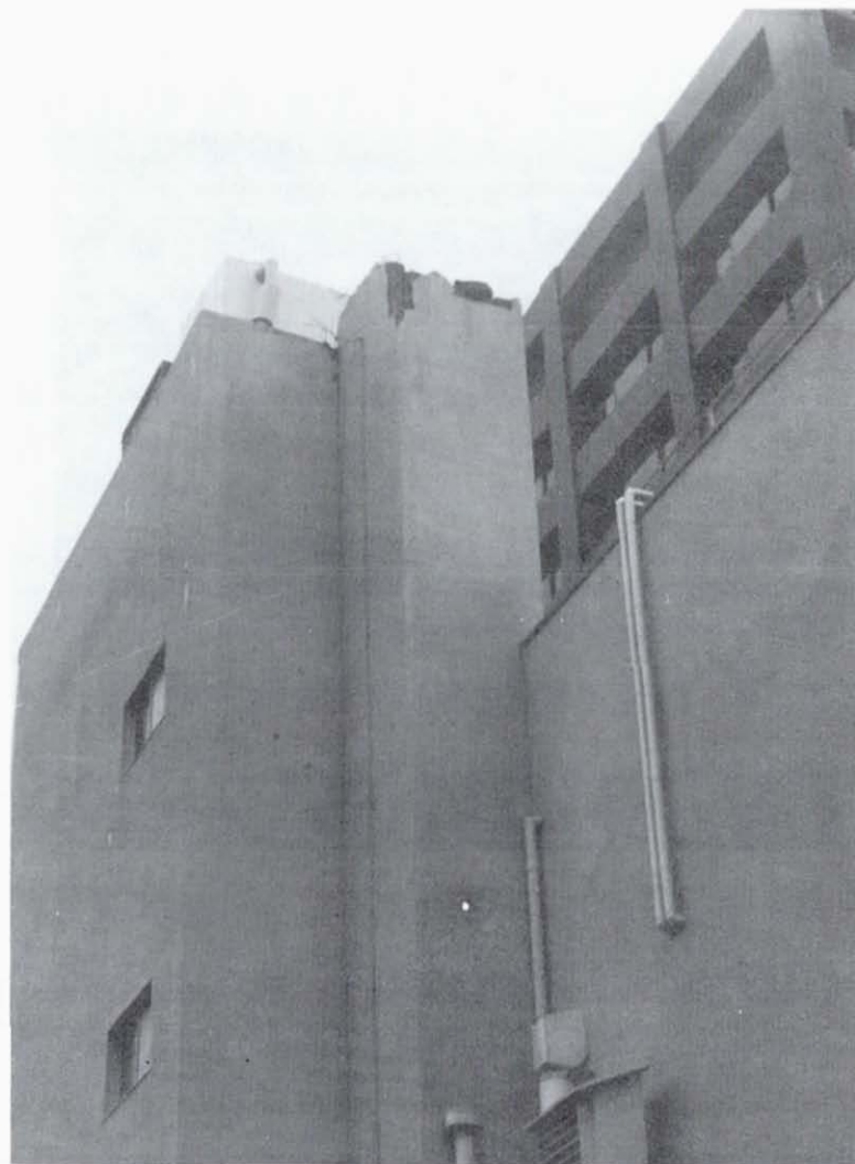
Figure 5.9 Downtown Sendai. Reinforced concrete chimney failure.
