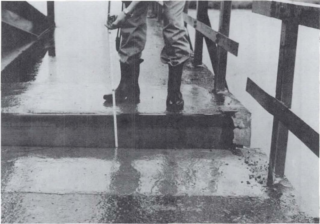
Figure 7.39 Vertical displacement of dislodged span.
