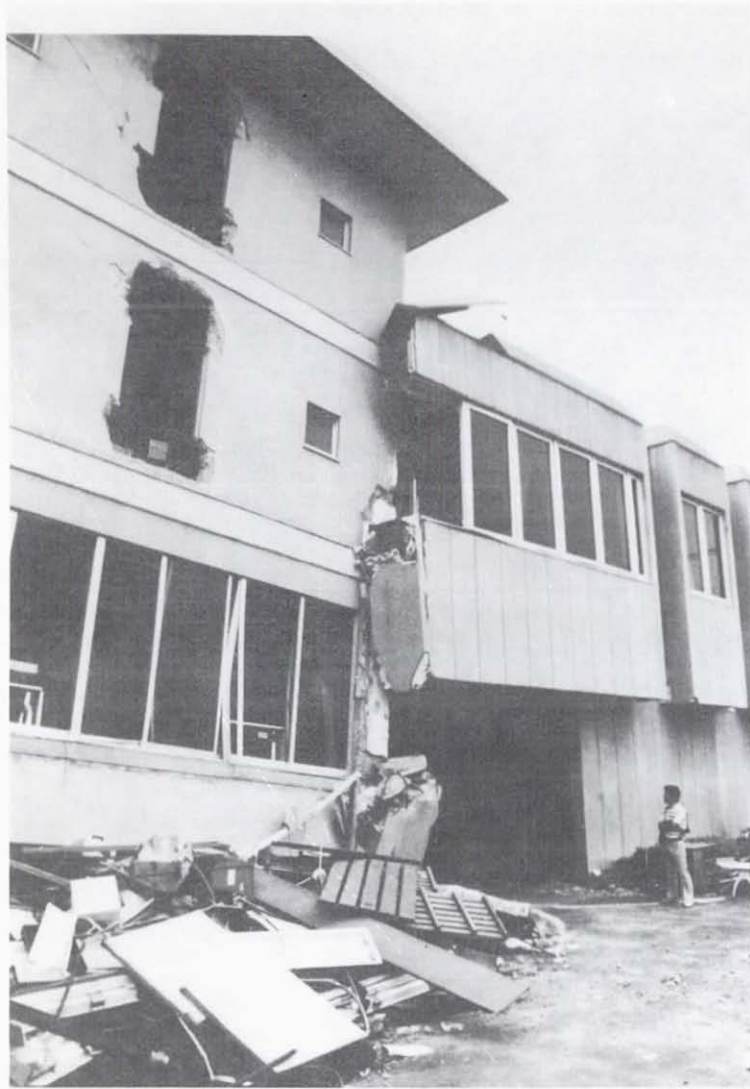
Figure 5.40 Yazaki Industries, showing area of impact between steel and reinforced concrete frames.
