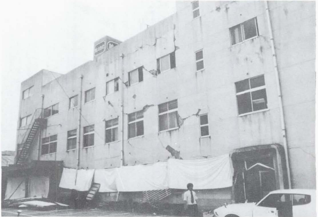
Figure 5.32 Kinoshita Building, Oroshicho area, of Sendai. Extensive diagonal cracking was observed on the east face (rear) of the building.
