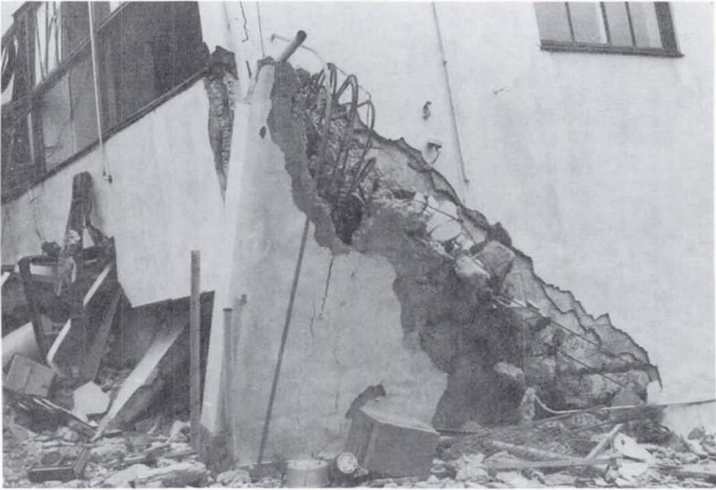
Figure 5.50 Paloma Building, detail of shear wall on west end of building.
