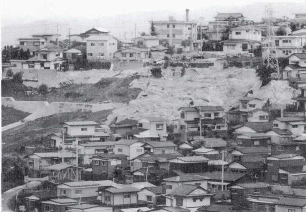
Figure 9.17 Rotational slump in artificial fill in Sendai (area covered by tarps) which destroyed one house and is threatening others. To left of slump is concrete slope protection dam (sabo works).
