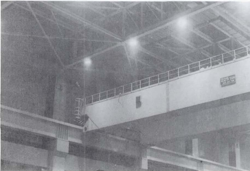
Figure 6.6 Fukushima Nuclear Power Plant: a view of the braced steel frame roof and the overhead crane of the turbine building of Unit 6.
