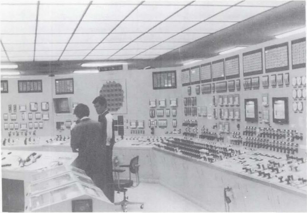
Figure 6.9 Fukushima Nuclear Power Plant: a partial view of the control room of Unit 5. At the time of the visit on June 23, 1978, 11 days after the earthquake, this unit was operating.
