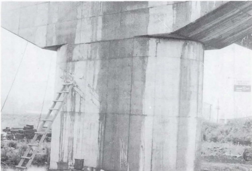
Figure 7.52 Shear cracking in the relatively lightly reinforced upper portion of the pier.
