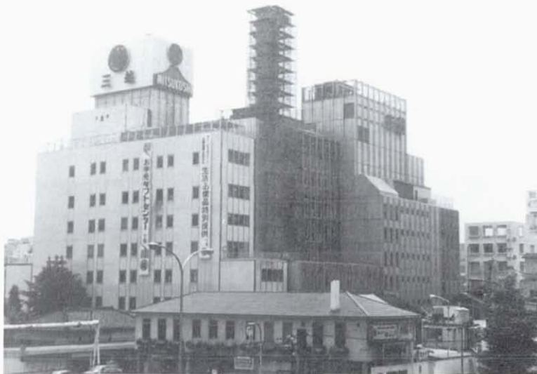
Figure 5.8 Chimney damage to the Mitsukoshi Department store. Numerous such chimneys suffered such damage.
