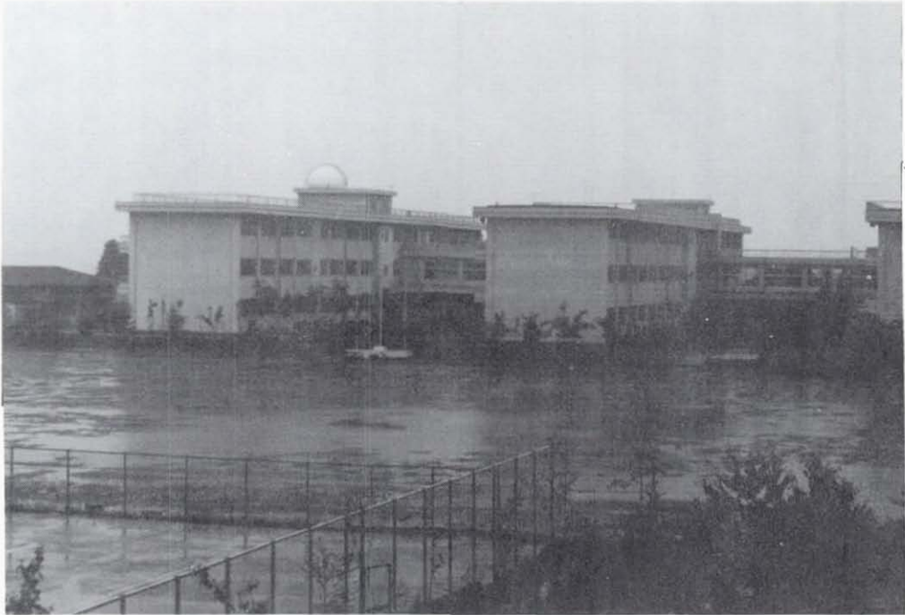
Figure 5.58 Izumi High School. Three adjacent reinforced concrete frame buildings with shearwalls suffered minor damage.
