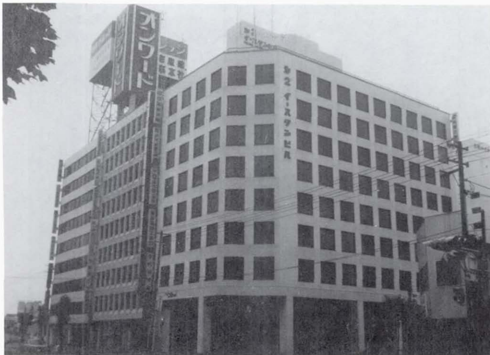
Figure 5.6 Second Eastern Building Company Building, Sendai. A typical modern building in Sendai; the only apparant damage to the glazed tile veneer on the exterior was cracking on spandrels and shear walls.
