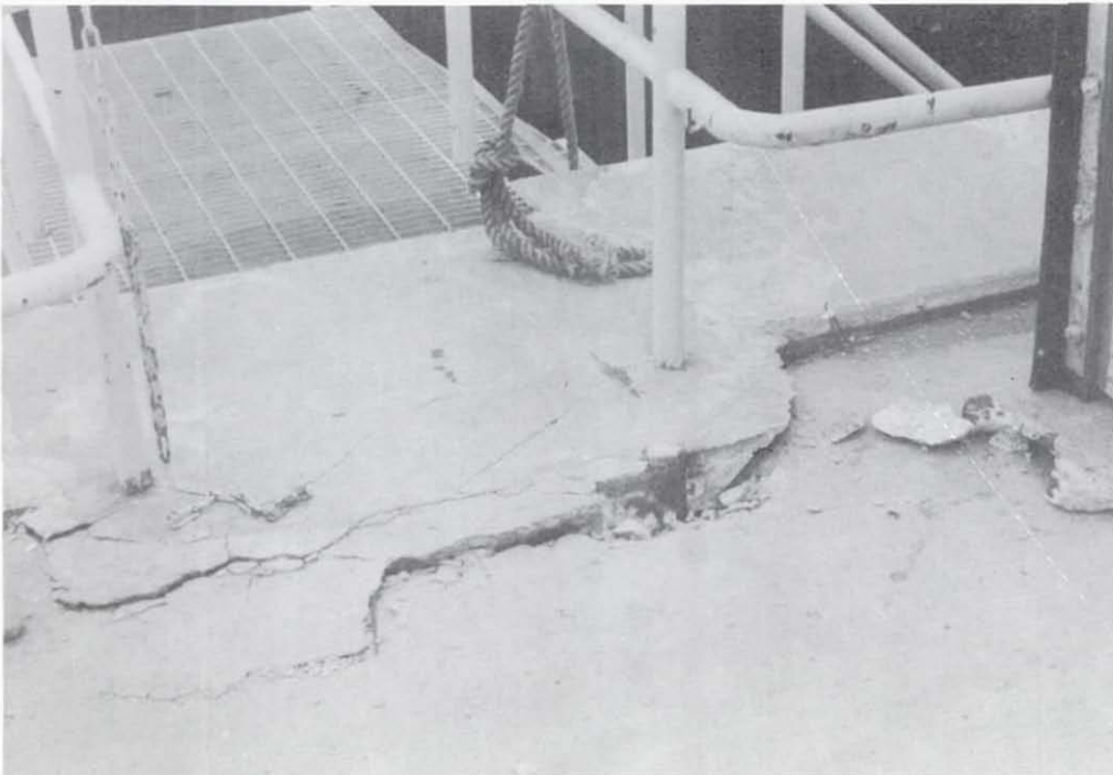
Figure 6.15 New Sendai Power Plant, Tohoku Electric Power Company: damage around the water intake structure from minor settlement. Other examples of minor settlement were observed throughout the site.
