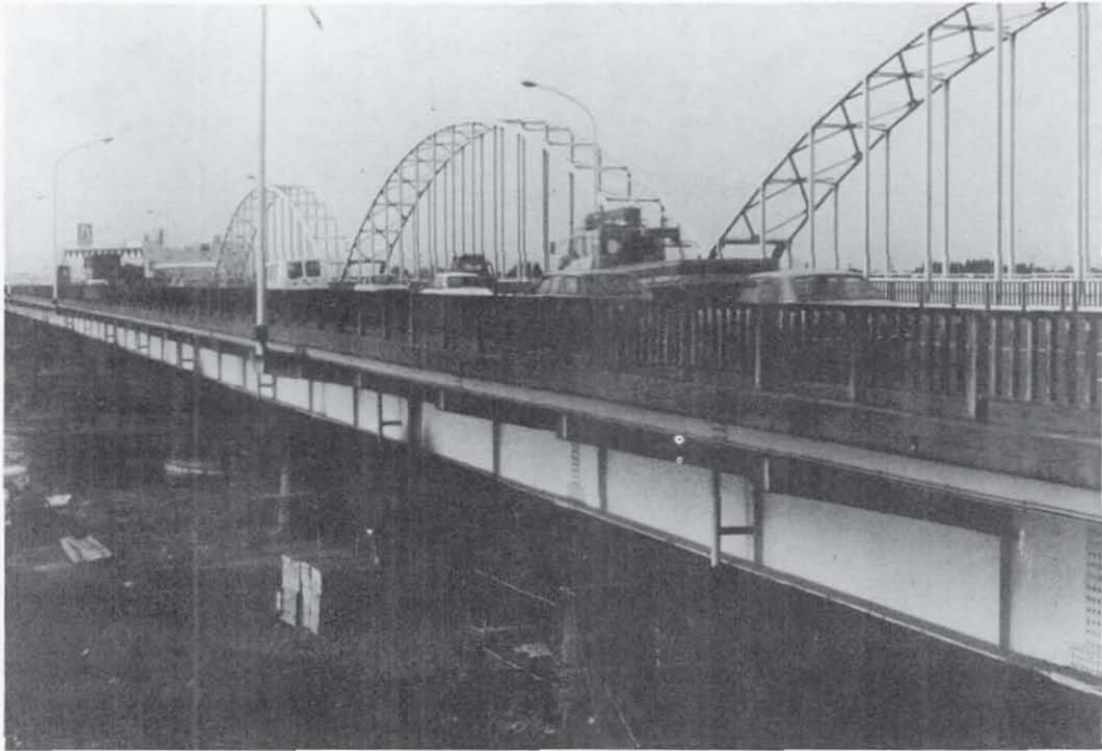
Figure 7.19 General view of the Sendai Ohashi Bridge. The deck arch bridge in the background, which is comprised of two steel plate girders with cross bracing and supported on slender circular columns, carries an industrial water pipeline and was reportedly undamaged.
