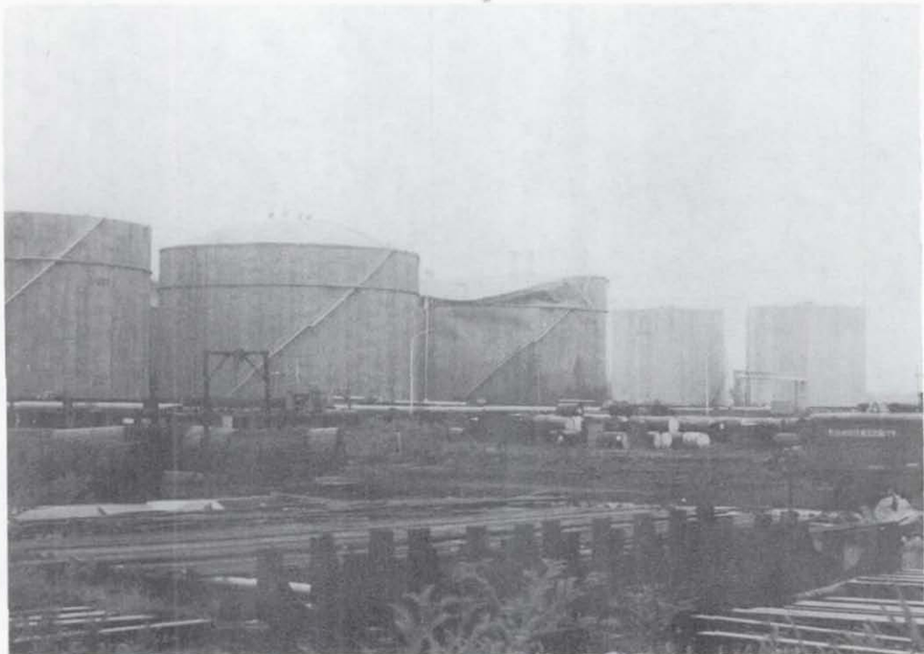
Figure 6.43 Sendai Refinery, Tohoku Oil Company, Ltd. Two other failed TC oil storage tanks.
