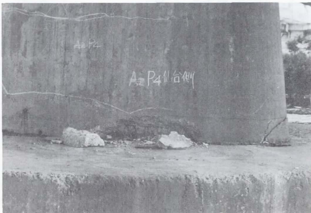
Figure 7.24 Sendai Ohashi Bridge. Typical damage to the base of a pier before repair.
