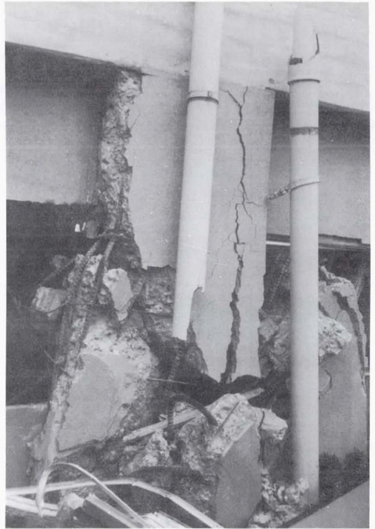
Figure 5.41 Yazaki Industries, showing damage to lower story reinforced concrete column.
