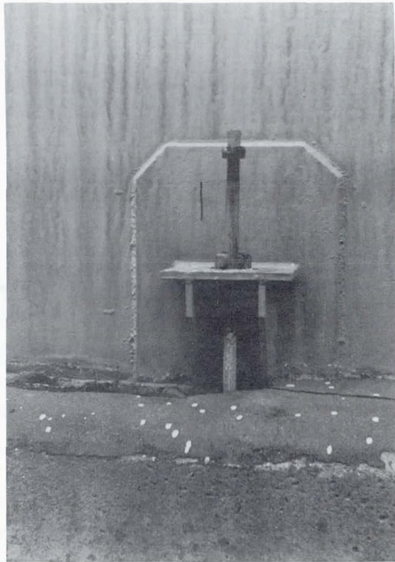
Figure 6.45 Sendai Refinery, Tohoku Oil Company, Ltd. A large water storage tank (left) near the main refinery complex appeared to have experienced significant rocking. Detail (right) of one of the pulled-out, or stretched, anchor bolts of the water storage tanks shown at left.
