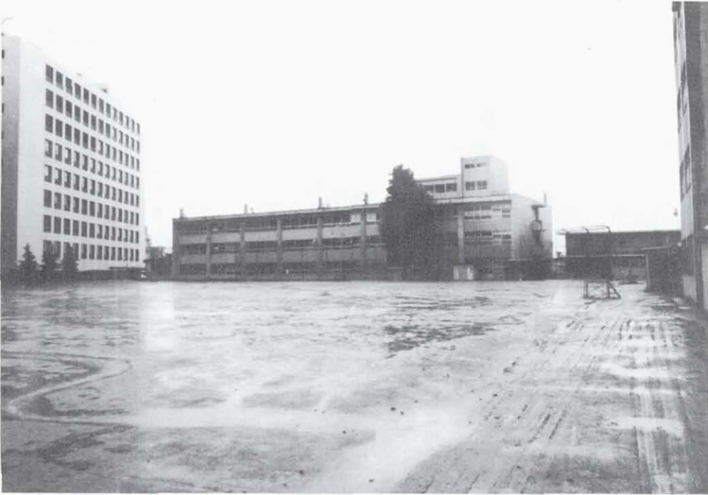
Figure 5.53 Tonan High School, west face. A small bluff on the opposite side of the building may have amplified ground motion. The adjacent structures were undamaged.
