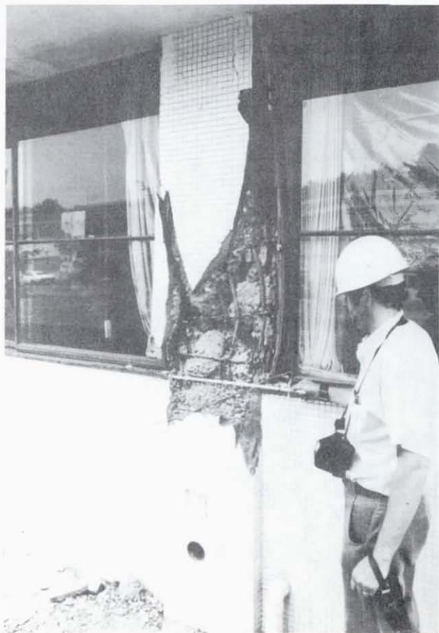
Figure 5.75 Tohoku Institute of Technology, Building 3. Damage to the ground floor columns on the south side of the building. Similar damage is present on the opposite side of the building.
