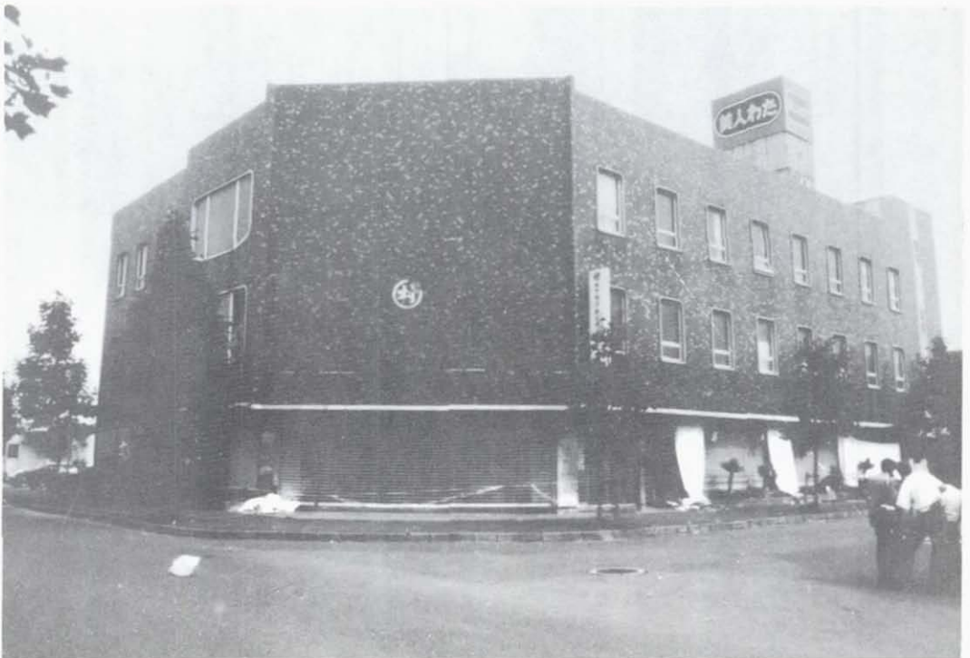
Figure 5.33 Kinoshita Building. The brick facing on the west side of the structure showed little sign of damage.
