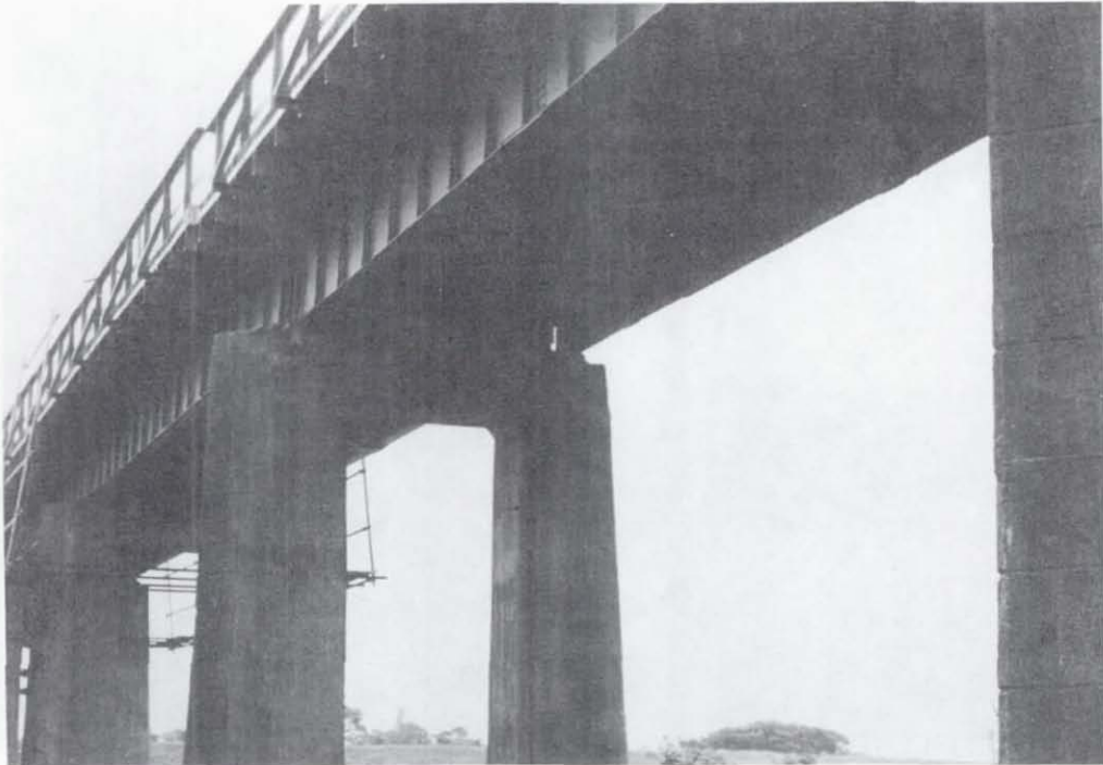
Figure 7.37 Spalled concrete at bent cap of Kimazuka Bridge.
