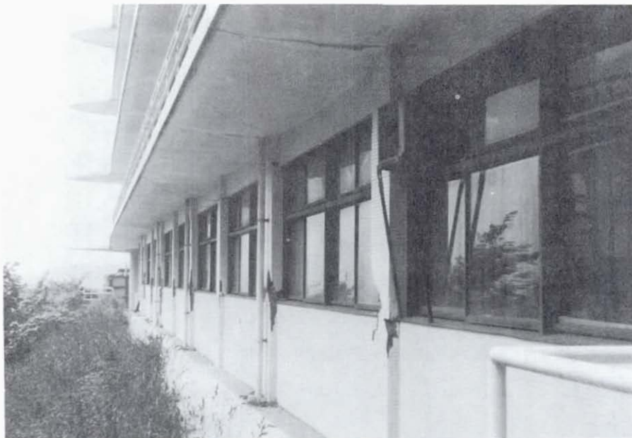
Figure 5.75 Tohoku Institute of Technology, Building 3. Damage to the ground floor columns on the south side of the building. Similar damage is present on the opposite side of the building.
