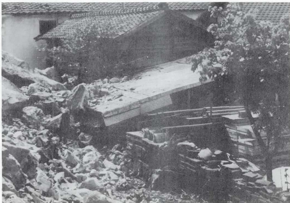
Figure 9.13 Rock fall from slope shown in figure 9.12 impinging on storage shed next to slope.
