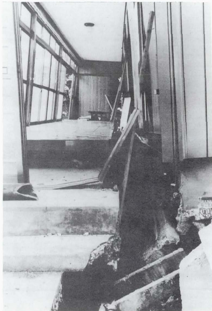
Figure 5.85 Sendai. Damage to single family residence due to ground settlement. (Japan National Land Agency photograph)
