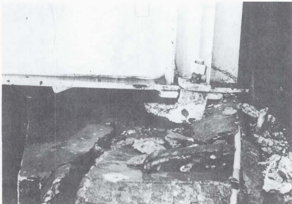
Figure 7.8 Kin-noh Bridge. Detail of bearing damage and abutment ledge failure, from February earthquake. Note extension of anchor bolt caused by 20 cm displacement of span towards abutment.
