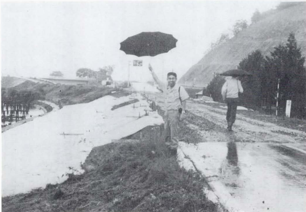
Figure 7.36 Road damage and temporary stabilization of the Kitakami Dike near the bridge site.
