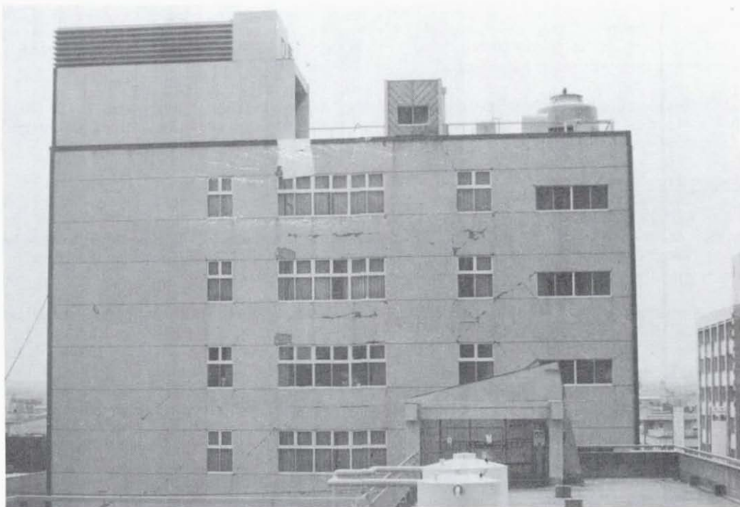
Figure 5.34 Maruhon Building, Oroshicho area, showing shear cracking in the panels on the east face between window openings.
