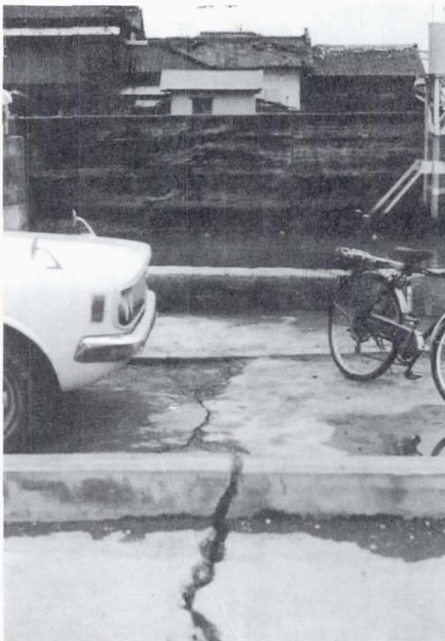
Figure 8.8 Site 2, Natori River. View is west across tributary of Natori River. Dike section shown in Figs. 8.6 and 8.7 is to right of houses in background of this figure. Note crack in concrete pavement in foreground is aligned with crack in retaining wall in background.
