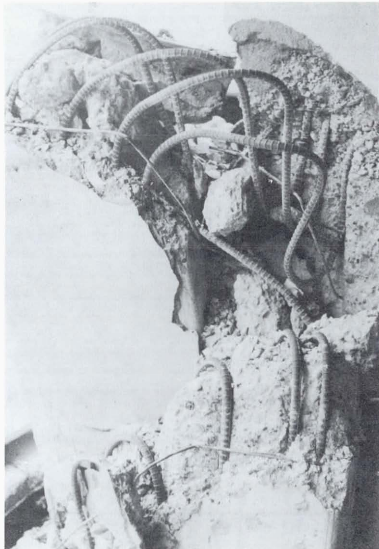
Figure 5.43 Yazaki Industries Buildings. Detail of column shear failure, east side. Note use of deformed bars.
