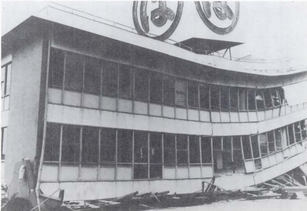
Figure 5.51 Taiyo Fisheries Plant, viewed from the west. The first story columns in the center portion of the building failed, leaving the ends of the building standing. (Japan National Land Agency photograph)
