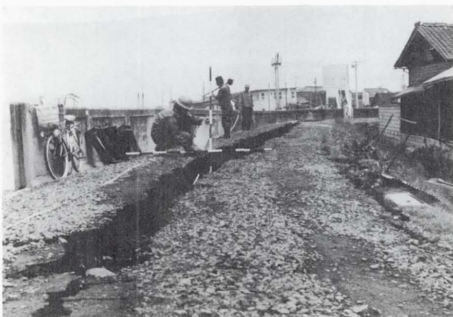
Figure 8.7 Site 2, Natori River. Settlement, lateral spreading, and longitudinal cracking of dike. View is east. (Photo courtesy Tohoku Regional Construction Bureau)
