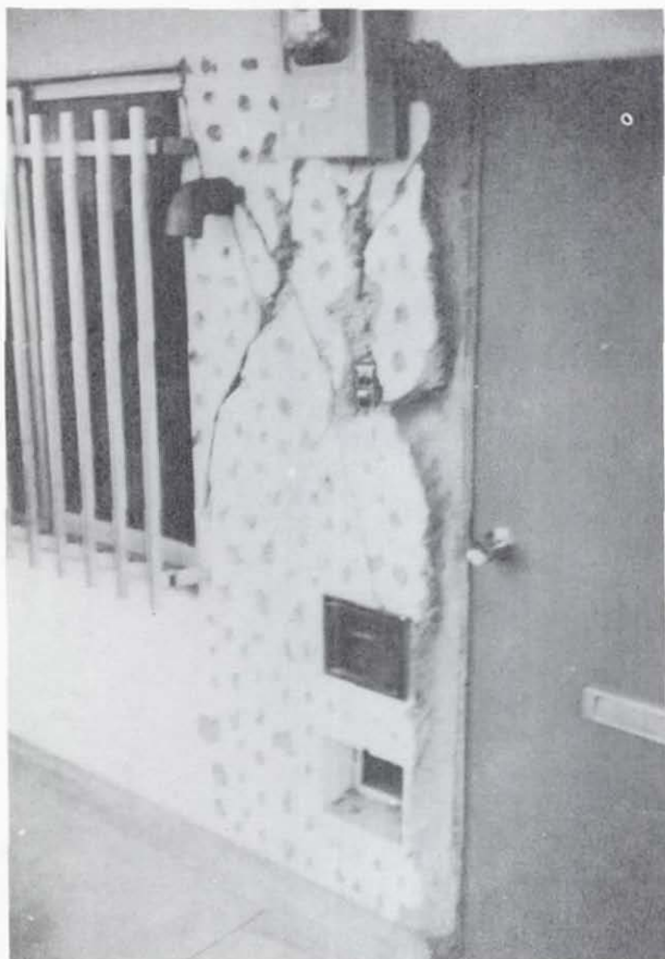
Figure 5.82 Sunny Heights Apartment Building. Detail of cracking of panels adjacent to doorways. Such cracking was typical at all levels on the east facade of the structure.
