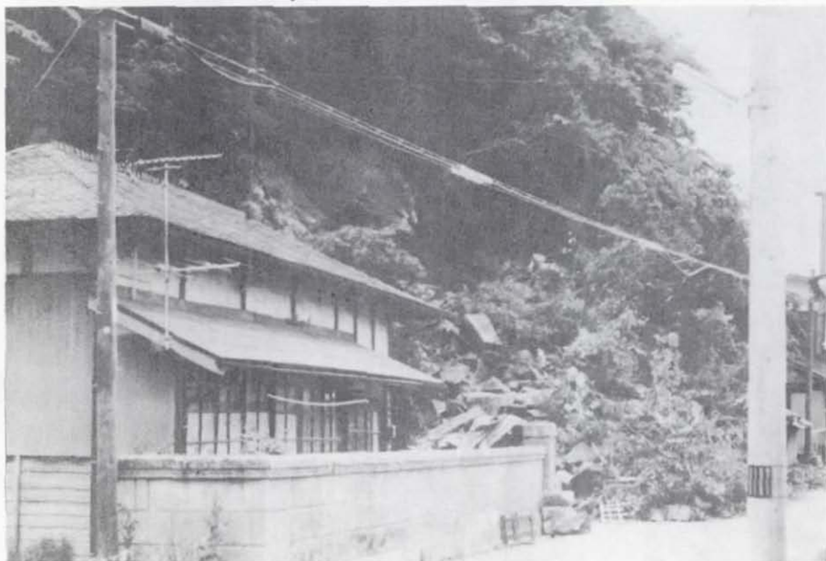
Figure 9.9 Rock fall in Miocene tuff causing damage to concrete wall adjacent to house. (Photograph courtesy of Y. Tsuruya)
