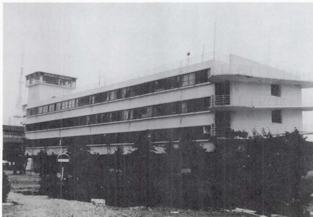
Figure 5.74 Tohoku Institute of Technology, Building 3. General view of the north elevation.
