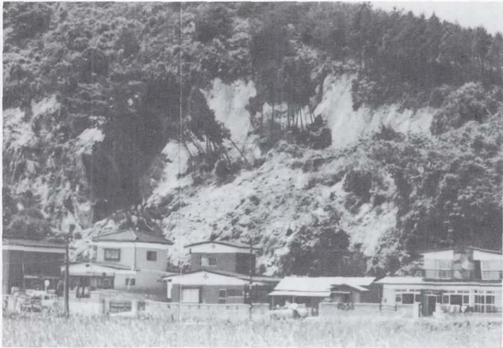
Figure 9.2 Rock fall on steep slopes of Miocene pumiceous tuff breccia near Takayamasuita. This rock fall damaged four houses close to the base of the slope. (Photograph courtesy of Y. Tsuruya, Slope Protection Division, Ministry of Construction).
