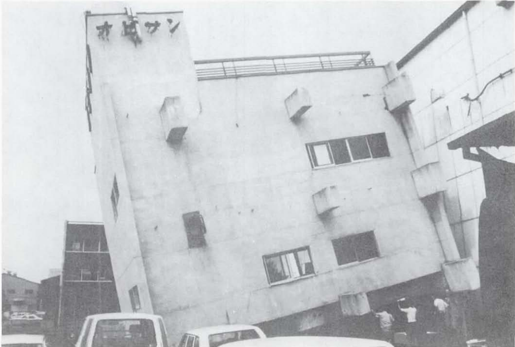
Figure 5.28 Obisan Building, viewed from the south. The upper stories rotated as a rigid body when the first floor column support was lost.
