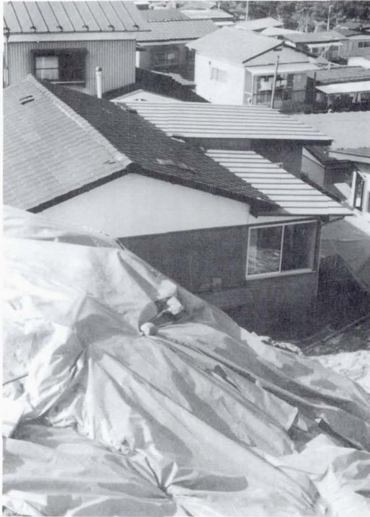
Figure 9.19 Toe of slump and house below in danger of being overridden by slide mass. House has been evacuated.
