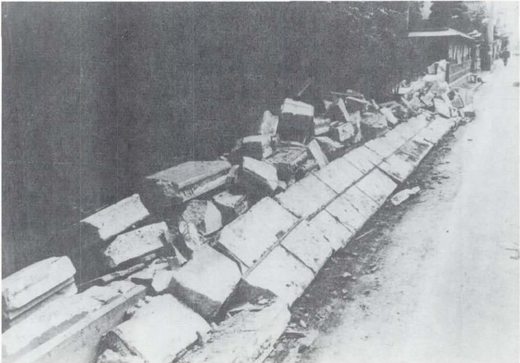
Figure 5.87 Failure of unreinforced concrete masonry wall in Sendai (Japan National Land Agency photograph)
