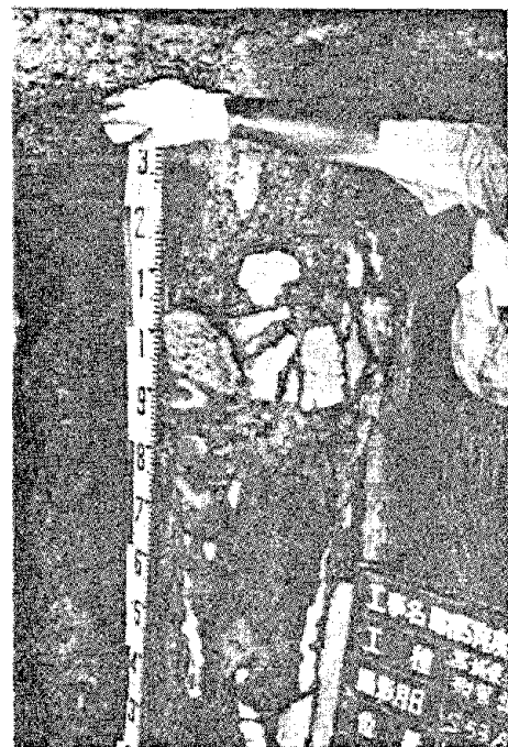
Fig. 4a) Damage of Pile (Case 3)
