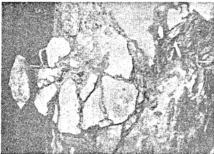
Fig. 4b) Damage of Pile (Case 3)
