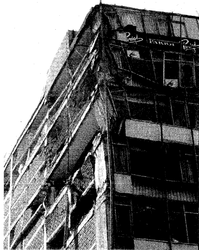
(b) Neighboring nine story building showing impact damage to columns.
