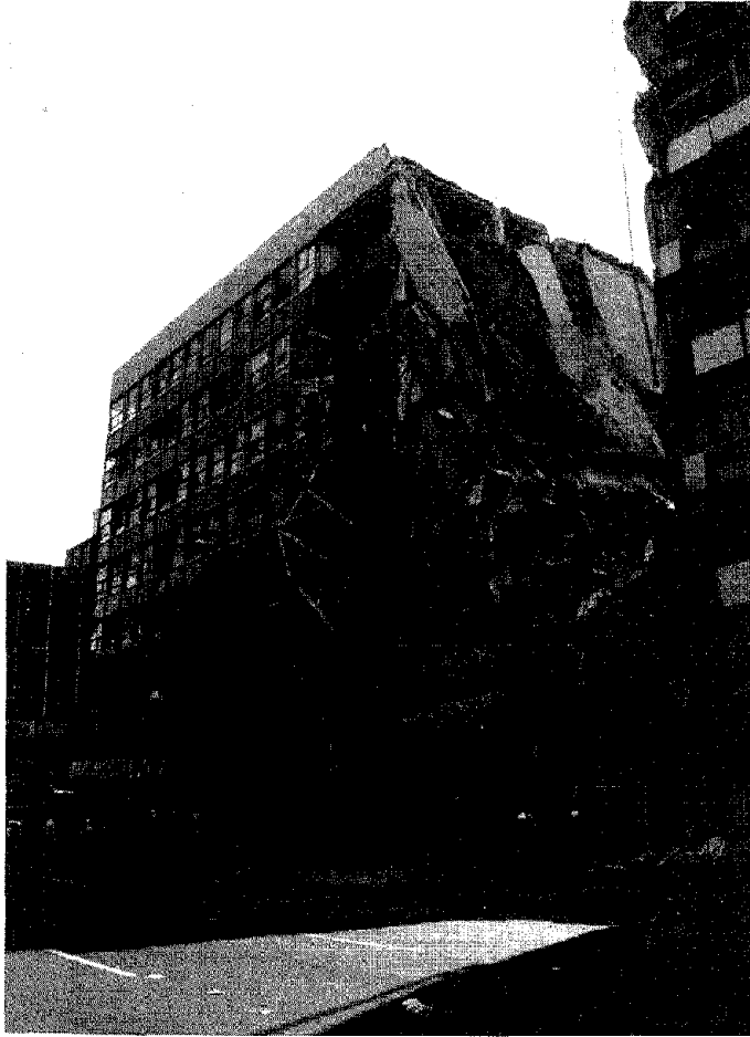
(a) Seven story office building on Ave. 20th de Novembre which collapsed due to pounding.
