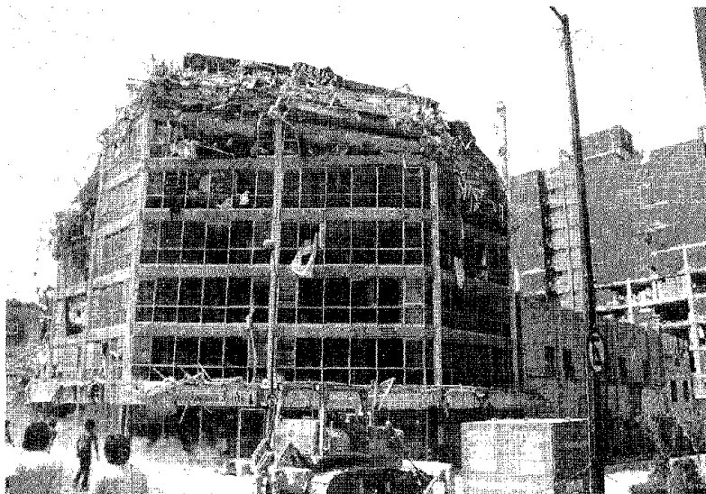
(b) Upper story failure in clothing store.
