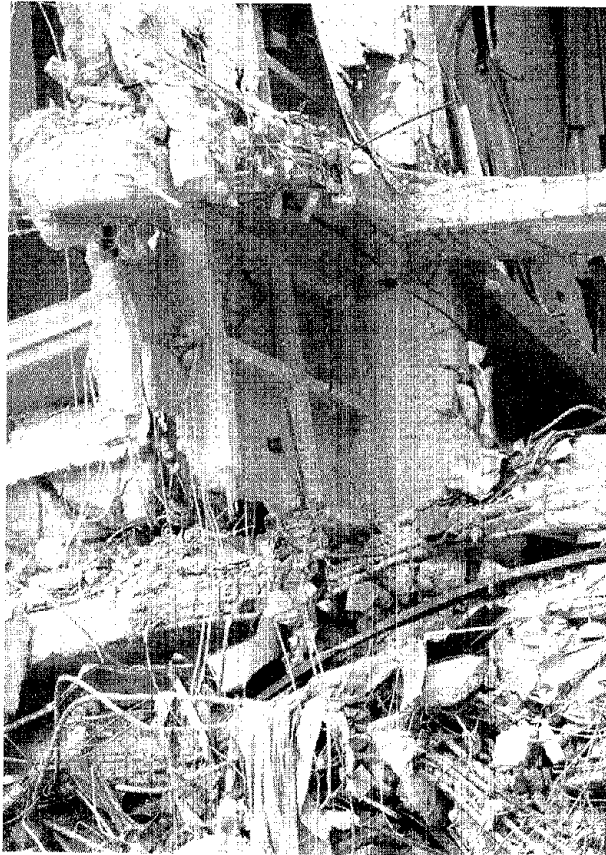
Figure 5.39. Collapsed 10 story apartment building in the corner of Dinamarca and Chapultepec. This waffle slab structure failure is attributed to base column failure and possible pounding with the neighboring structure.
