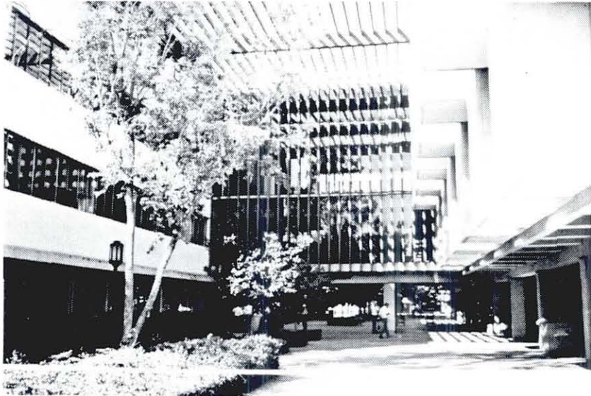
Photo 18 The library building complex on the campus of the California State University in Los Angeles. The two buildings are connected by a structurally-separated walkway structure.
