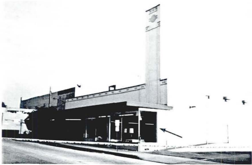
Photo 35 This remodeled masonry building experienced considerable damage to windows. Because large pieces of broken glass were strewn on the sidewalk, the building was cordoned off.
