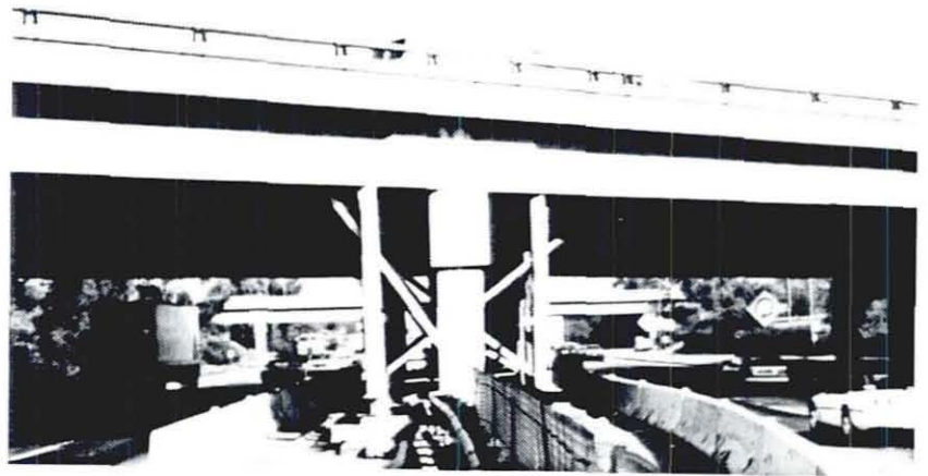
Photo 44 Shoring scheme used to temporarily support precast concrete girders.
