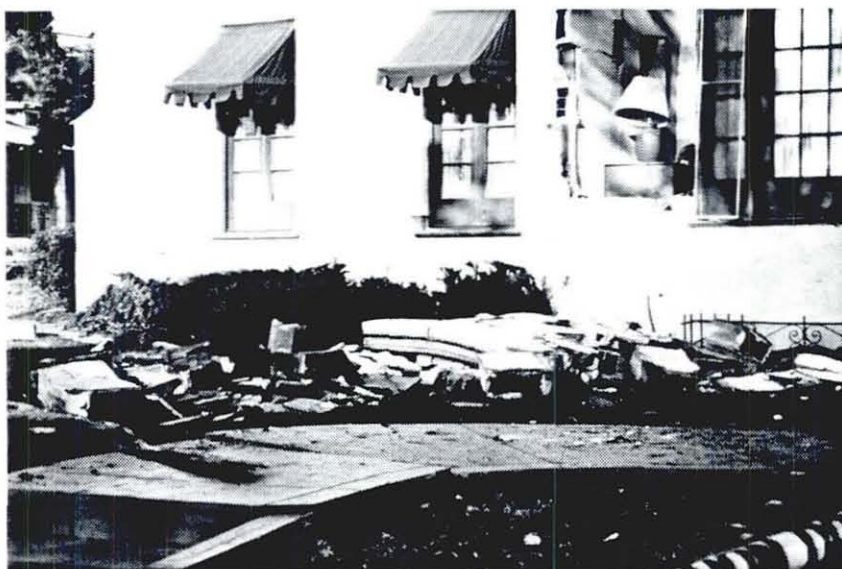
Photo 8 Large pieces of clay tile fell on the front yard of the house shown in Photo 7.
