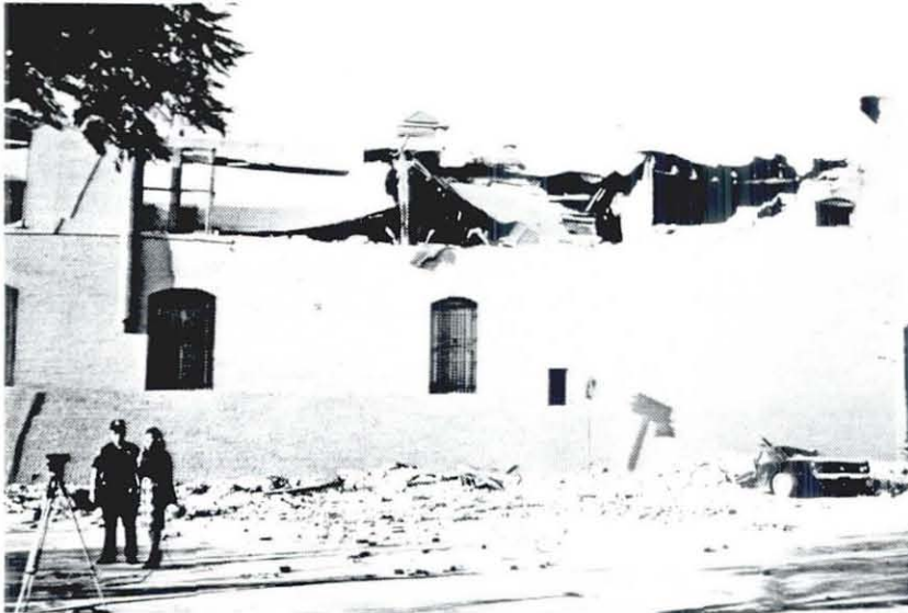
Photo 2 Collapsed unreinforced brick parapet and wall of a building in Uptown, Whittier. Falling bricks crushed cars parked adjacent to the building.
