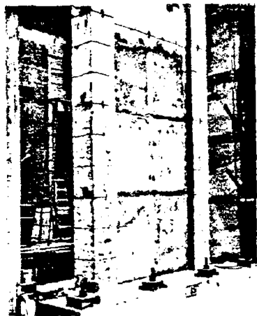
Figure 2.34 Specimen B5R after repair.
