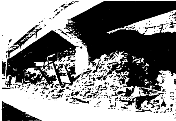
Photo 10 Damage to the National Highway No. 128 in Katsuura City
