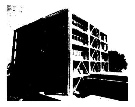
Figure 9 Building 113, after major seismic upgrade showing "K" brace frames.
