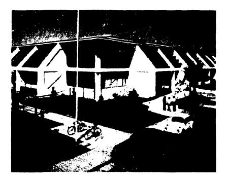
Figure 5 Building 311, after major seismic upgrade showing external buttresses.
