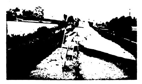
Figure 13. Cracking and slumping of lavee along the San Lorenzo River in downtown Santa Crus, resulting from liquefaction of foundation soils.
