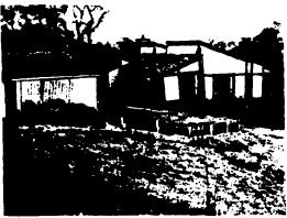
Figure 12. A badly damaged house in the Los Altos Hills area, supported on poles. The few connections between the poles and the floor framing failed due to poor quality welds. The floor joists were steel under the center portion of the house and wood at the edges. there appeared to be a lack of continuity between the two types of framing.
