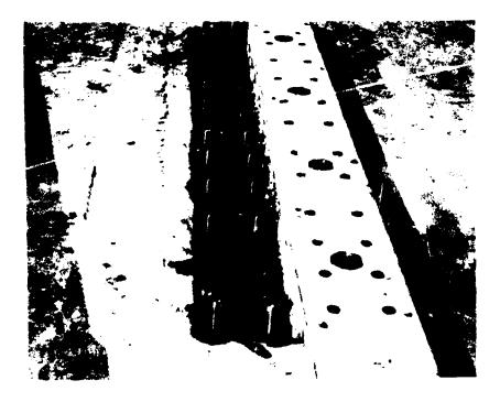
Figure 7 Building 311, Roof level drag-struct shear anchors.
