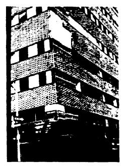
Fig. 5. Loss of Glass to Building, Oakland
