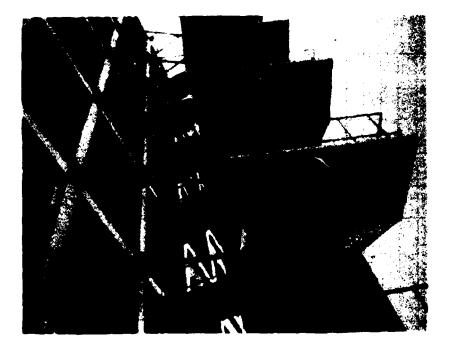
Figure 12 Building 111, stair tower upgrade, lateral supports are attached to each building floor level.
