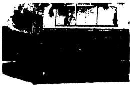
Figure 1. Two-story house with wood-framed daylight basement located about 100 feet from ground fissure in Santa Cruz Mountains. No apparent structural damage except collapsed masonry chimney.
