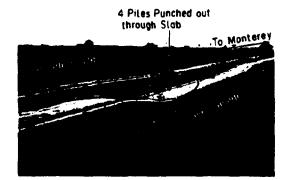
Photo. 9 Overall view of Struve Slough bridge, RC girder bridge with 21 spans and about 232m long, crossing over Struve Slough. There are 3 girder hinges along the longitudinal direction.
