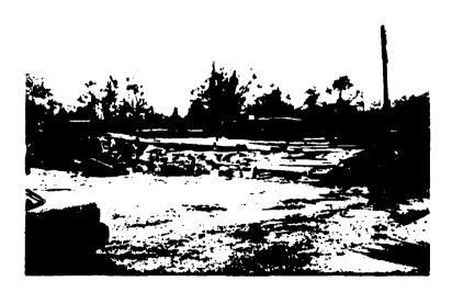
Figure 7. Collapse of Masonry Commercial Structure, North Charleston
