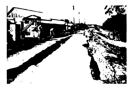
Figure 15. Liquefaction-induced fissures in levee of the Pajaro River, near Watsonville. The fissures were deeper than the height of the levee.
