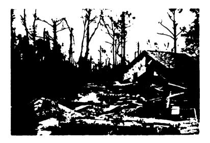
Figure 3. Shear Failure of House, Bull Bay.
