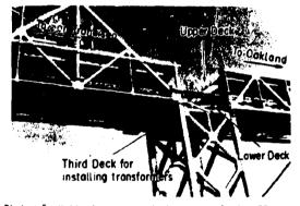
Photo. 5 Wall of one-span decks on steel pier E9. Upper and lower decks fell down, but fortunately those two decks stopped on the third deck which install transformers (from CALTRANS).
