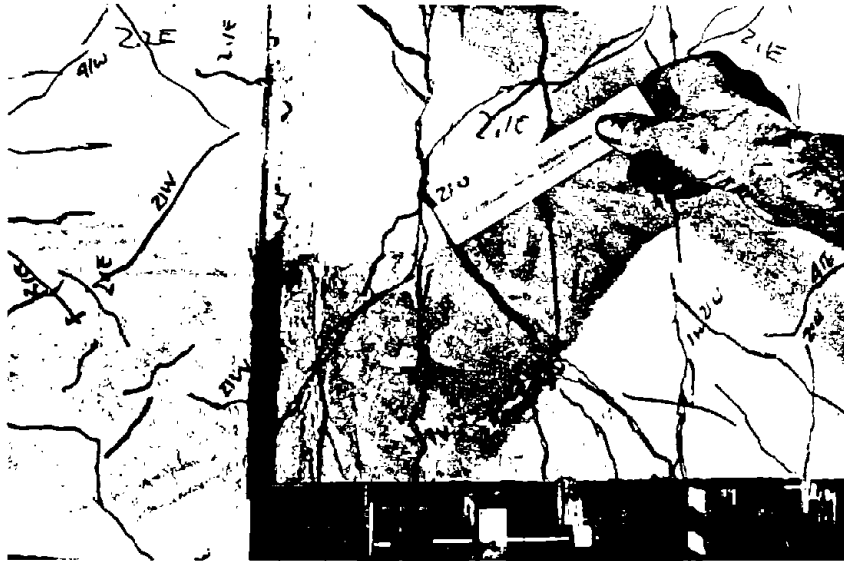
Fig. 4.21 Crack opening in beam of B-M-Z4 at 6 \Delta_y , cycle 1.
