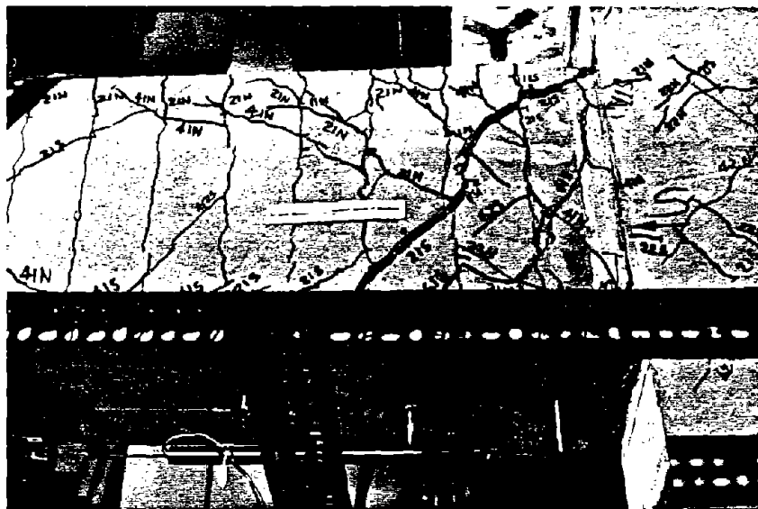
Fig. 4.24 Shear crack opening of A-M-24 at 6 \Delta_y , cycle 2.
