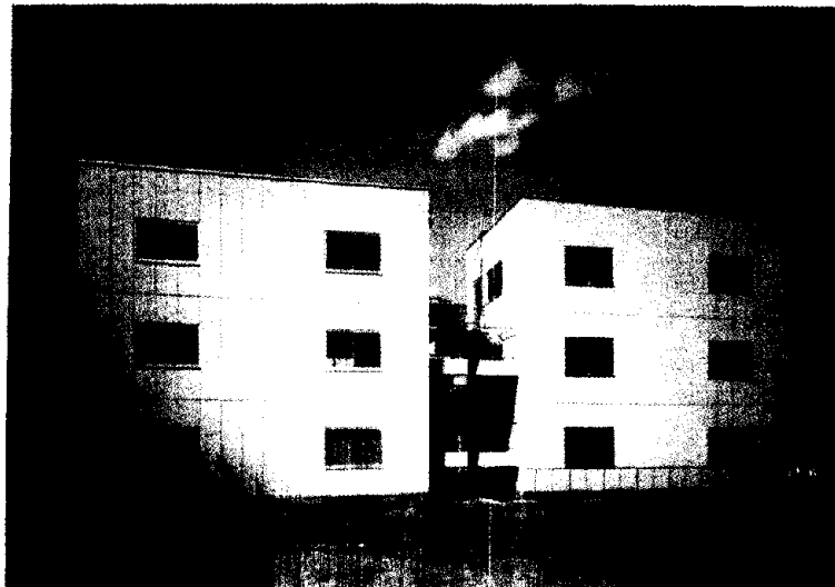
View of the experimental base isolation building. Left-Building with conventional structure Right-base isolation structure.
