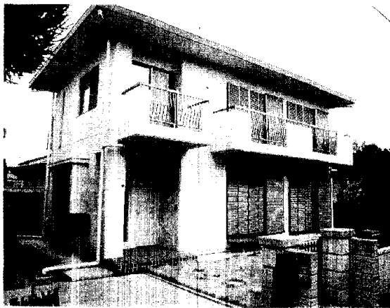
View of the Menshin apartments
