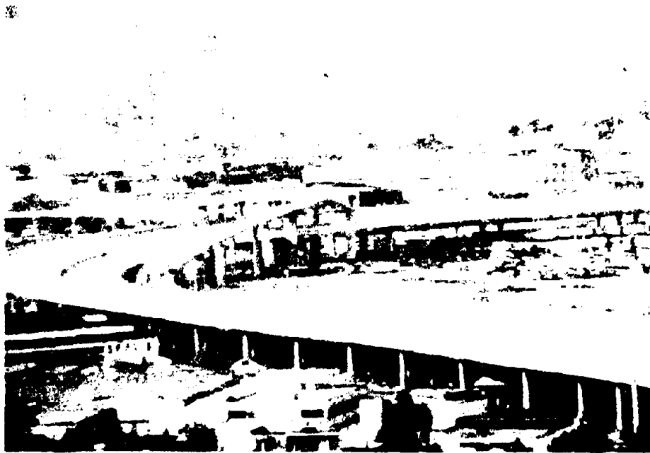
Figure 21. Aerial view of the Six Street exit ramp
