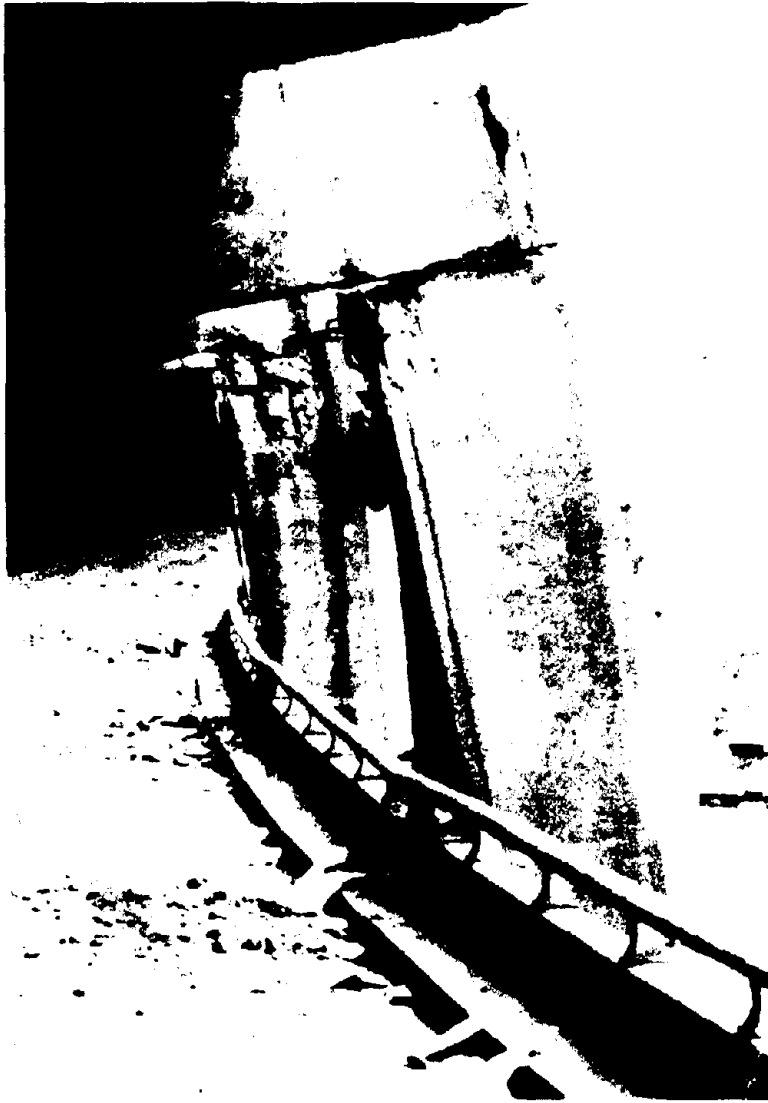
Figure 11 A close-up view of failure of Type 2 bents
