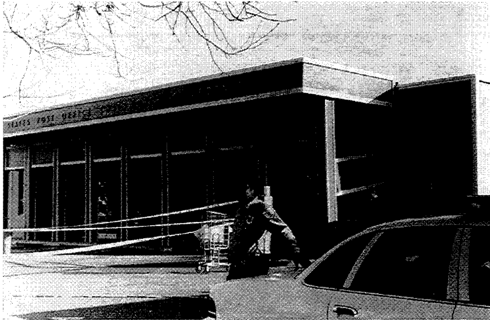
Figure 3.35 The Chatsworth Post Office was closed due to damage. Mail was being collected in the parking lot.
