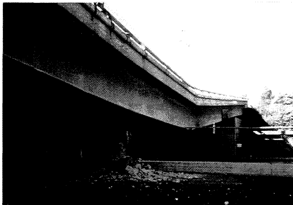
Figure 4.44 View of collapsed span of I10 over Fairfax Ave.; note rotation of girder over Pier 2 (Courtesy of EERC)
