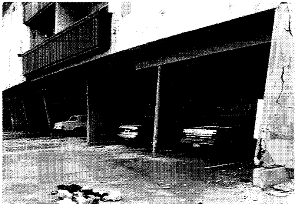
Figure 3.5 Steel pipe columns between parking bays supported the upper stories of the Northridge Meadows apartment buildings. Few of the buildings in the north half of the complex collapsed, but all were damaged.
