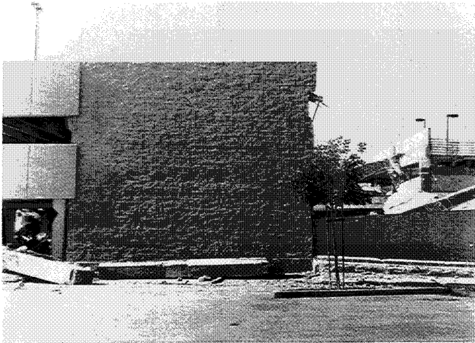
Figure 3.66 At the Northridge Fashion Center, major portions of the three-level south parking garage collapsed. The garage was precast concrete with intermittent shear walls. Most of the shear walls remained standing, largely undamaged, indicating that the lateral load was not adequately transmitted to these walls.
