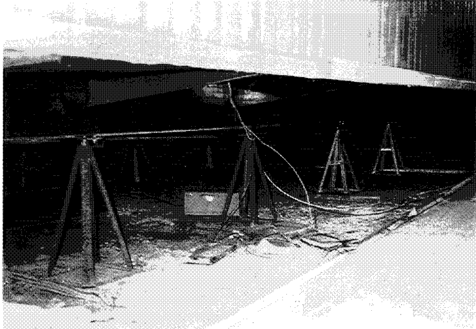
Figure 3.21 Another foundation system used for manufactured housing consists of supports constructed of small metal angles.
