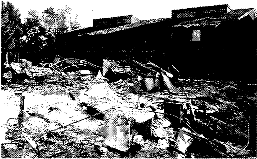
Figure 6.6 Multi-family residential building destroyed by fire.
