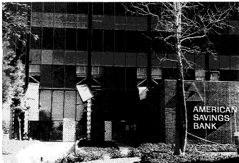
Figure 3.52 The first-story columns of the steel-framed building housing the American Savings Bank on Topanga Canyon Road in Canoga Park flexed during the quake and ended up slightly displaced from their original positions.
