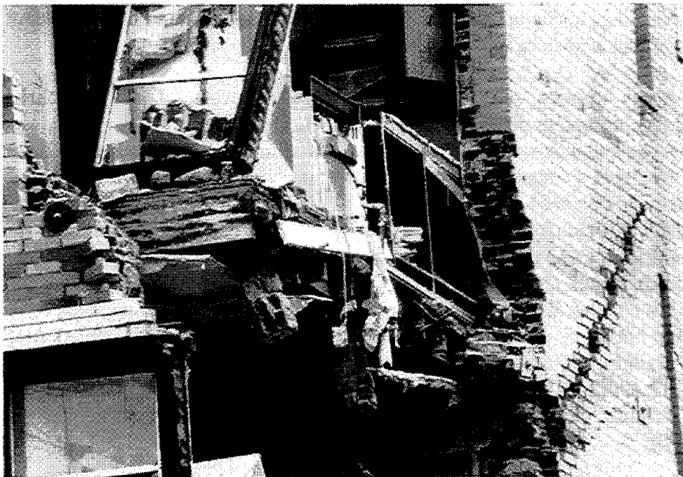
Figure 3.38 A close-up view of the third-story floor diaphragm of the building picture above shows (lower right) a rehabilitation bolt still holding a few bricks to the floor joists, after all the walls on three out of four sides of the bolts had disintegrated.
