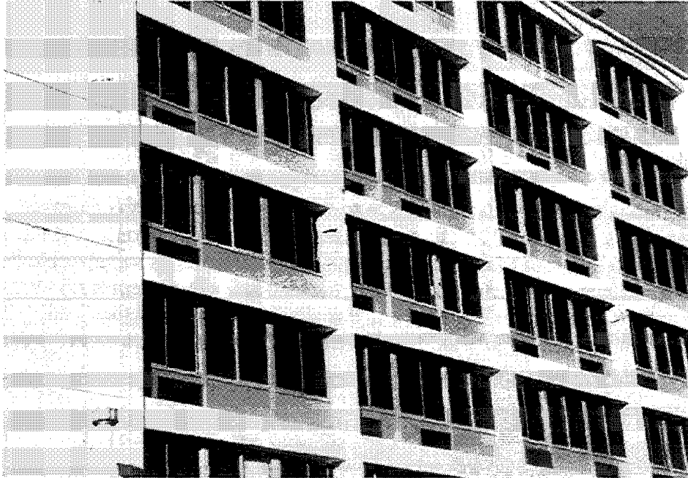
Figure 3.16 The bottom two stories of the concrete frame Holiday Inn in Van Nuys were damaged in the 1971 San Fernando quake and subsequently repaired. In the 1994 Northridge quake, damage was concentrated at the top of the fourth floor columns.
