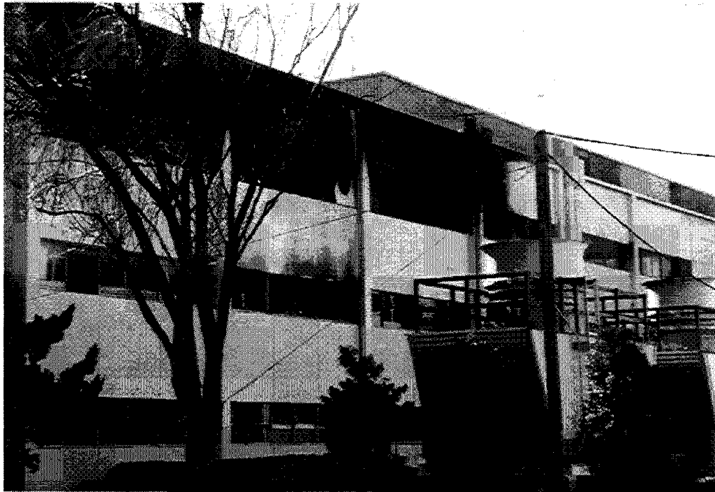
Figure 6.7 University science building damaged by fire.
