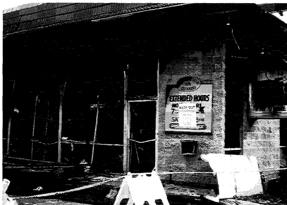
Figure 6.1 Fire damage in a single story commercial building.
