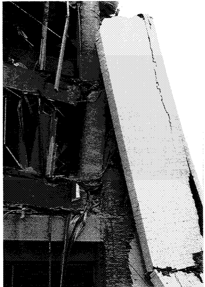
Figure 3.44 The exposed concrete frame of the Kaiser Permanente building, revealing deep beams, suggests that the building had a strong- beam, weak-column configuration. Except for the second story columns, the columns and beams remained intact while the joints disintegrated.
