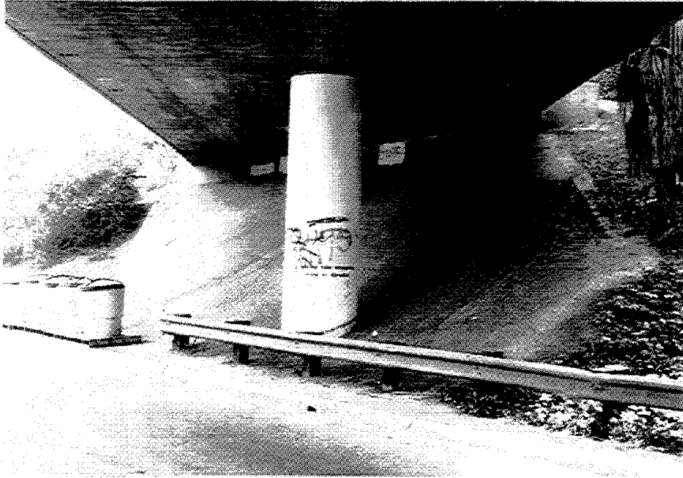
Figure 4.34 Cadillac Ave. ramp; view to east showing jacketed pier
