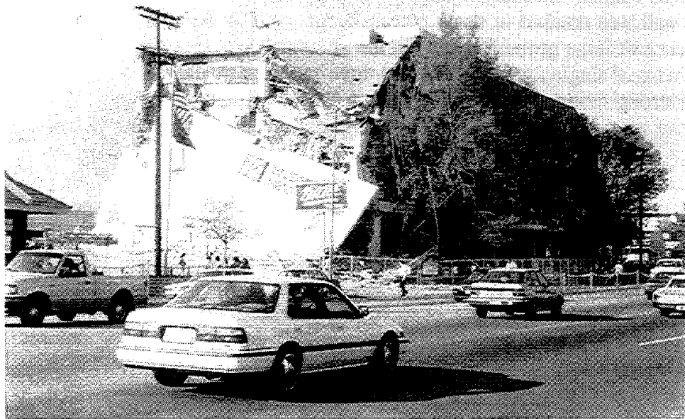
Figure 3.42 Both end walls of the Kaiser Permanente building slid, partially intact, to the ground. The south wall is pictured here. Both ends of the building suffered damage to the concrete frame at all story levels, while the middle half of the building, except for the second story, remained intact.
