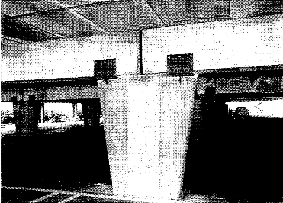
Figure 3.64 The interior columns of the two-level parking garage at the Trans World Bank in Sherman Oaks had been seismically strengthened after it suffered damage in the 1971 San Fernando quake. The interior columns fared well in the 1994 Northridge quake.
