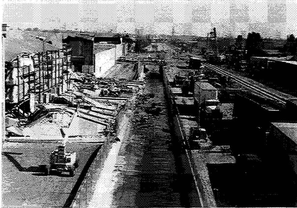
Figure 3.33 The south wall of the concrete tilt-up Levitz furniture store/warehouse south of the Northridge Fashion Center fell away from the building into the alley and stream channel. The damaged roof was being supported by the racks of furniture. On the south side of the stream channel a freight train derailed during the earthquake. That clean-up effort was still underway three days after the quake.
