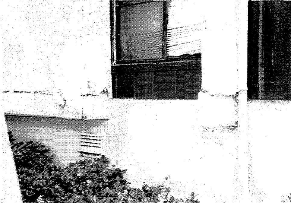
Figure 3.8 Horizontal cracks at the interface of the foundation wall (usually concrete) and the first story (typically wood-framed with stucco facade) were often seen in damaged low-rise apartment buildings.
