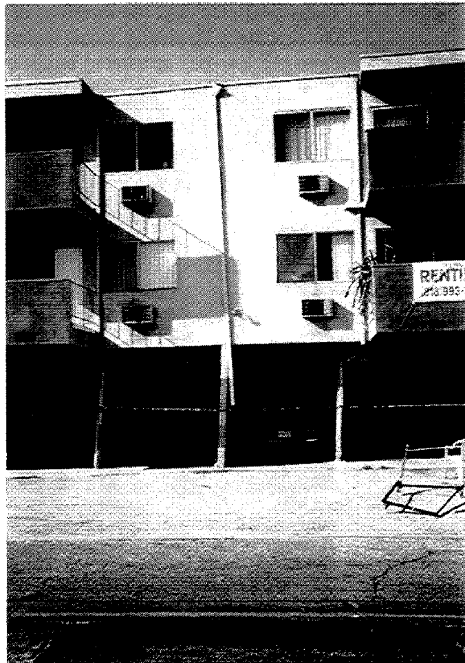
Figure 3.7 Racking, or leaning, of open first story parking areas was a common feature of damaged two and three-story apartment buildings.
