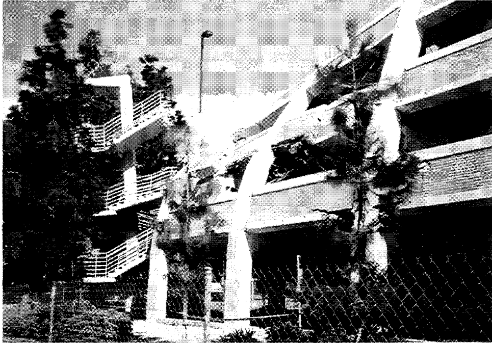
Figure 3.60 The three-year old four-level parking garage at the Northridge campus of California State University partially collapsed in the earthquake. The collapse apparently started at the interior, causing the exterior walls to be pulled in to the middle of the structure. Precast concrete "trees" were connected to form a moment-resisting frame at the exterior of the structure.
