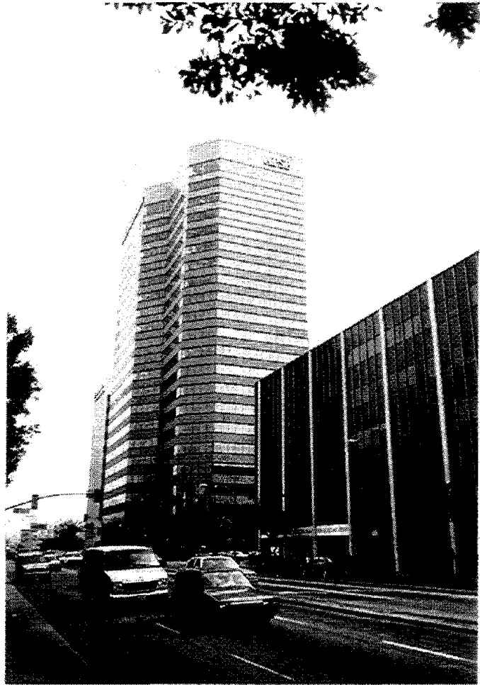
Figure 3.57 There was no evidence of damage to the twenty-two story American Pacific State Bank in Sherman Oaks. The adjacent eight-story parking garage had damaged columns.
