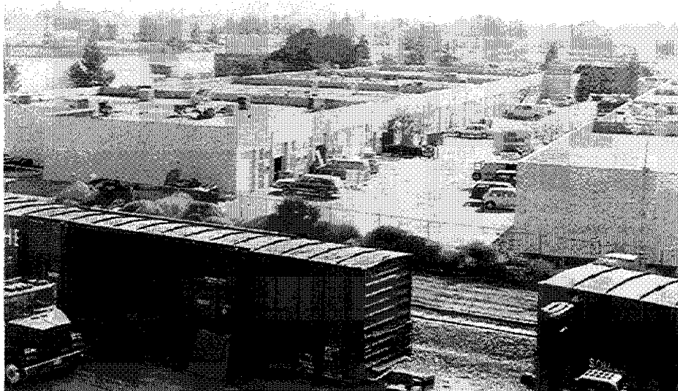
Figure 3.34 The single-story modern masonry commercial buildings directly south of the damaged Levitz furniture store and train derailment were apparently undamaged. All parapets and piers between garage openings appeared intact.
