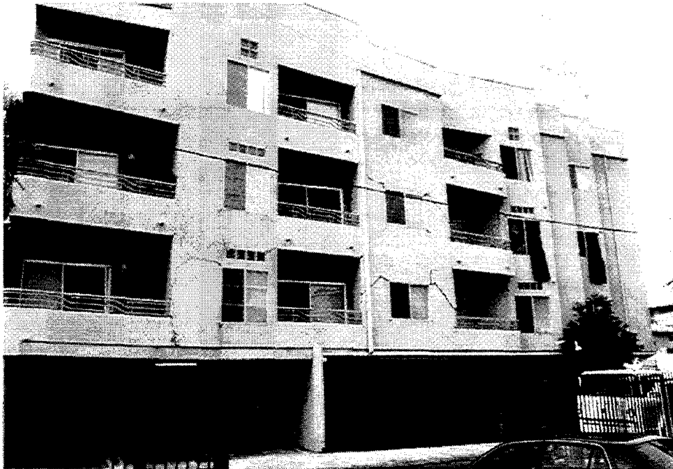
Figure 3.9 Typical damage in to low-rise apartment buildings included diagonal cracks in the stucco facade at the corners of windows and other openings.
