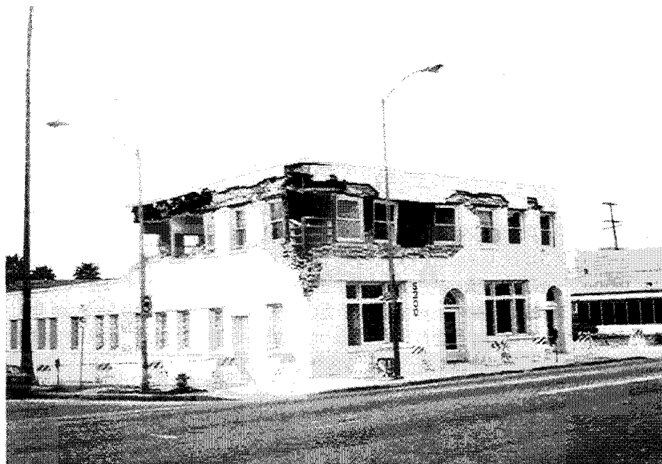
Figure 3.40 In other rehabilitated unreinforced masonry buildings, such as this two story structure in Hollywood, entire wall thicknesses were lost between rows of through-bolts.
