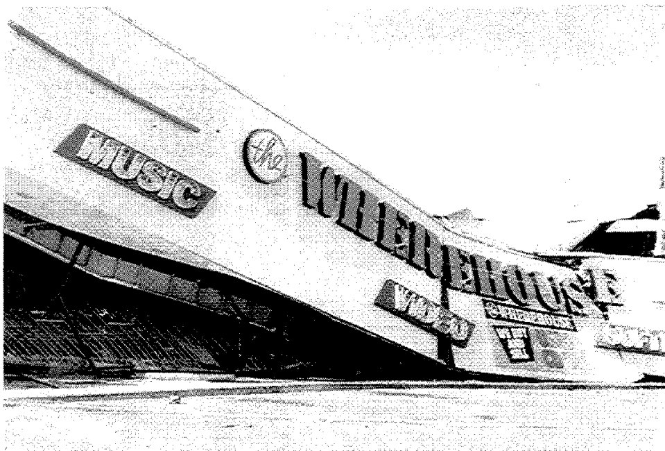
Figure 3.32 Many commercial buildings were damaged in the blocks south of the Northridge Fashion Center. The single-story Warehouse collapsed completely.
