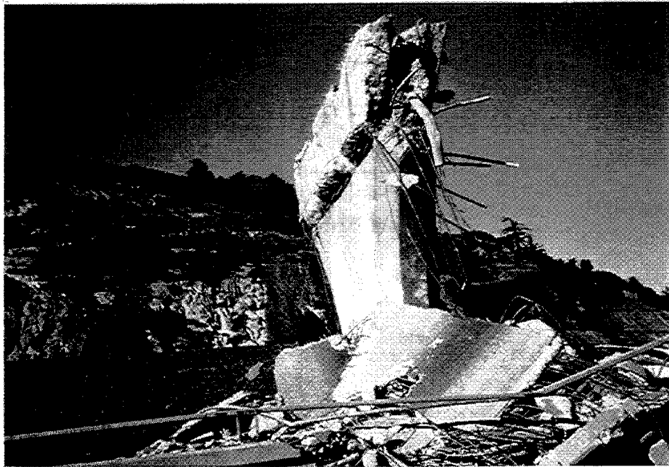
Figure 4.12 Damage at Pier 3 of the SR14/I5 Separation and Overhead, Ramp C, looking to the west (Courtesy of EERC)
