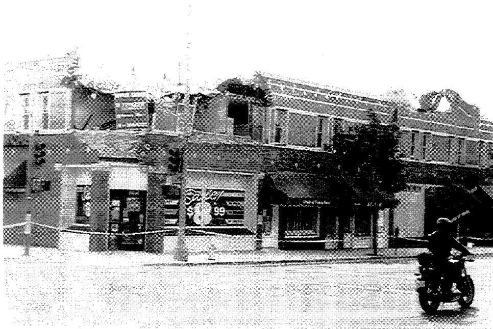
Figure 3.36 Damage to unreinforced masonry buildings, even those that had been rehabilitated, was common. Upper stories and corners were particularly vulnerable to damage. The rows of light-colored diamonds on the face of this building are the end plates of through-bolts used to connect the wall to the floor joists, a typical rehabilitation technique. The remains of parapet braces can be seen on the roof.
