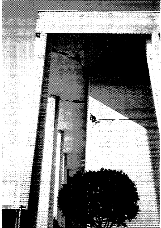
Figure 3.31 The Broadway department store at the Northridge Fashion Center had horizontal cracks in the facade and spalled corners at each floor level, and cracks in the soffit.
