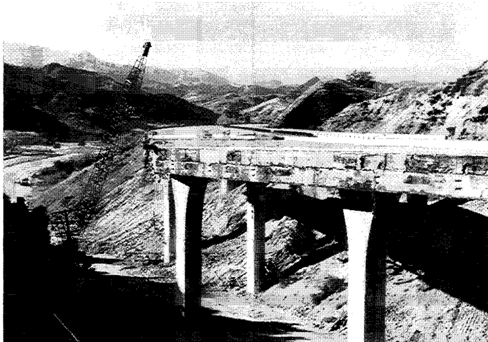
Figure 4.3: Ground level view of the southbound bridge at Gavin Canyon, looking to the northwest, showing the hinge bearing seat near Bent 3.
