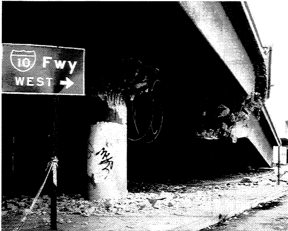
Figure 4.38 Collapsed westbound lane of I10 at Venice Blvd.; pier of Bent 7 in foreground
