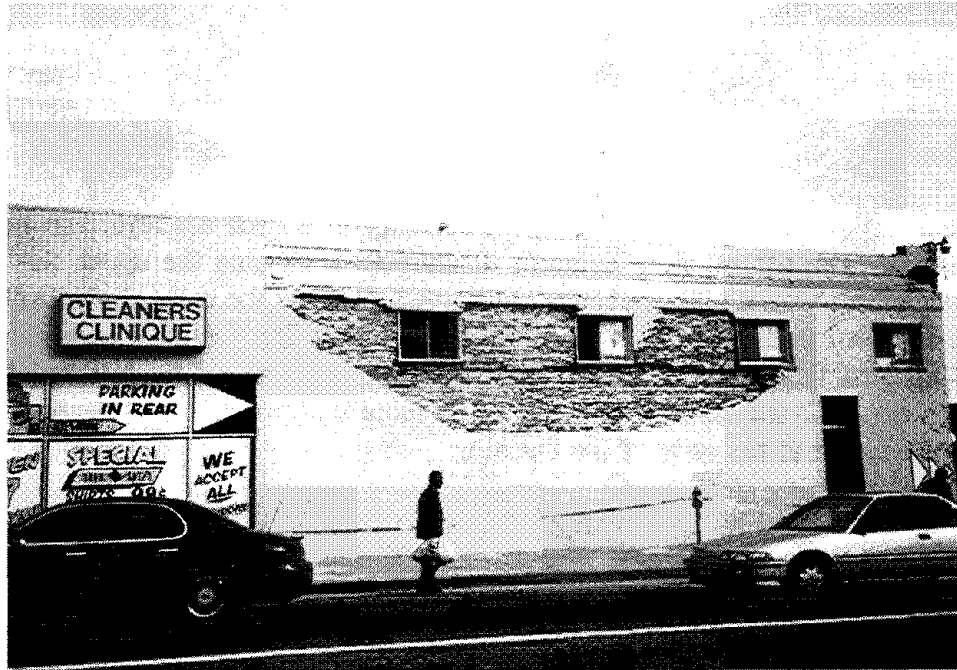
Figure 3.39 Only the exterior wythe of brick peeled off of this rehabilitated unreinforced masonry building in Santa Monica.
