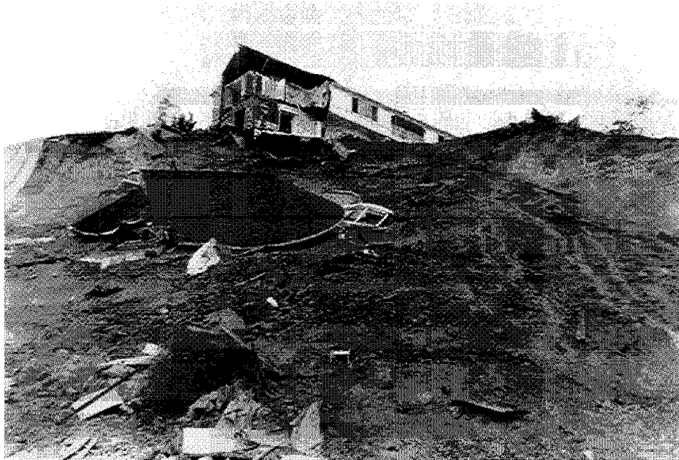
Figure 2.8 A landslide along the Pacific Coast Highway north of Santa Monica undermined the foundation of a house at the crest of the slope, bringing a portion of the house down.
