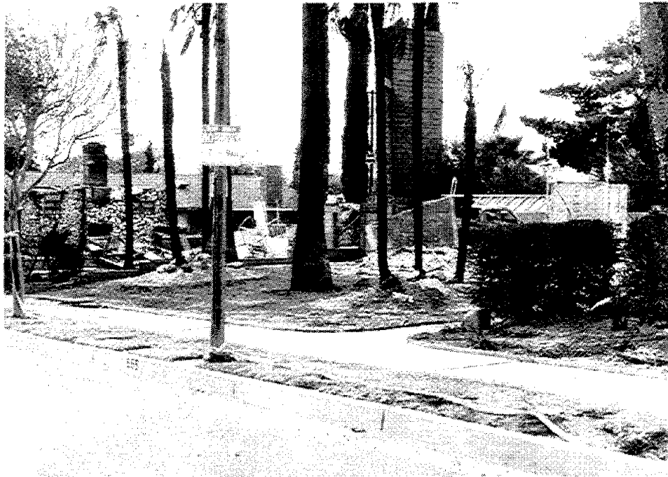
Figure 5.13 Houses destroyed by a fire resulting from the rupture of the 0.6-m gas main along Balboa Boulevard.
