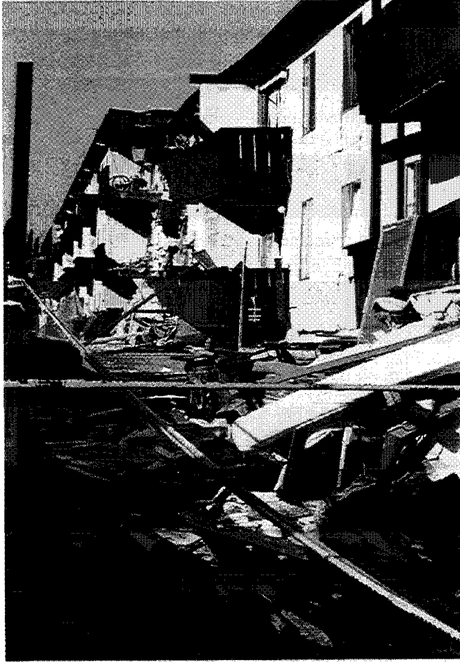
Figure 3.4 At the Northridge Meadows apartment complex near the epicenter the first story in several of the buildings collapsed, killing sixteen people. The second and third stories remained essentially intact. Large portions of the first story in these buildings were open space for parking. This type of collapse occurred in a significant number of similar apartment buildings throughout the affected area.
