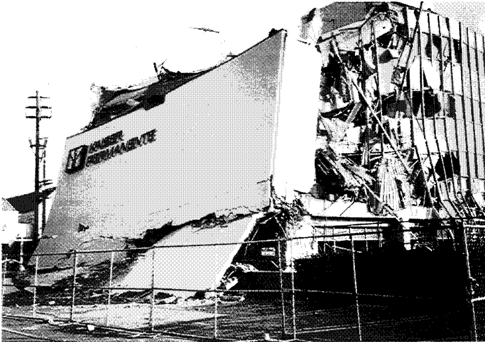
Figure 3.43 Damage at the north end of the building was similar to damage at the south.
