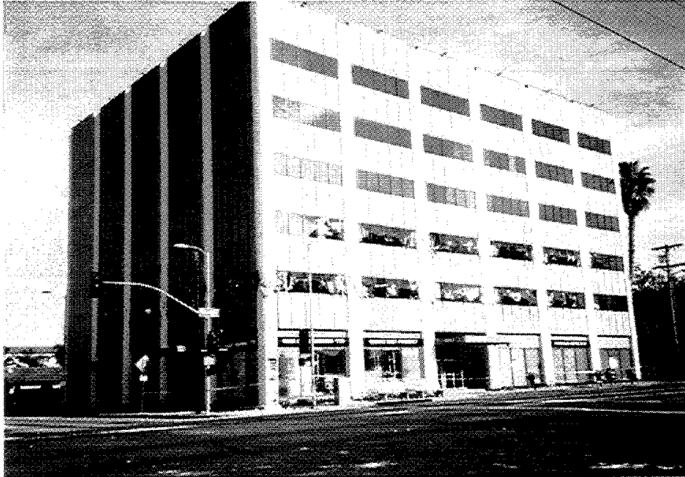
Figure 3.45 The six-story L-shaped concrete-frame Barrington Building on Olympic Boulevard in West Los Angeles lost its vertical-load carrying capacity at the second story.
