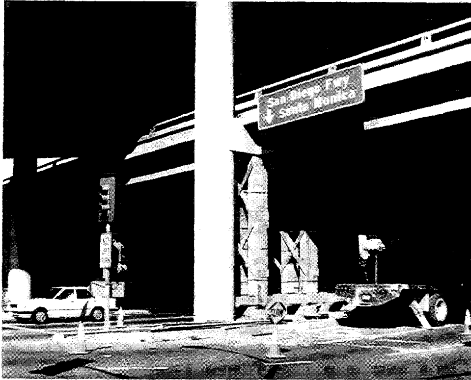
Figure 4.53 Overview of the outrigger joint at the SR90/I405 interchange, Jefferson Boulevard Undercrossing, center bent, west side, looking to the north
