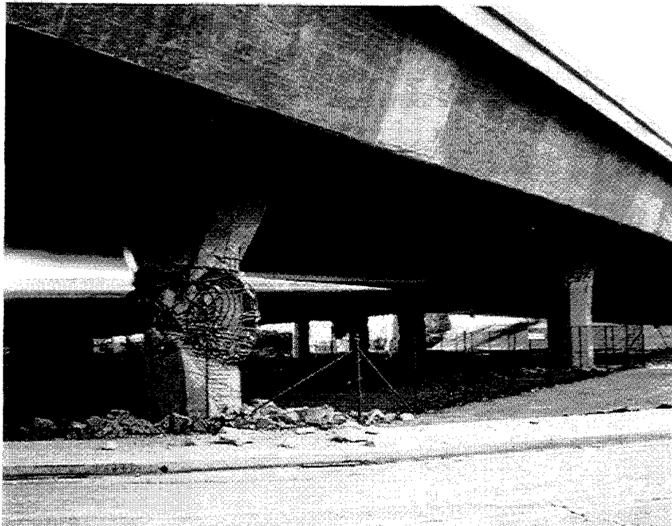
Figure 4.20 Damage to piers of the SR118 Mission-Gothic Undercrossing, looking to the northwest at the north face of the westbound bridge, Bents 3 (foreground) and 2.
