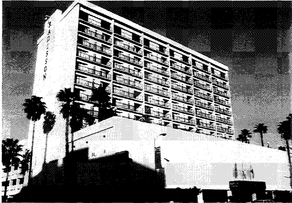
Figure 3.55 The concrete Radisson Valley Center Hotel in Sherman Oaks had serious damage to the columns at the first and fifth stories.
