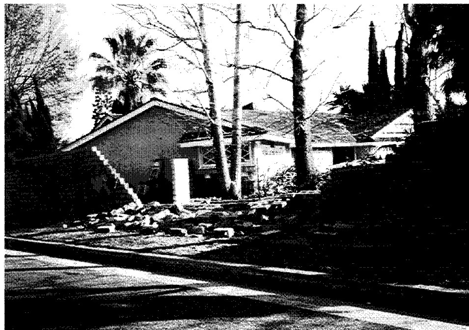
Figure 3.18 Damage to masonry privacy fences was ubiquitous. Many of these fences were tall enough to have been a serious threat to passersby when they failed. Luckily, due to the early morning hour of the quake, yards and sidewalks were essentially deserted.
