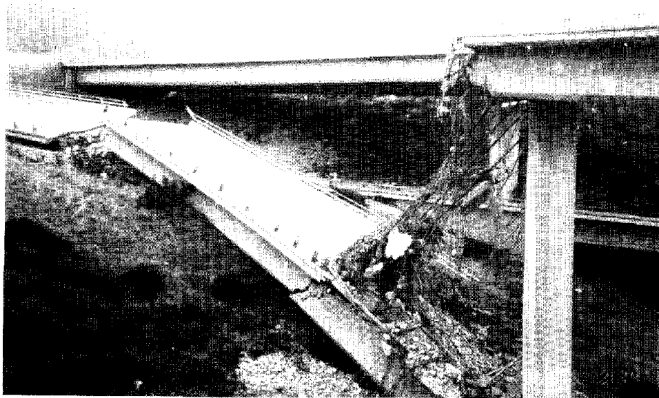
Figure 4.14. Collapsed portion of the SR14/15 North Connector Overcrossing, looking east. Pier 2 was at the left, near the broken hinge on the ground (Photo courtesy of EERC).
