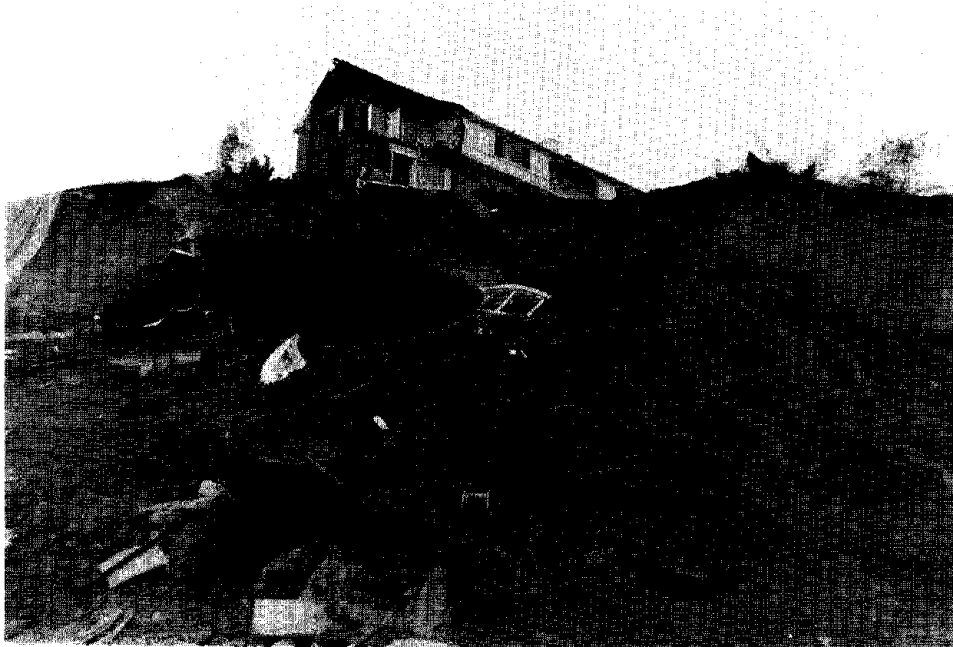
Figure 2.8. A landslide along the Pacific Coast Highway north of Santa Monica undermined the foundation of a house at the crest of the slope, bringing a portion of the house down.
