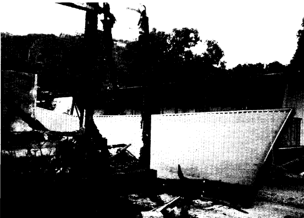
Figure 6.10. Collapsed roof which acted as a fire break in a manufactured housing development.
