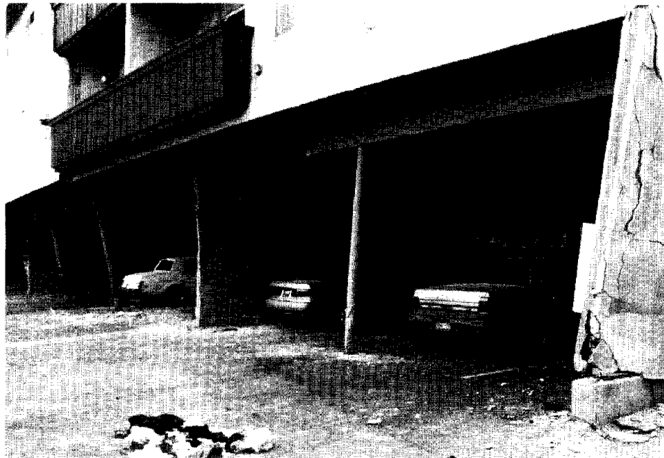
Figure 3.5. Steel pipe columns between parking bays supported the upper stories of the Northridge Meadows apartment buildings. Few of the buildings in the north half of the complex collapsed, but all were damaged.
