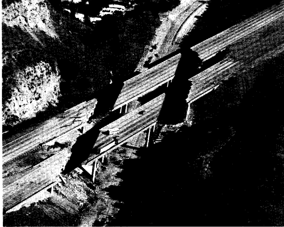
Figure 4.2. Aerial view of the bridges at Gavin Canyon, looking to the east, showing appearance of the four end spans shortly after demolition had begun.
