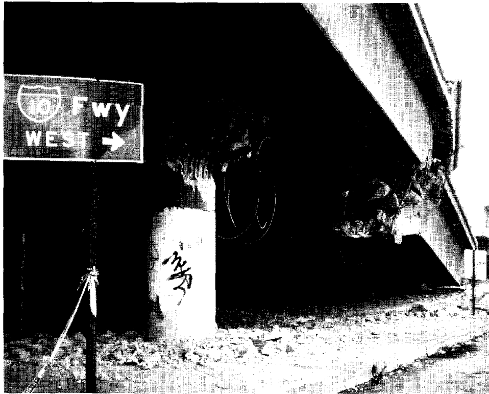
Figure 4.38. Collapsed westbound lane of I10 at Venice Blvd.; pier of Bent 7 in foreground.
