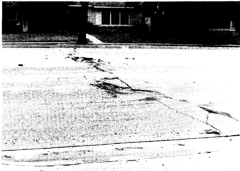
Figure 5.19. Transverse cracks in pavement along Balboa Boulevard in Northridge area.
