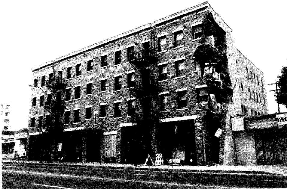
Figure 3.37. The corner of this rehabilitated unreinforced masonry apartment building in East Hollywood crumbled on all four stories.
