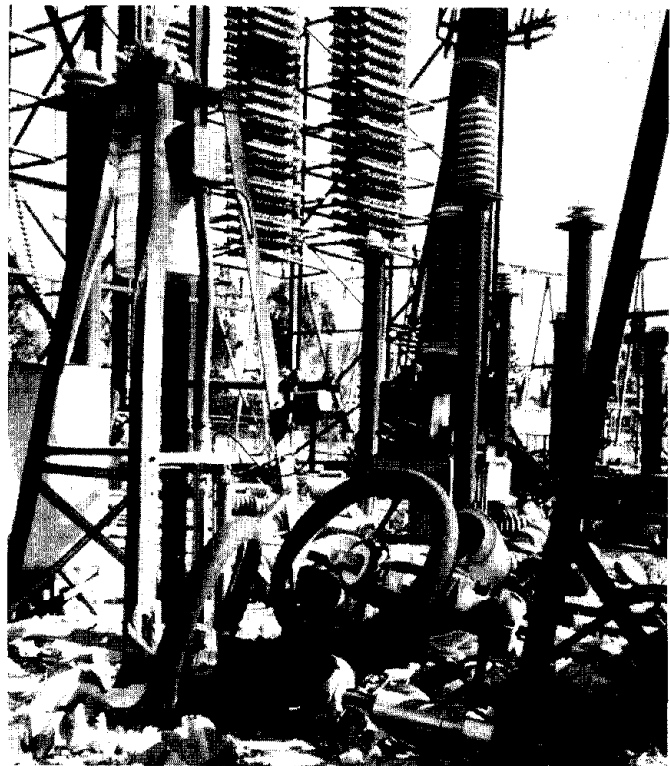
Figure 5.16. Porcelain is an integral part of high voltage electrical equipment due to insulation requirements and is also the most vulnerable to damage during strong earthquake shaking. (Photo courtesy of Edward Matsuda, Pacific Gas and Electric Company.)
