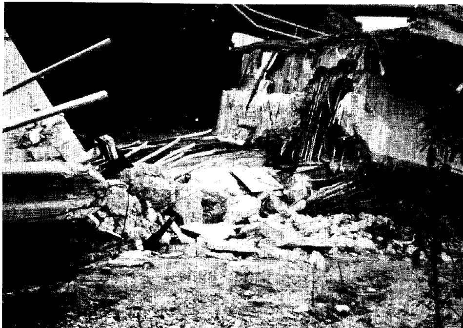
Figure 4.16. View of crushed Pier 2 and the hinge near Pier 2 (Photo courtesy EERC).
