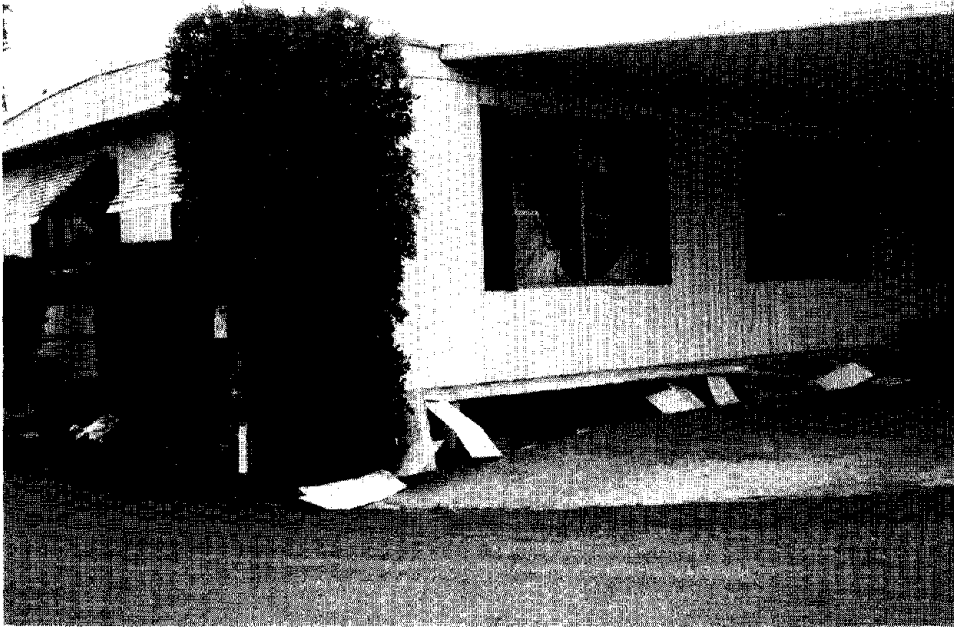
Figure 3.19. Damage to manufactured homes caused by collapsed supports was common.
