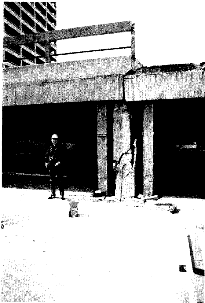
Figure 3.65. The exterior columns of the Trans World Bank parking garage, which had not been strengthened, were badly damaged.
