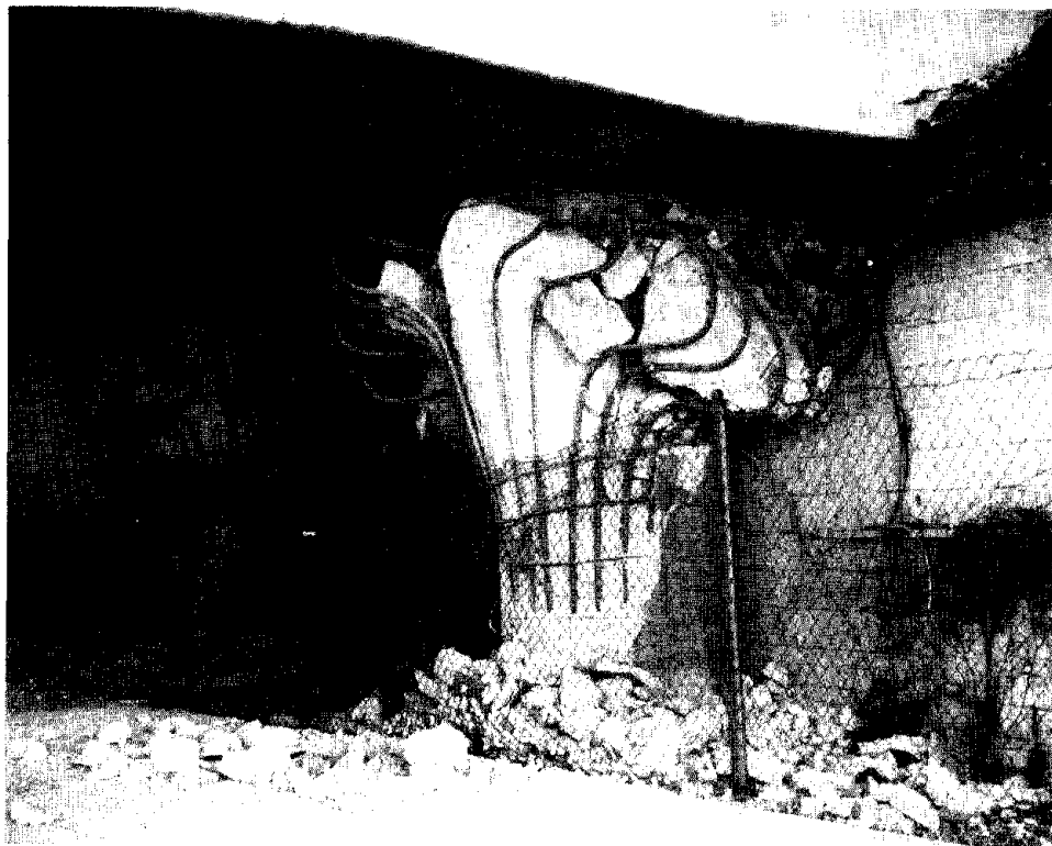
Figure 4.41. Piers of Bent 3 supporting eastbound lane of I10 at La Cienega Blvd.
