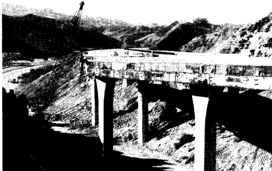
Figure 4.3. Ground level view of the southbound bridge at Gavin Canyon, looking to the northwest, showing the hinge bearing seat near Bent 3.
