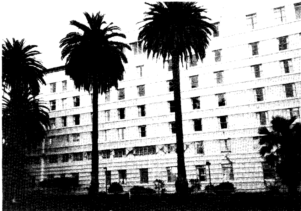
Figure 3.23. The seven-story northwest wing of St. John's hospital in Santa Monica experienced severe X-cracking in the piers between the second story windows.
