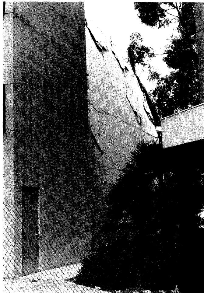
Figure 3.63. At the east and west faces of the Kaiser Permanente Hospital parking garage, shear walls made up the lateral force resisting system. Both walls had horizontal cracks caused by the out-of-plane bending when the walls were pulled inward. Neither wall had major diagonal cracking, suggesting that the lateral load was never fully delivered to the walls. The stair towers remained erect. The east wall and stair tower are shown here.
