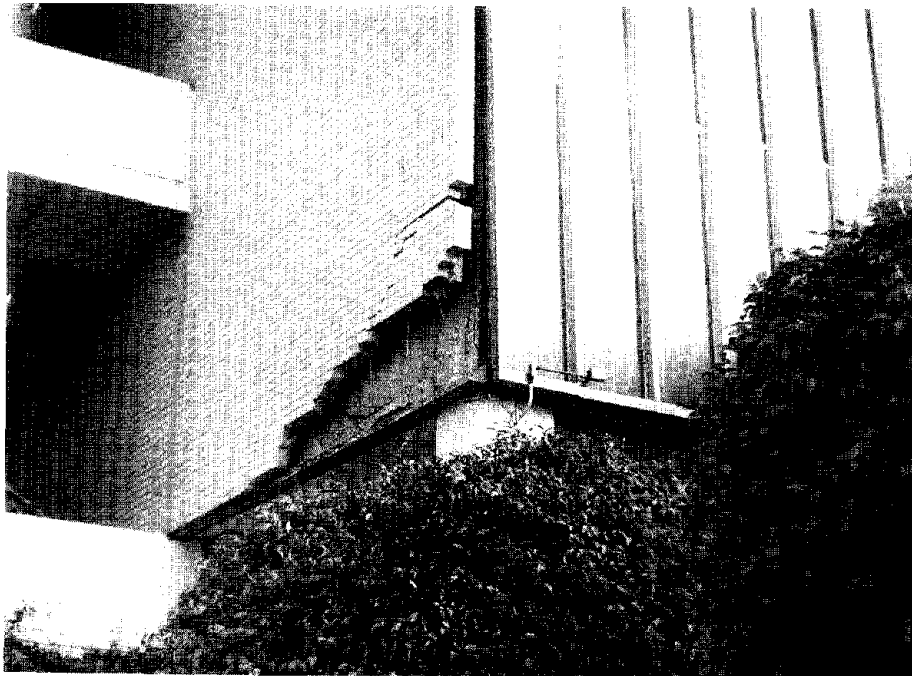
Figure 3.50. The similar west wall of was damaged, but did not peel away from the structure. This close up of the interface between the first and second stories shows that the masonry facade is supported on a steel angle. At the west end of the building, the facade was crushed at the toe where it is supported by the angle.
