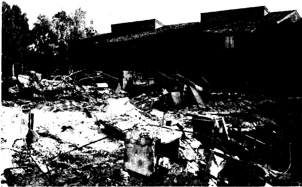
Figure 6.6. Multi-family residential building destroyed by fire.
