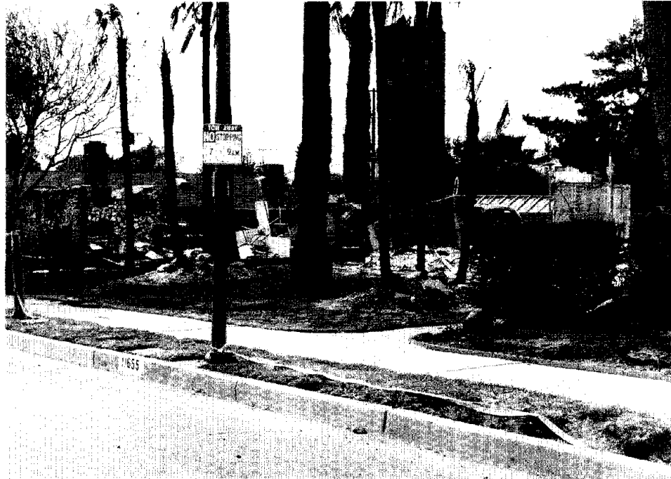
Figure 5.13. Houses destroyed by a fire resulting from the rupture of the 0.6-m gas main along Balboa Boulevard.
