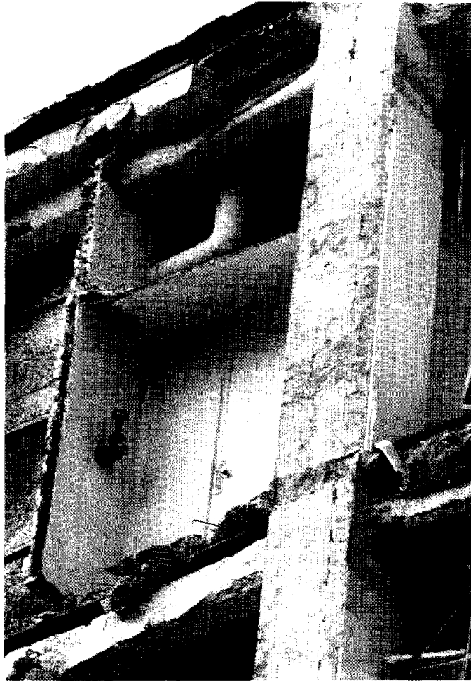
Figure 3.51. The exposed structure of the Sherman Way office building shows remains (at the floor level and the column) of the minimal ties that anchored the masonry facade.
