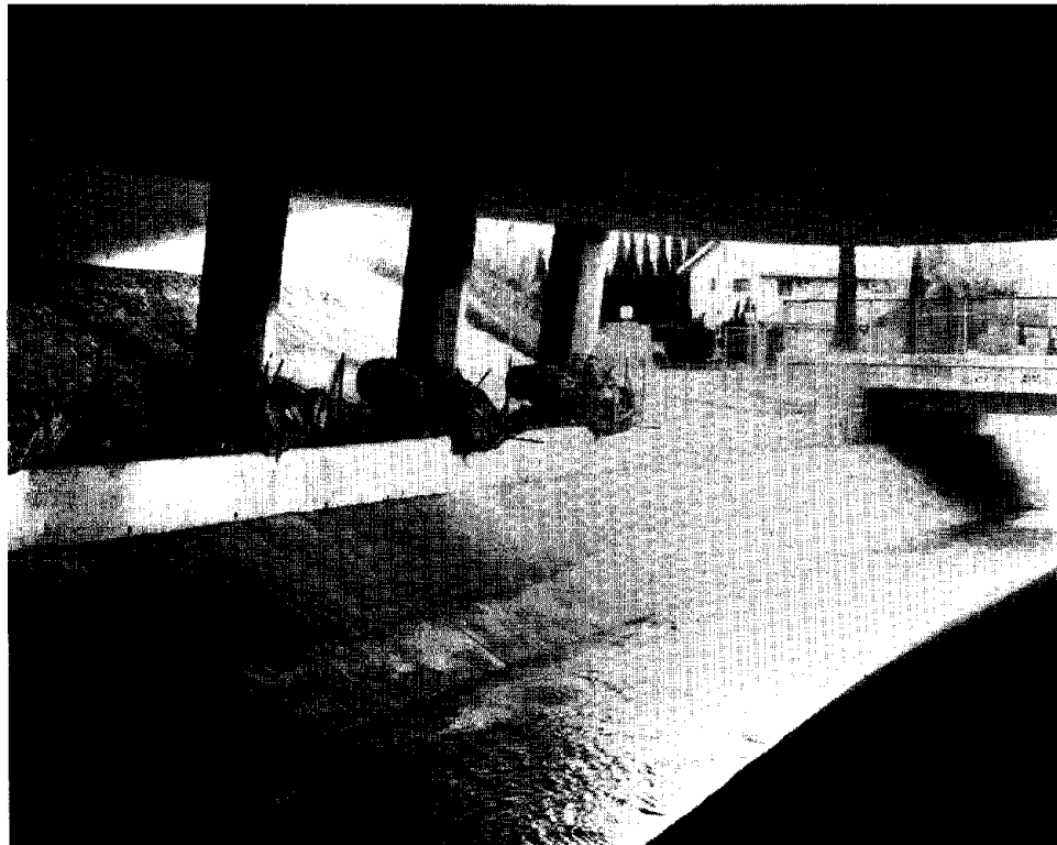
Figure 4.28. Damage to piers of Bent 3S of State Route 118 at Bull Creek Canyon Channel, looking to the southeast.
