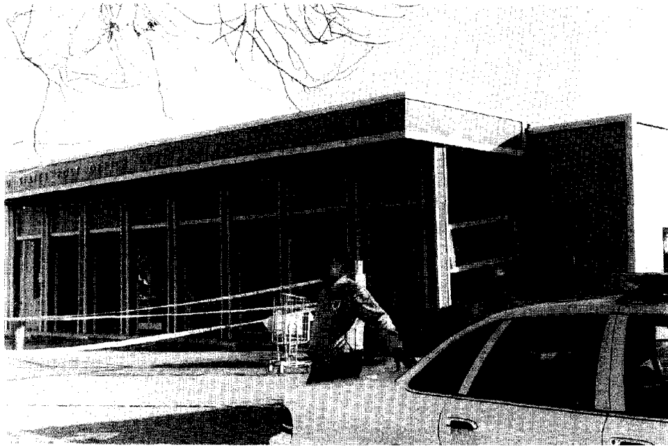
Figure 3.35. The Chatsworth Post Office was closed due to damage. Mail was being collected in the parking lot.
