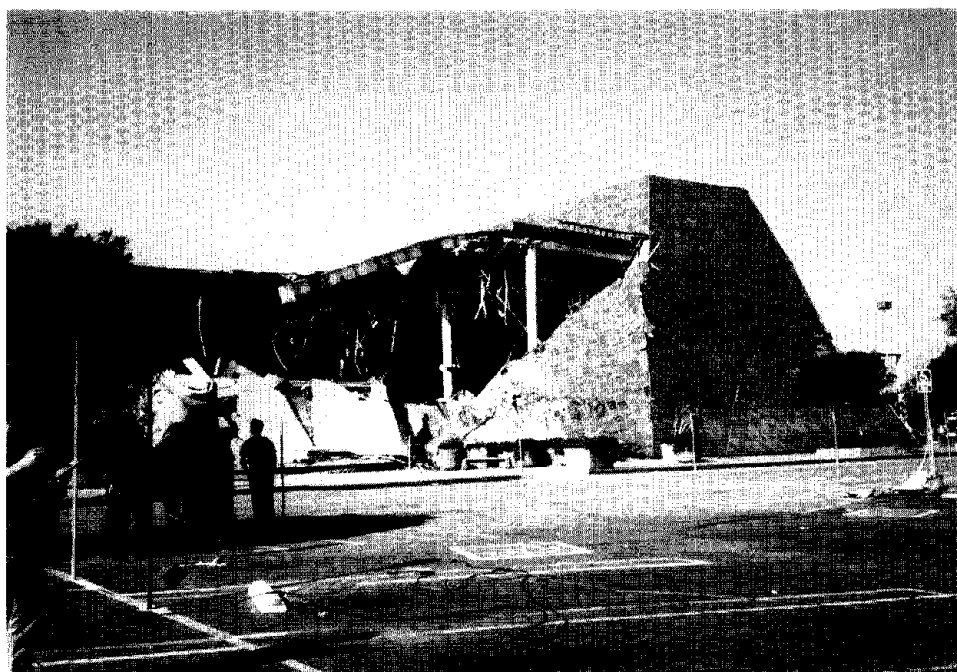
Figure 3.30. The Bullock's department store had an extremely irregular vertical geometry. At the northeast end it was shaped like a truncated pyramid.
