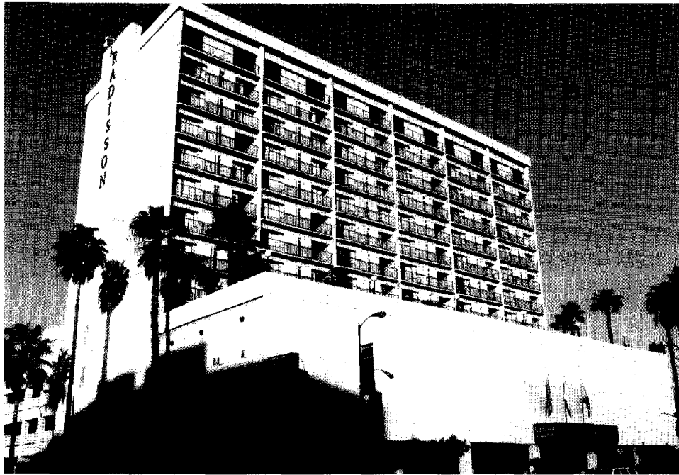
Figure 3.55. The concrete Radisson Valley Center Hotel in Sherman Oaks had serious damage to the columns at the first and fifth stories.
