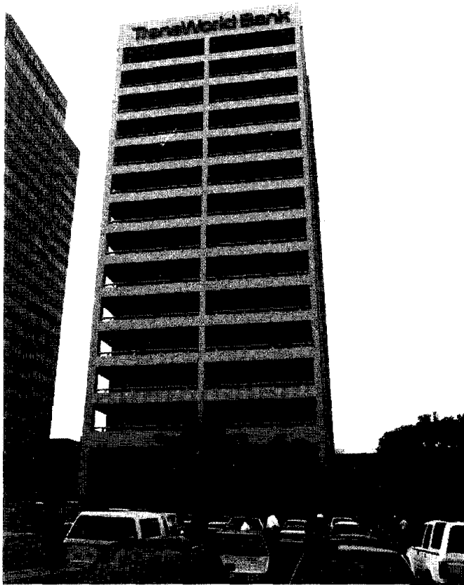
Figure 3.53. The Trans World Bank building, in Sherman Oaks, was damaged in both the 1971 San Fernando and 1994 Northridge earthquakes.
