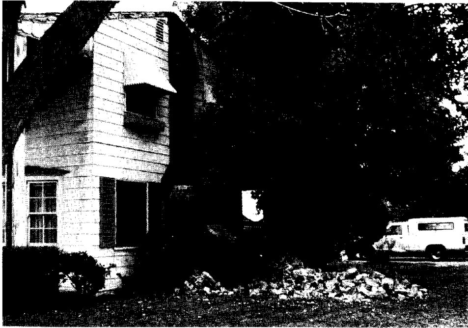
Figure 3.17. Failure of masonry chimneys was common.
