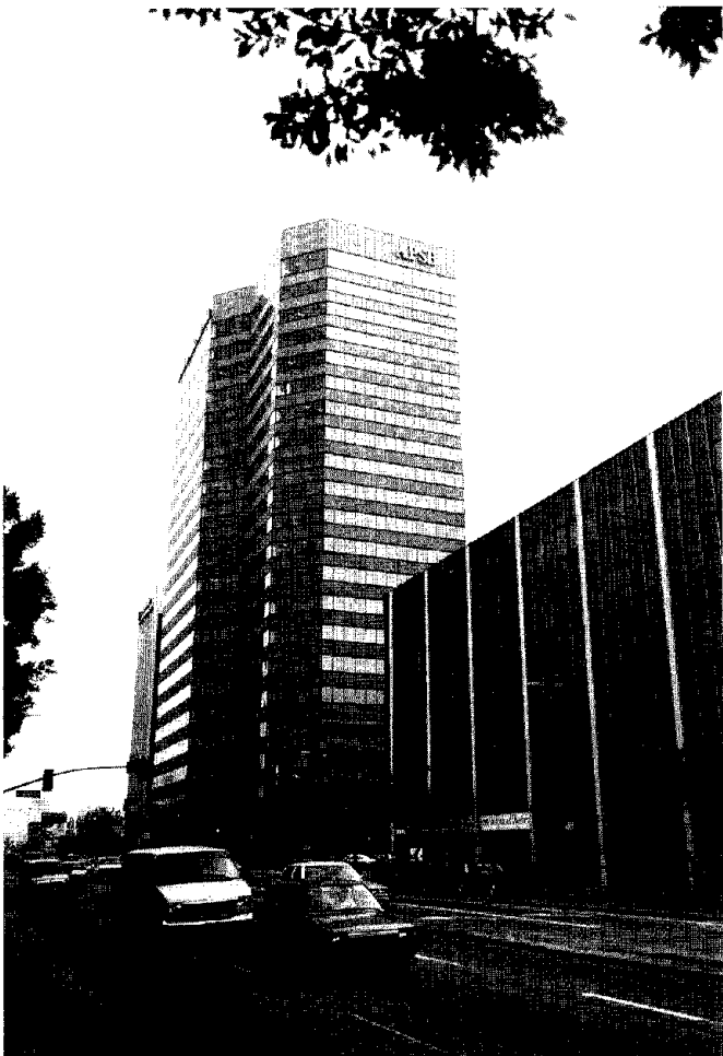
Figure 3.57. There was no evidence of damage to the 22-story American Pacific State Bank in Sherman Oaks. The adjacent eight-story parking garage had damaged columns.
