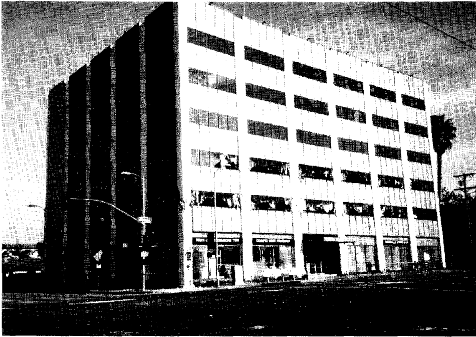
Figure 3.45. The six-story L-shaped concrete-frame Barrington Building on Olympic Boulevard in West Los Angeles lost its vertical-load carrying capacity at the second story.
