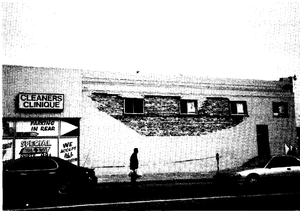
Figure 3.39. Only the exterior wythe of brick peeled off of this rehabilitated unreinforced masonry building in Santa Monica.
