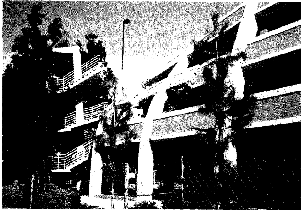
Figure 3.60. The three-year old four-level parking garage at the Northridge campus of California State University partially collapsed in the earthquake. The collapse apparently started at the interior, causing the exterior frame to be pulled in to the middle of the structure. Precast concrete "trees" were connected to form a moment-resisting frame at the exterior of the structure.
