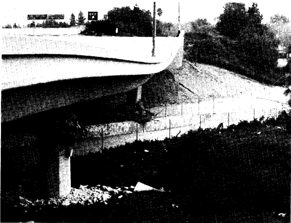
Figure 4.26. Ground-level view of State Route 118 at Bull Creek Canyon Channel, looking along the south edge, towards the east.
