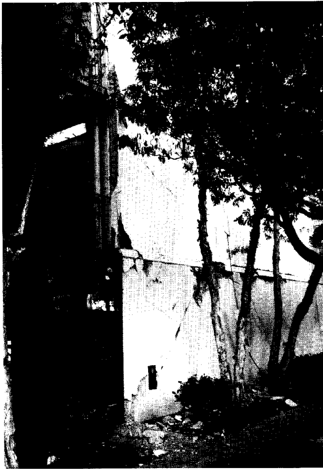
Figure 3.26. The Bay Vista Health Care Center was closed due to damage. Differential movement between the building and its base was indicated by the crack at the foundation line. The corner of the concrete foundation wall spalled, apparently due to crushing. A facade panel over the garage opening was dislodged.
