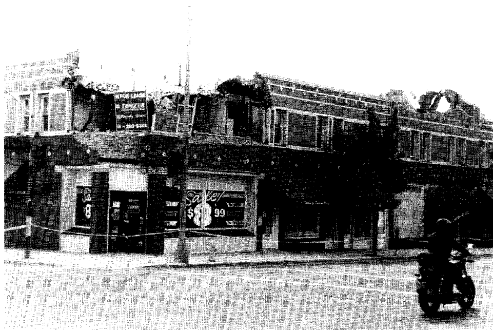
Figure 3.36. Damage to unreinforced masonry buildings, even those that had been rehabilitated, was common. Upper stories and corners were particularly vulnerable to damage. The rows of light-colored diamonds on the face of this building are the end plates of through-bolts used to connect the wall to the floor joists, a typical rehabilitation technique. The remains of parapet braces can be seen on the roof.
