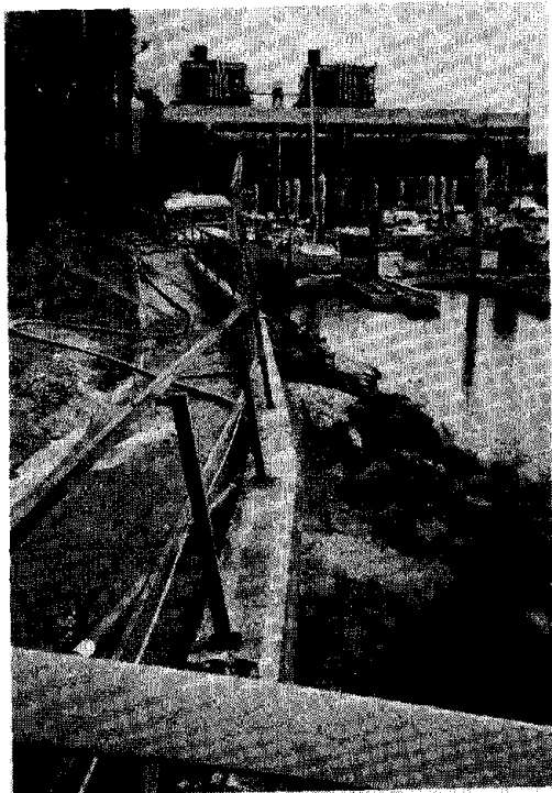
Photo 6.2 Displaced Bulkhead
