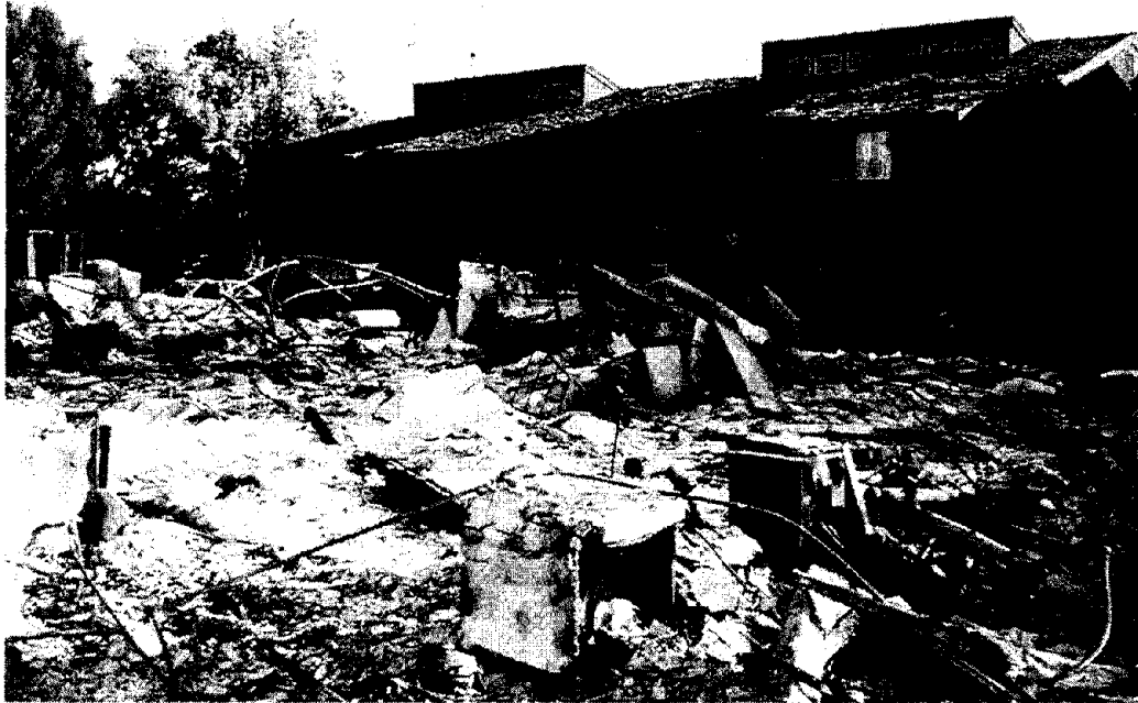
Figure 61 Multi-family residential building destroyed by fire.
