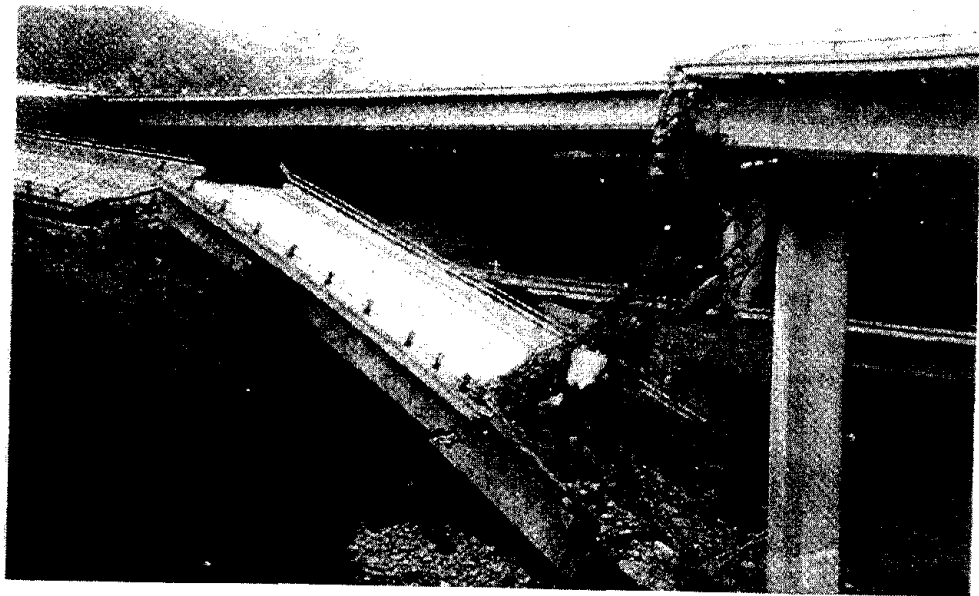
Figure 30 Collapsed portion of the SR14/15 North Connector Overcrossing, looking east.. Pier 2 was at the left, near the broken hinge on the ground (Courtesy of EERC)
