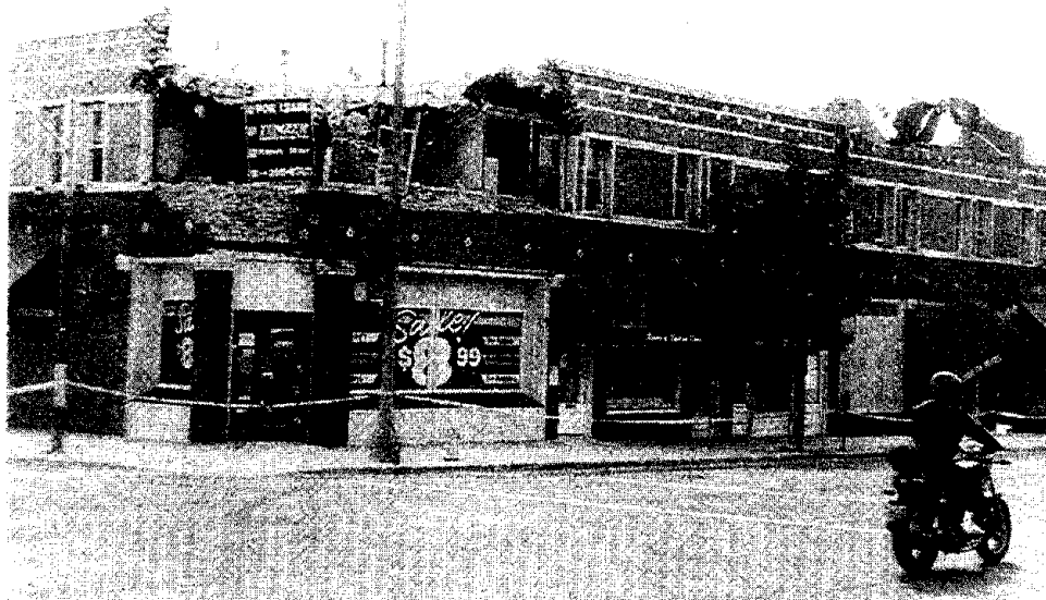
Figure 12 Damage to unreinforced masonry buildings, even those that had been rehabilitated, was common. Upper stories and corners were particularly vulnerable to damage. The rows of light-colored diamonds on the face of this building are the end plates of through-bolts used to connect the wall to the floor joists, a typical rehabilitation technique. The remains of parapet braces can be seen on the roof.
