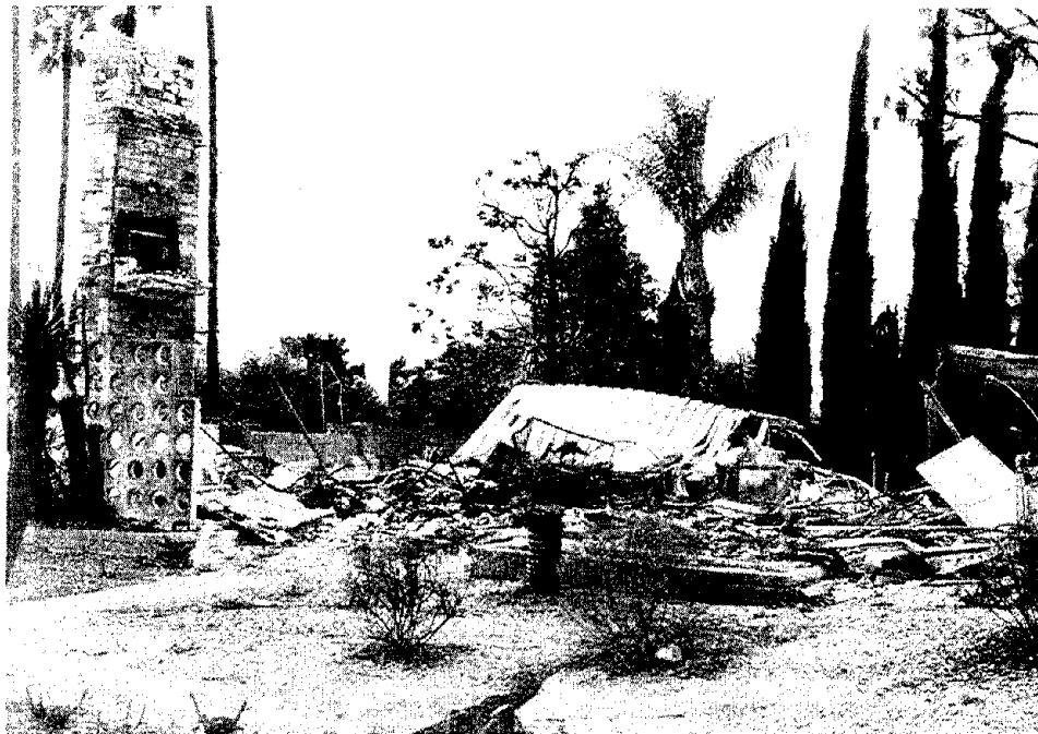
Figure 49 Houses destroyed by a fire resulting from the rupture of the 0.6-m gas main along Balboa Boulevard.
