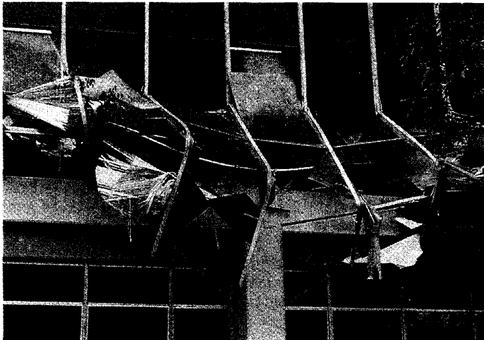
Figure 14 The second story of the concrete frame Kaiser Permanente office building on Balboa Avenue in Northridge completely collapsed. The first story was relatively undamaged, suggesting it was far stiffer than the story above.
