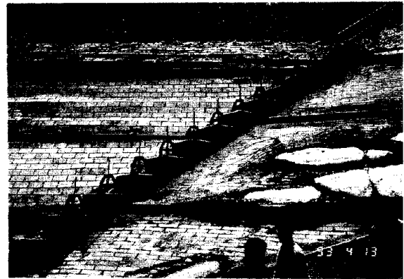
Photo.2 Undulating Deformation of Facing Concrete Blocks on the Upstream Ground Slope of the Mombetsu Dam Left Bank
