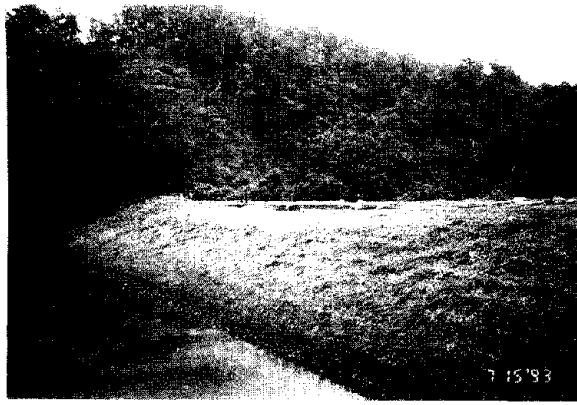
Photo.6 Damage to Niwa-Ikumine Dam (Photographed from the spillway on the left bank on July 15, By the Courtesy of the Kita-Hiyama Land Improvement District)
