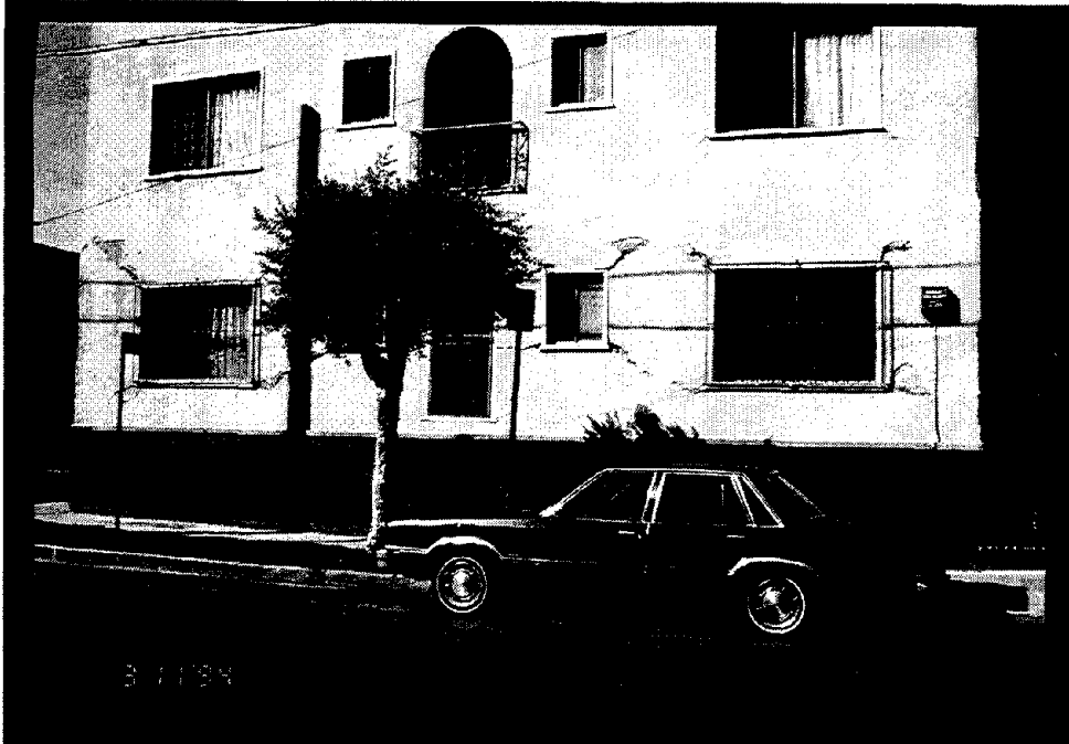
Figure 1 Residential construction is characterized by multiple door and window openings. The corners of these rectilinear openings create stress concentrations, making these locations particularly vulnerable to cracking.
