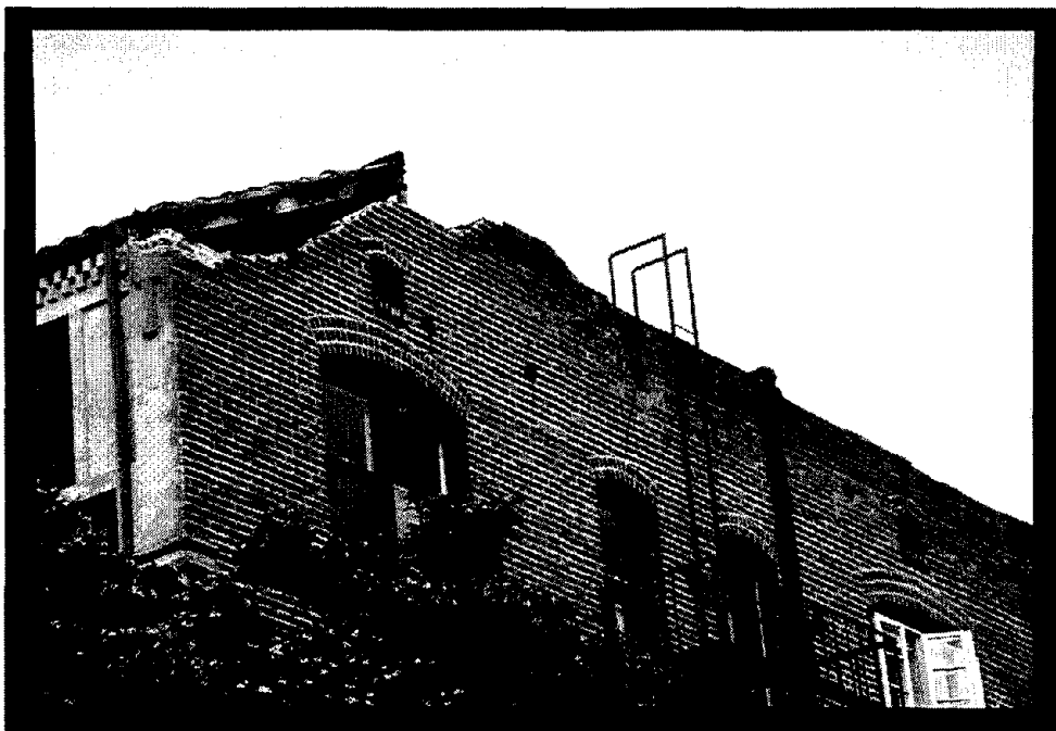
Figure 5 Loss of portions of the parapet and wall at Uptown Manor, an unreinforced masonry building, caused several living units to be declared unsafe by city inspectors.
