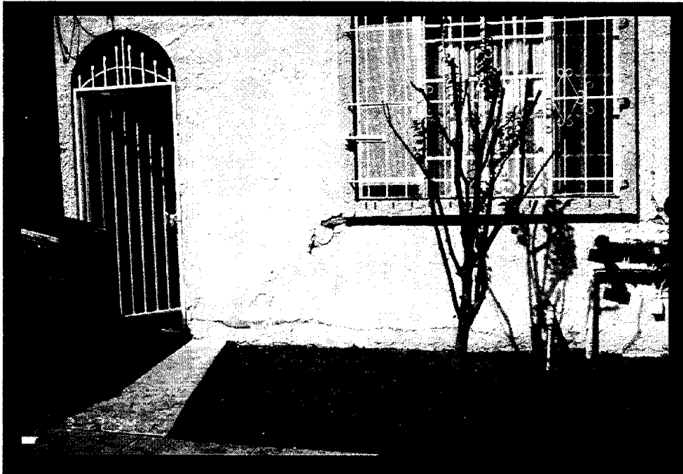
Figure 6 Sunset Apartments E, a three-story wood-frame apartment building, was declared by city inspectors to be potentially unsafe pending more detailed evaluation (yellow tagged). Note the horizontal crack in the stucco at the foundation line, the vertical crack to the right of the window, and the diagonal crack and buckled area of stucco at the lower corner of the window.
