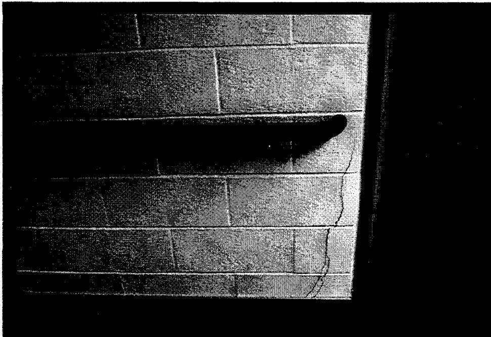
Figure 18 At Pledgerville Senior Center, a 9-year old reinforced masonry building about 13 km from the epicenter, inclined vertical cracks were observed adjacent to door openings.
