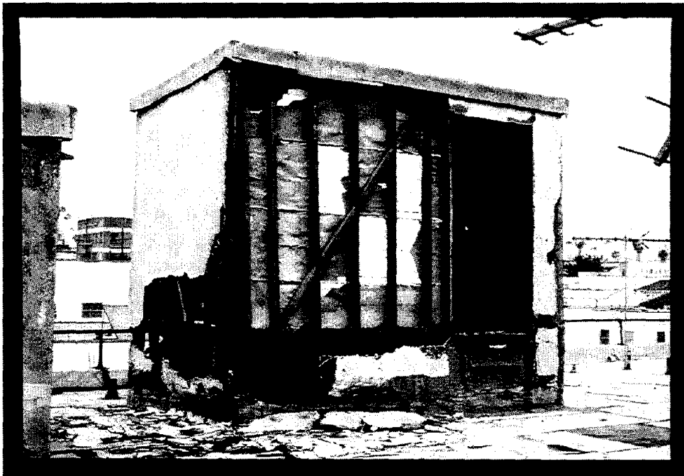
Figure 22 The wood-framed, stucco-clad elevator penthouse on the roof of the 3-story Vadehra IIIb building experienced extensive damage to the stucco, but the operation of the elevator was not affected.
