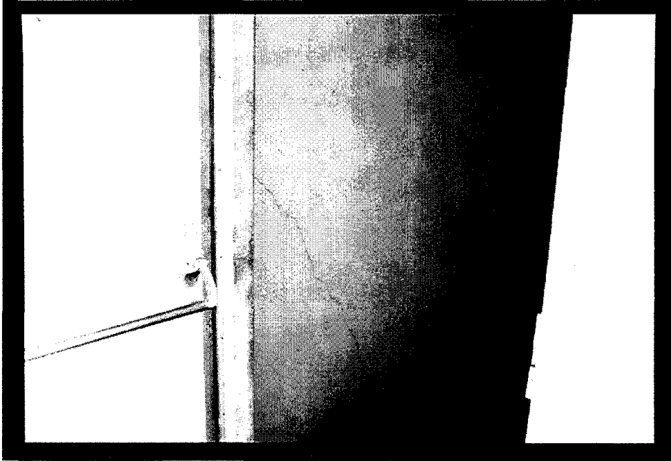
Figure 12 Structural damage in concrete buildings included diagonal cracks in shear walls, such as these in Beverly Towers.
