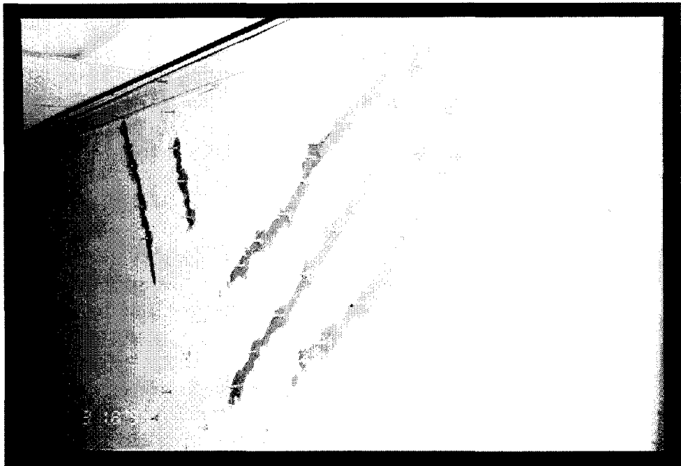
Figure 13 Some of the diagonal cracks in concrete shear walls were already under repair at the time of this study. At Santa Monica Christian apartments, cracks were being repaired using an epoxy injection technique.
