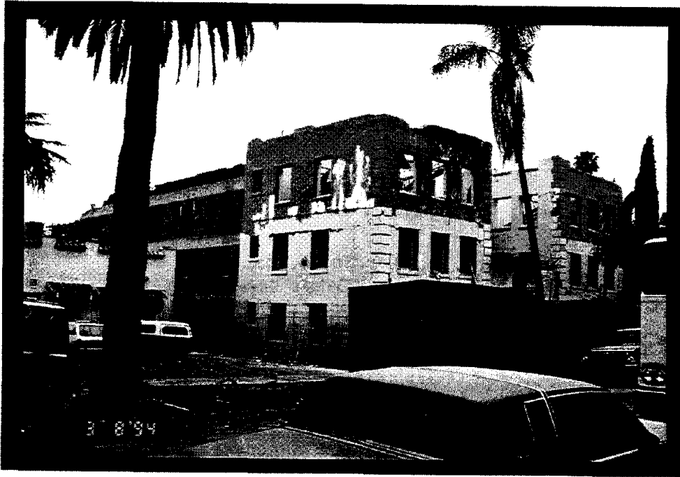
Figure 4 Vadehra IV, an unreinforced masonry building, was condemned because of extensive earthquake damage. When this photograph was taken, the top story had already been removed by the demolition team.
