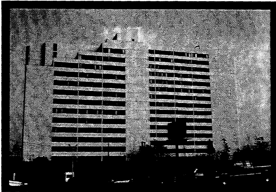
Figure 10 Cathay Manor, a 16-story building about 33 km from the epicenter, was determined to be a concrete shear wall building.
