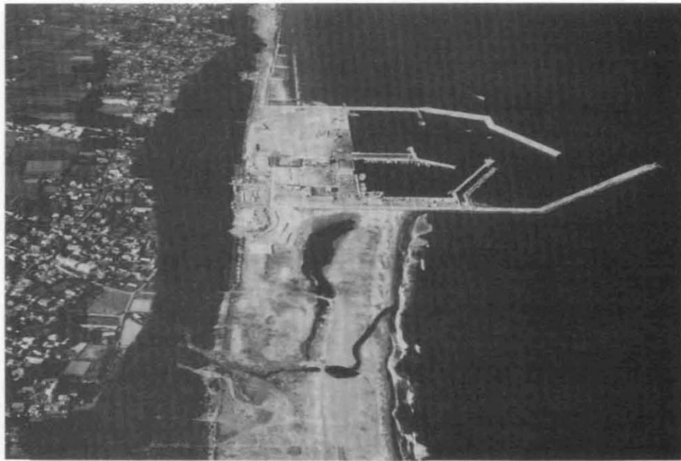
Photo 5 Severe Erosion and Sedimentation around Misawa Fishery Port
