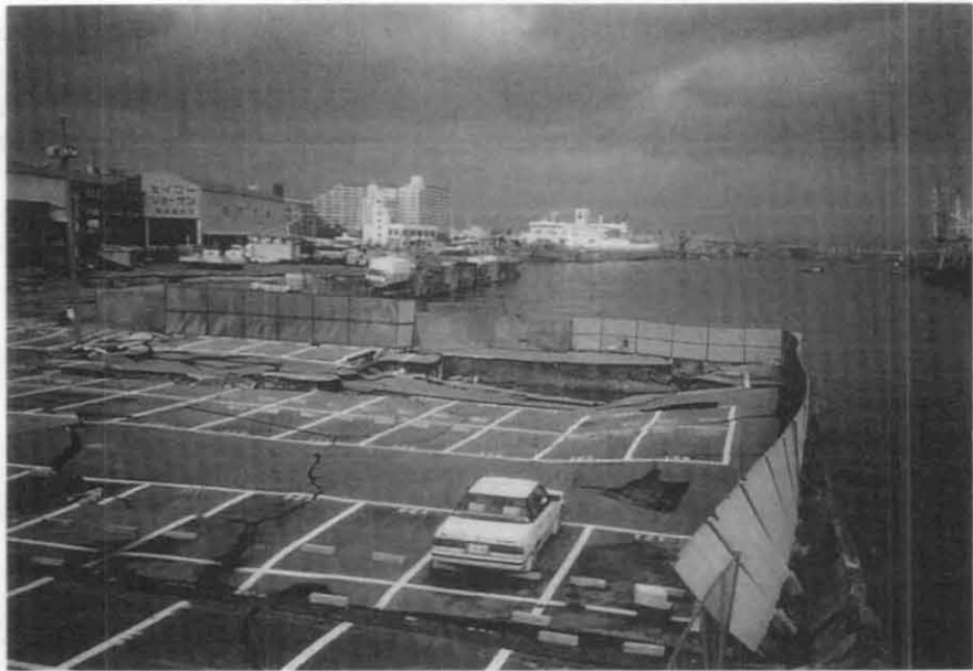
Photo 1 Damage to a Parking Lot at Uozakihama
