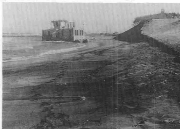
Photo 4 Collapsed Meteorological Observatory at Niigata Coast
