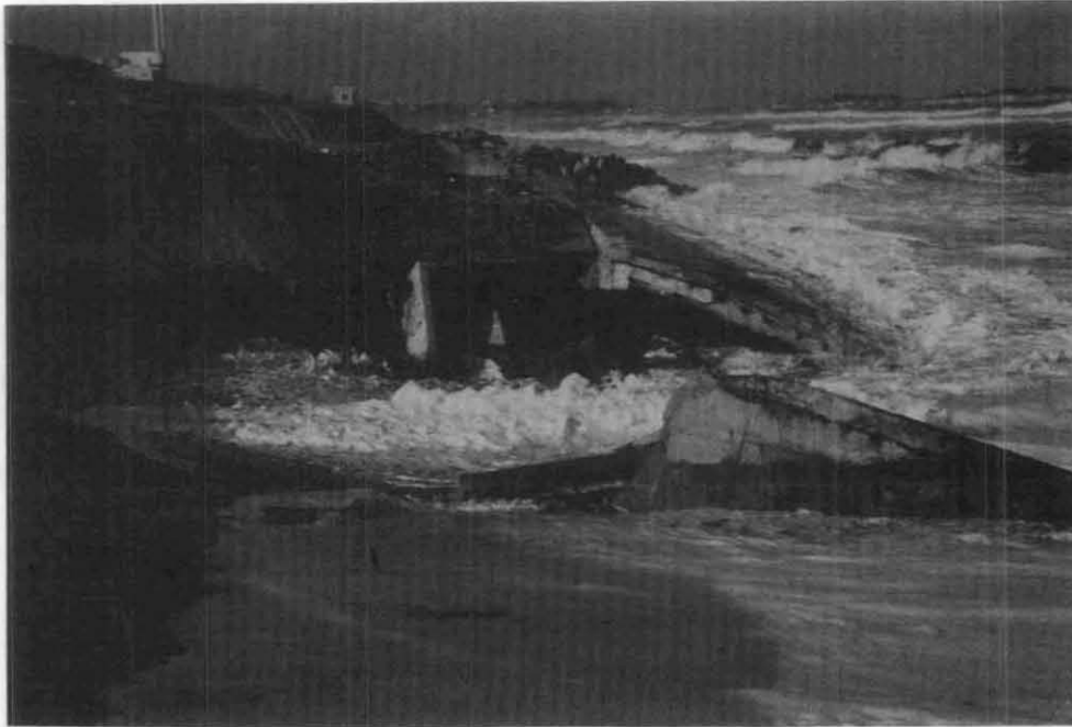
Photo 6 Seawall Damage by Erosion at Oarai Beach
