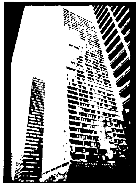
Figure 1. Window Glass Breakage in Downtown Houston, Texas Following Hurricane Alicia in August 1983
