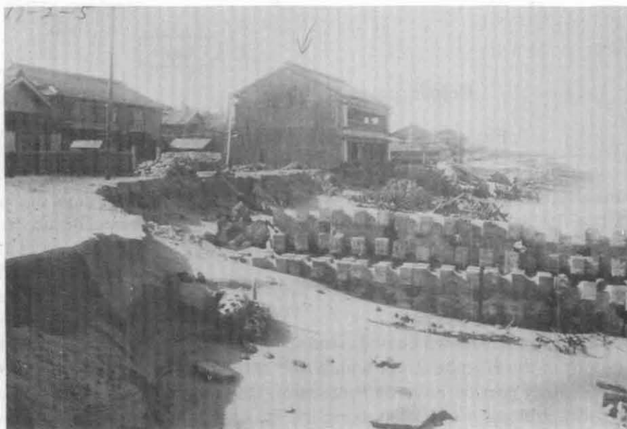
Photo 2 Hotel is about to Collapse
