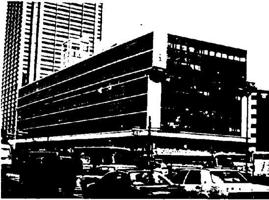
Photo.1. Complete collapse of mid-height story of a eight story building.
