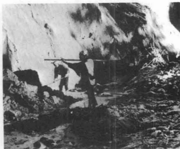
Photo 1 Digging Decomposed Granite for Separation of Iron Sand
