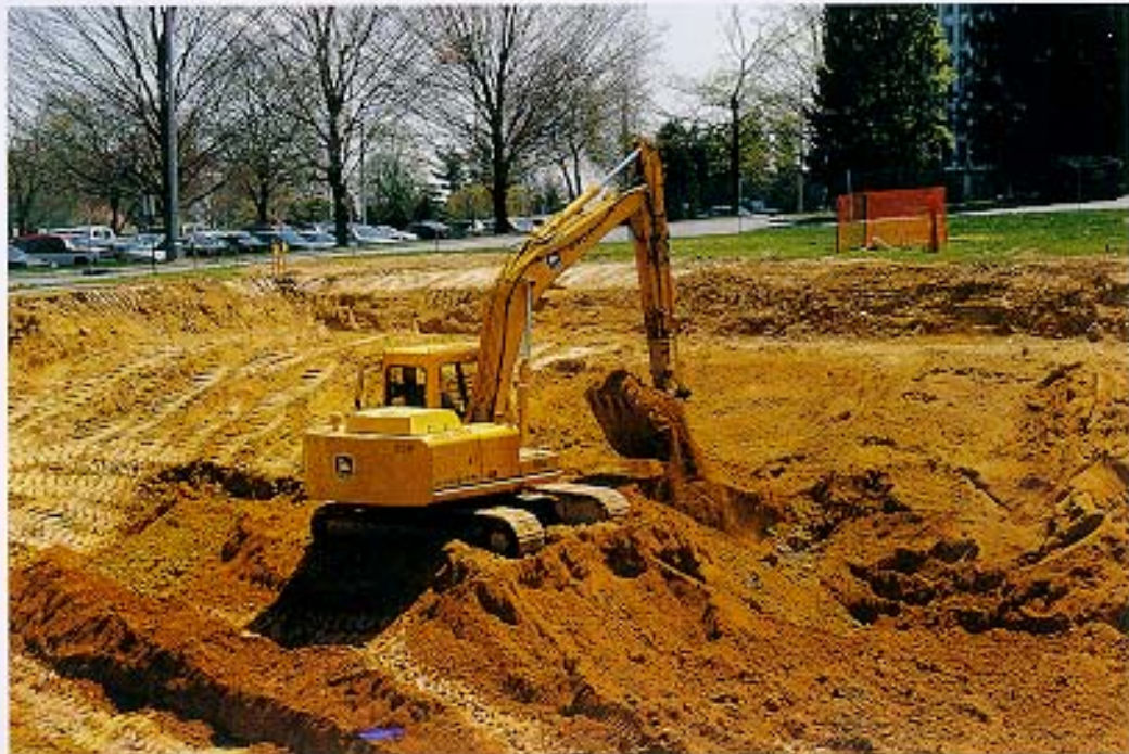
Excavation for NIST's new Advanced Chemical Sciences Laboratory
