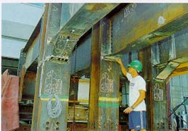
Investigation of beam column connections
