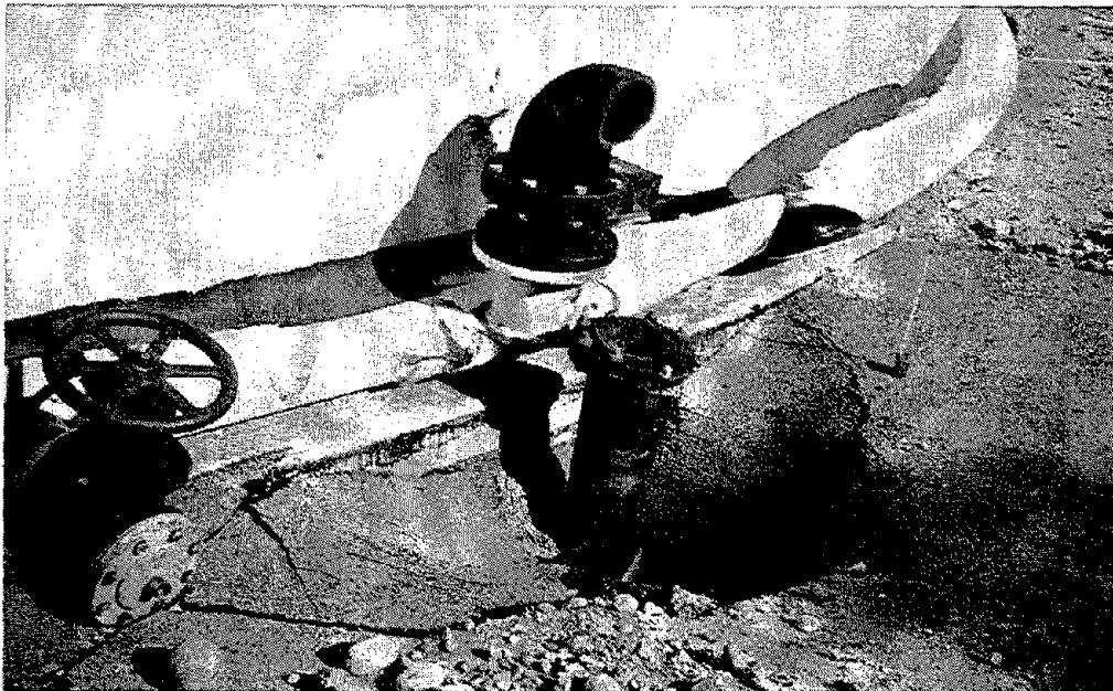
Fig. 4.21 Damaged 0.85 mg welded steel tank in Newhall area. Cast iron fittings failed and tank wall is torn across elephant foot buckle. Anchor straps are coned by the elephant foot buckle.
