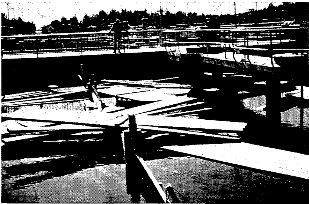
Fig. 4.32 Wood baffles damaged by sloshing at water treatment plant. (MWD)
