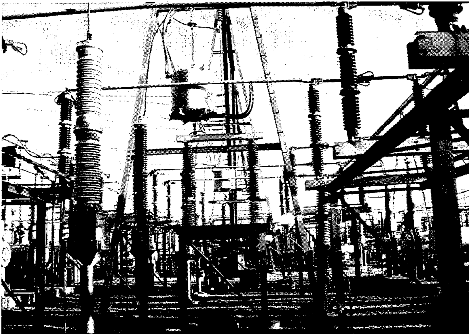
Fig.3.40 Rigid bus used to connect disconnect switches at line drop contributed to disconnect switch damage.
