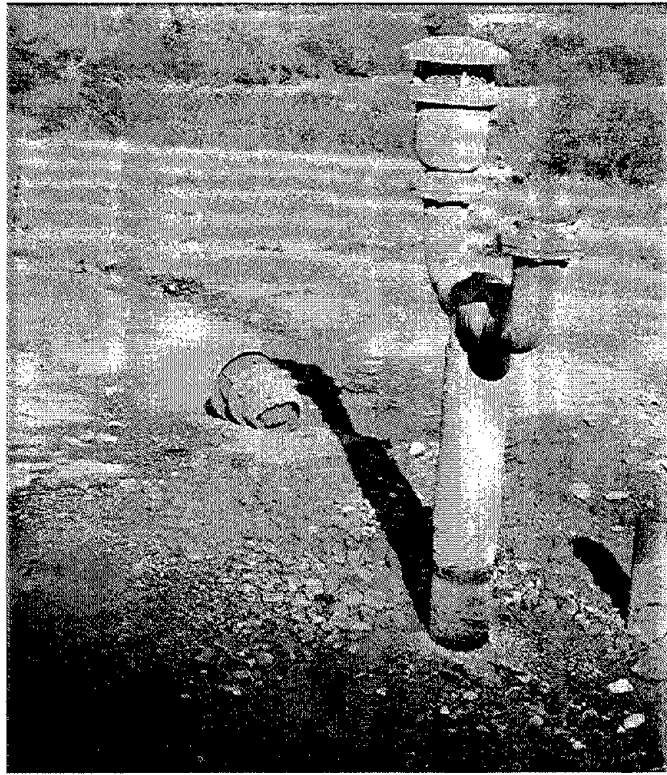
Fig. 4.17 Typical damaged to air and vacuum valves installation.
