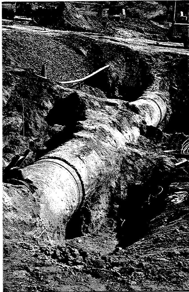
Fig. 4.2 Excavating pulled joints and repair of 54-inch MPCCP with rubber gasket joints near Rye Canyon.
