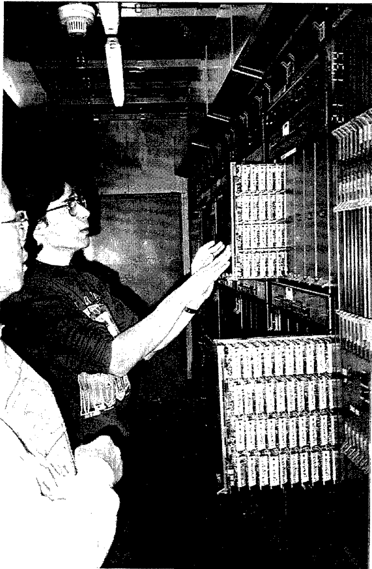
Fig. 6.4. Line disruption due to unseated or damaged circuit boards.
