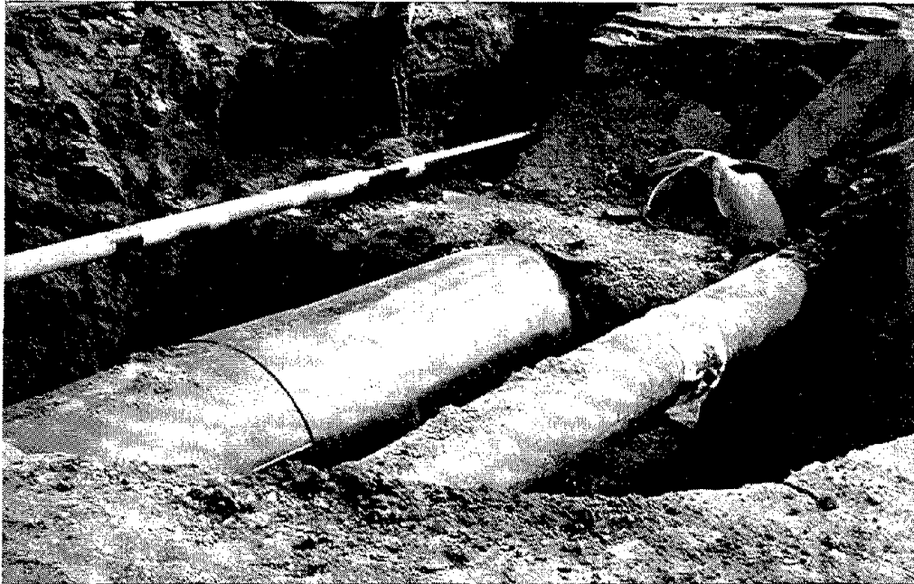
Fig. 4.37 Completed pipeline repairs at Balboa Blvd. at Halsey St.
