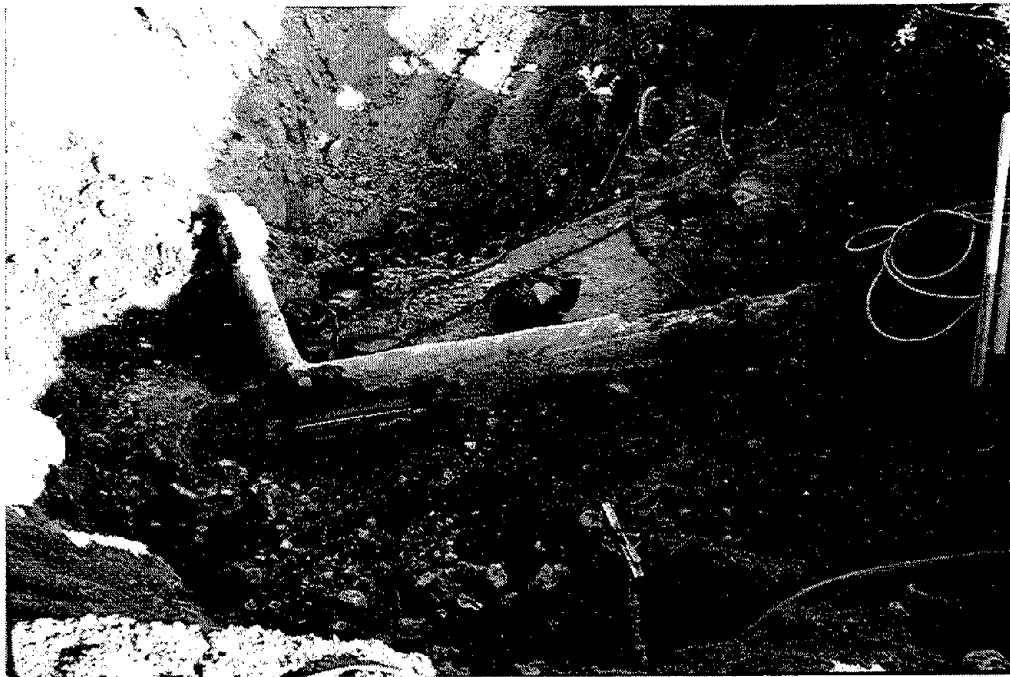
Fig. 4.13 Repaired 77-inch WSP wye branch stiffener at Terminal Hill.
