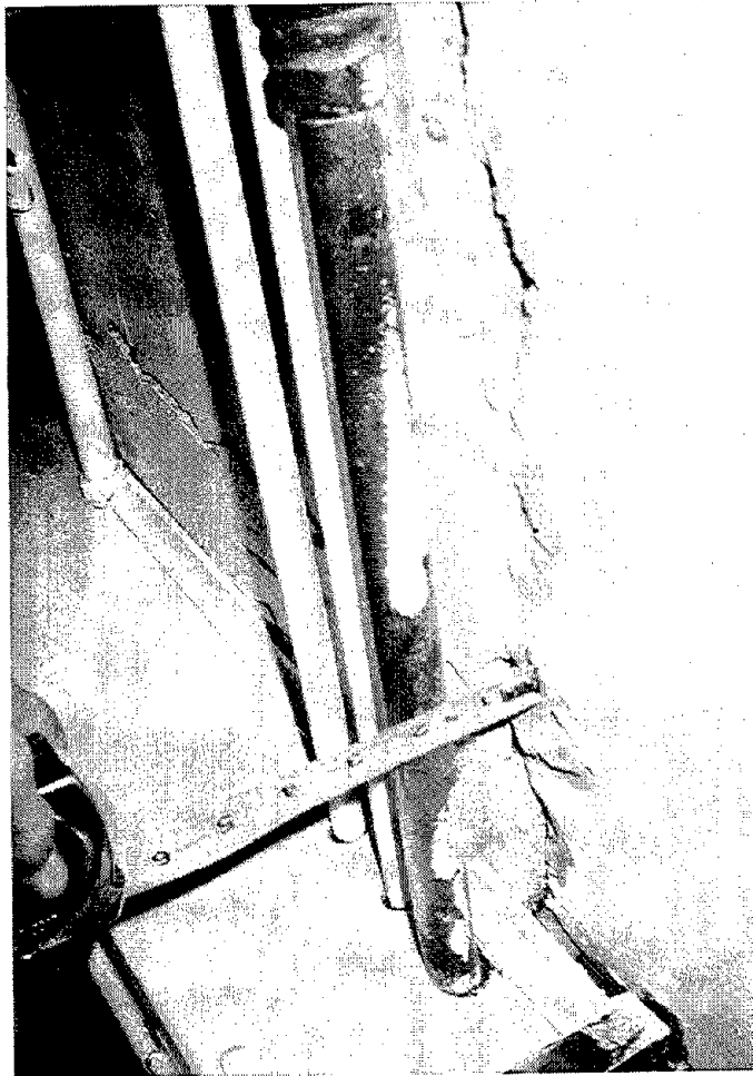
Figure 15.17. VA Hospital. Bldg. #40. Interior of infill wall at northeast corner.
