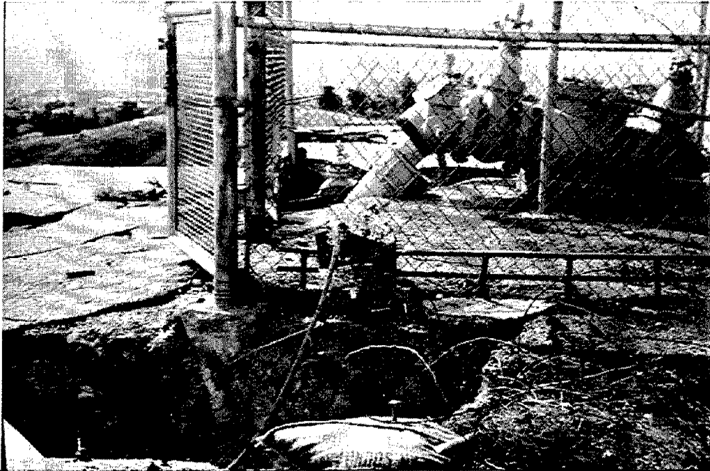
Fig. 4.25 Typical ground erosion from tank draining. (LADWP)
