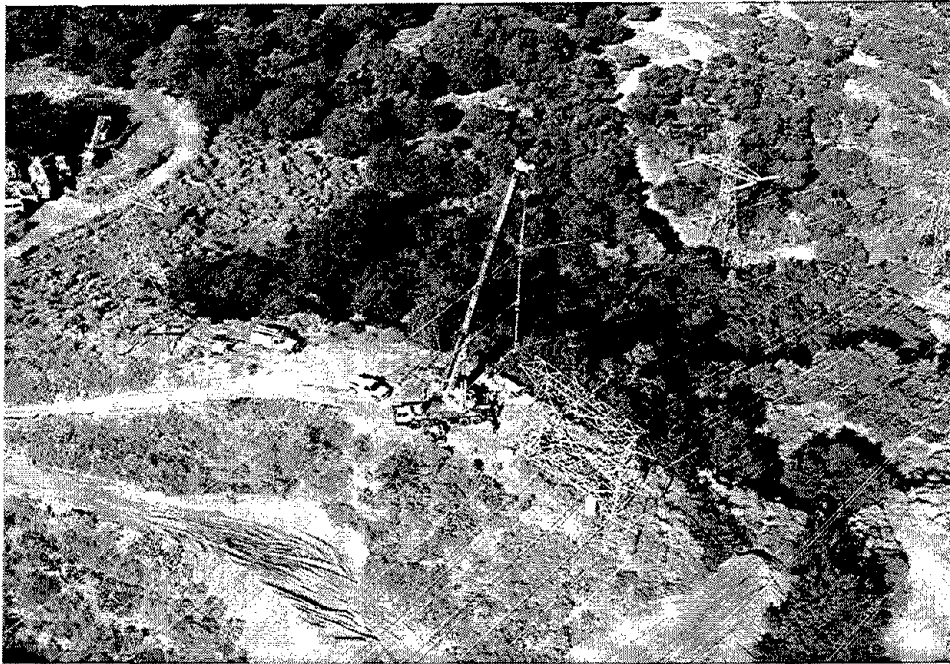
Fig. 3.43 A crane was used to temporarily replace a failed transmission tower to restore service.
