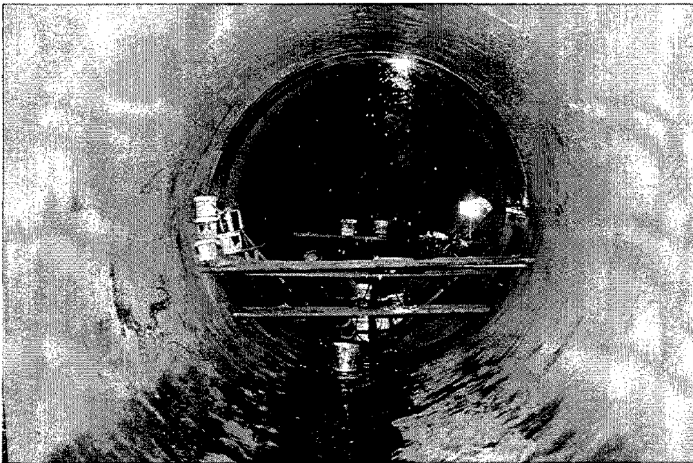
Fig. 4.10 Internal repair by steel liner of Elsmere Canyon 120-inch concrete conduit. (J. Herbaugh)
