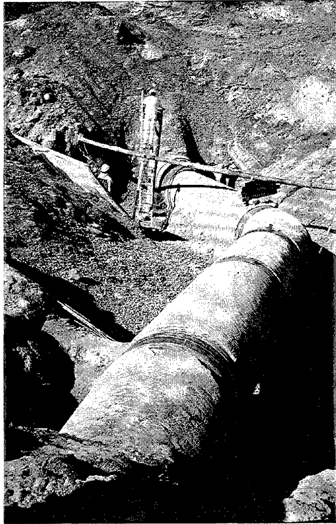
Fig. 4.3 Repaired 54-inch using contractor fabricated WSP compound bend with welded butt straps near Rye Canyon.
