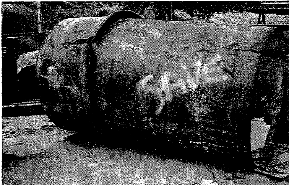
Fig. 4.36 48-inch welded steel bell and spigot joint from Balboa Blvd. at Halsey St.
