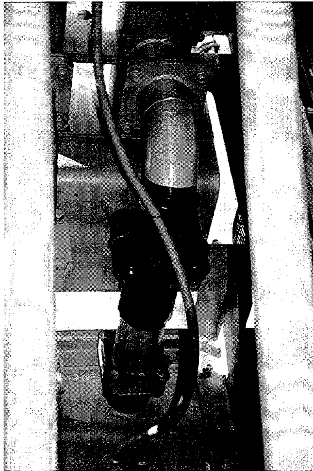
Fig.3.14 Transmission-line splice shroud used to stop leaking transformer radiator connection.
