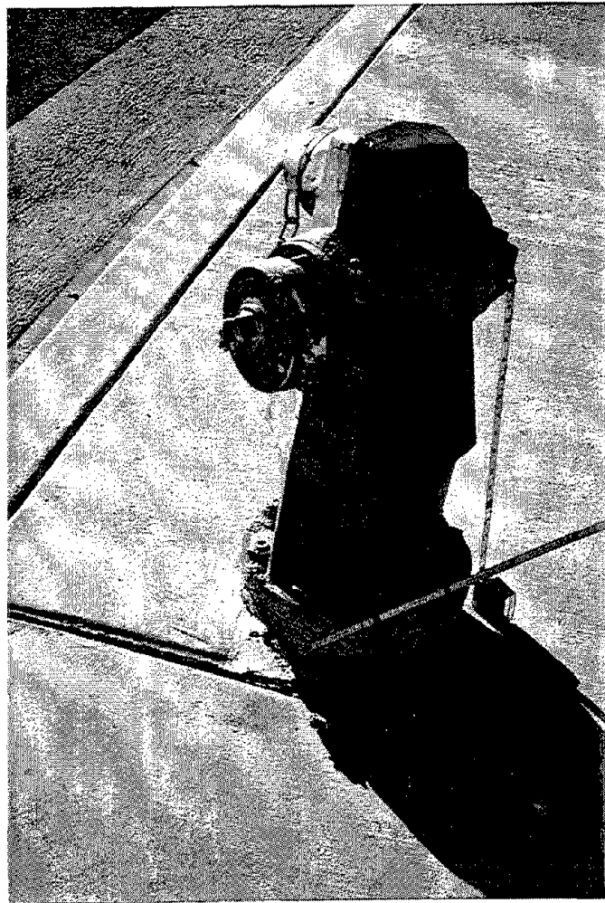
Fig. 4.16 Typical broken fire hydrant.
