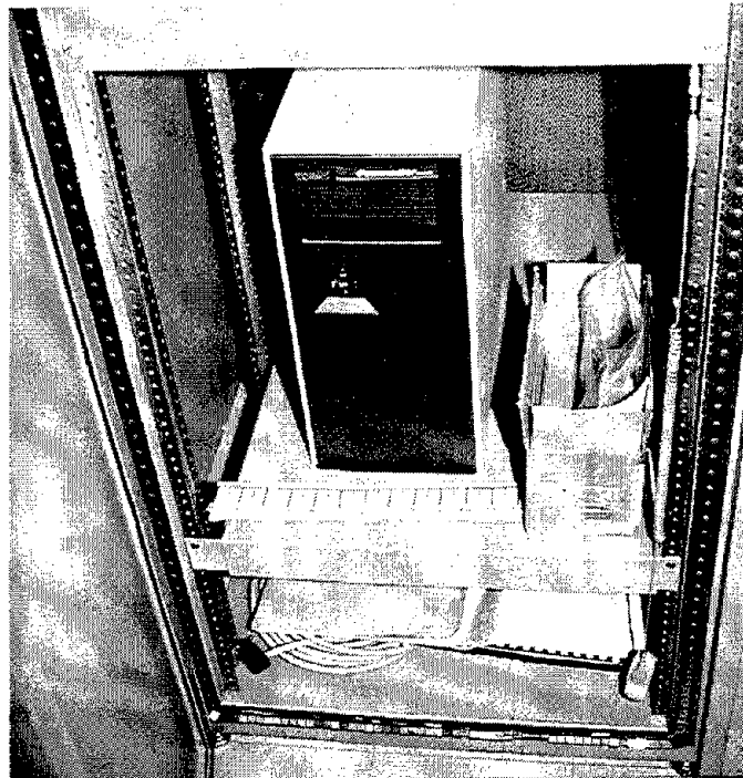
Fig. 10.6 A uninterruptible power supply in the bottom of a cabinet was unanchored. It did not move and continued to operate after the earthquake.
