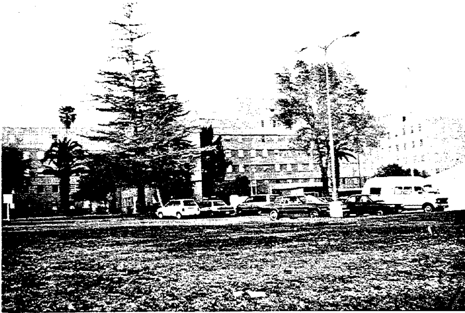
Figure 15.6. VA Hospital. View of south side of building #3.
