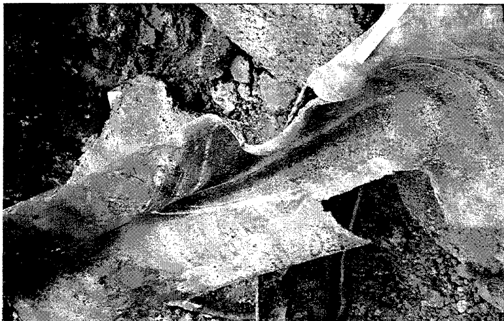
Fig. 4.34 Balboa Blvd. at Halsey St. compression zone 68-inch WSP buckled bell and spigot joint.
