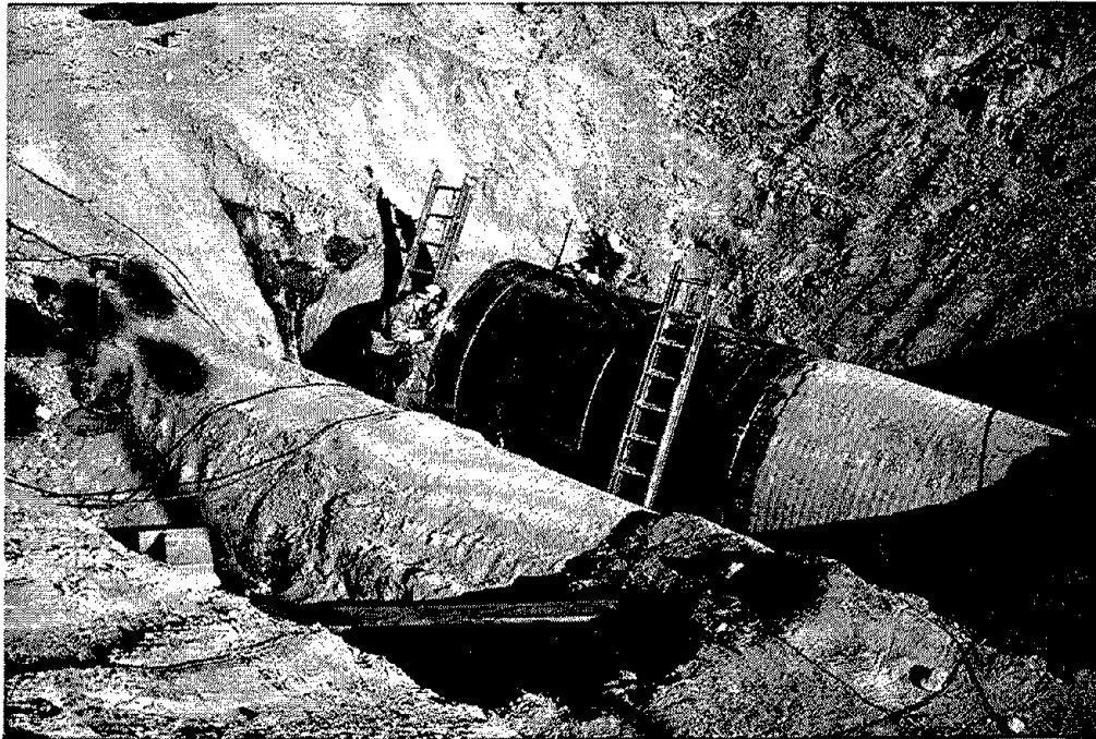
Fig. 4.5 Repaired Jensen influent 85-inch WSP, two 5 ft lengths of pipe, connected with three butt straps.
