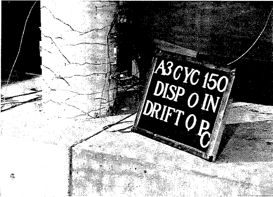
FIGURE 4-10 Specimen A3 at End of Fatigue Testing
