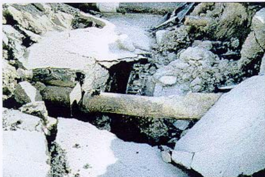
3-6: Broken water and gas mains on Balboa Boulevard in an area of extensive ground failures possibly caused by faulting. The broken gas main (foreground) ignited and caused a fire that burned down five houses and damaged several more.
