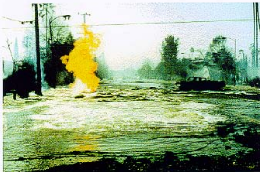
3-7: This fire on Balboa Boulevard in Granada Hills destroyed several homes and was caused by an unusual sequence of events. Adjacent water and gas mains broke because of ground failure (possible faulting). According to eyewitness, the truck stalled because of the flooding, and when the driver attempted to restart the vehicle, the leaking gas was ignited.
