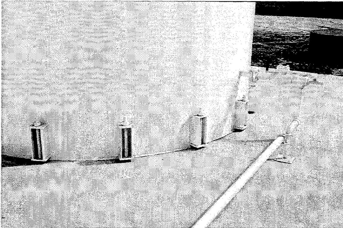
Figure 10.5 Anchor bolts and chairs on Tank AG2.
