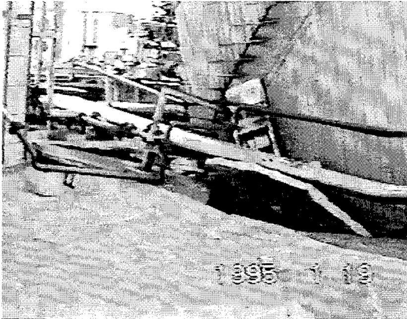
Figure 11.2 Settlement and tilting due to liquefaction (GATX video).
