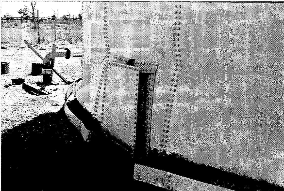
Figure 9.7 CSA-70 clean-out door, tank on rock foundation.
