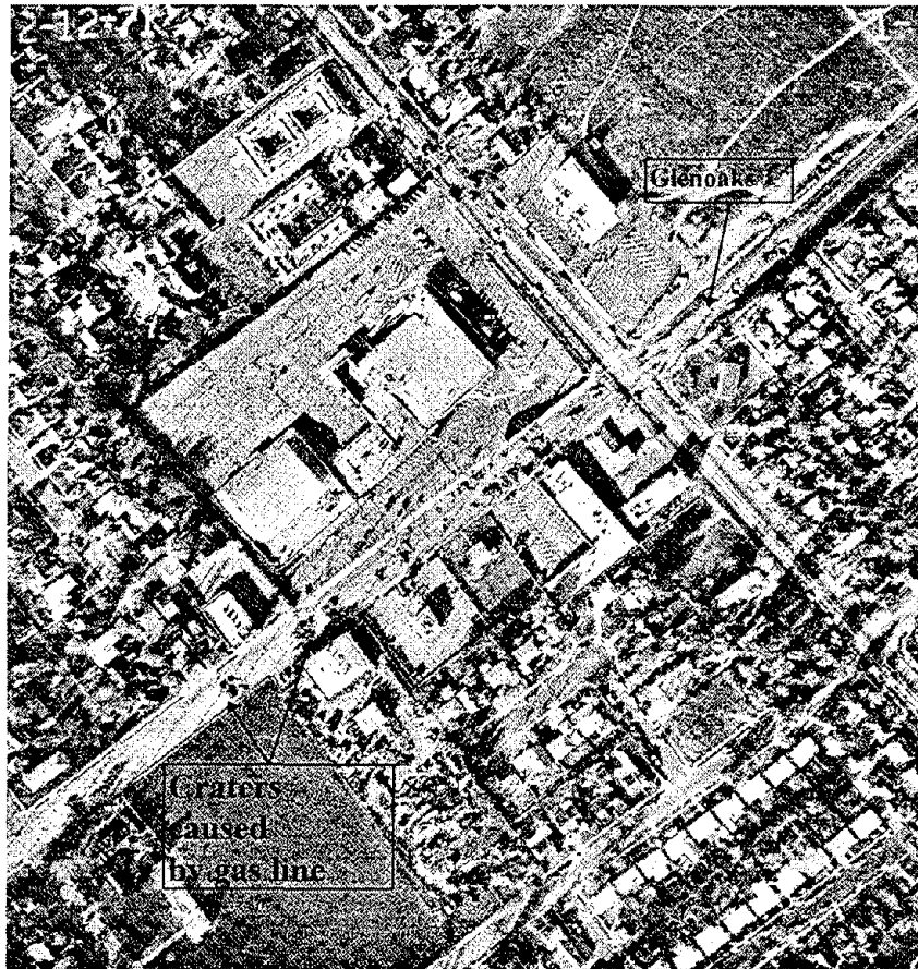
Figure 1. Cratering caused by gas leakage and explosions along Glenoaks Blvd. After the 1971 San Fernando Earthquake
